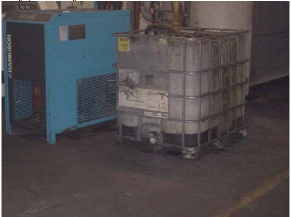
Photograph 12 – Compressor blow-down oil collection tank
