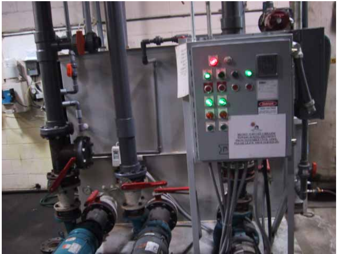
Photograph 17 – Chiller tower tank and pumps
