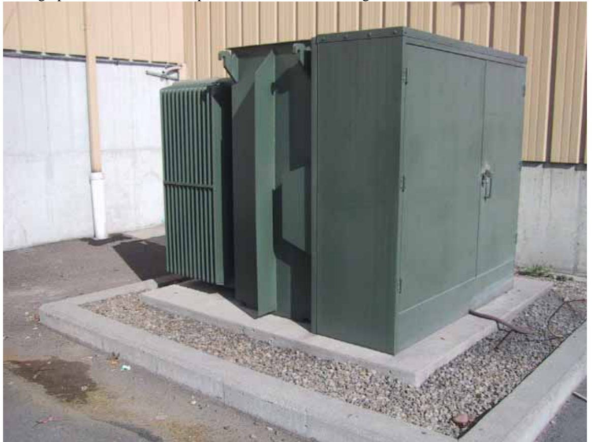
Photograph 10 – Pad-mounted transformer
