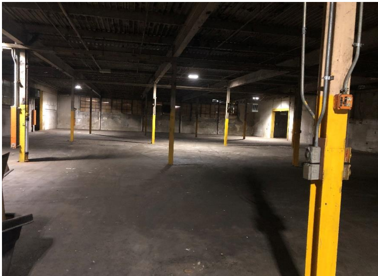
View of a typical vacant portion of the onsite building.
