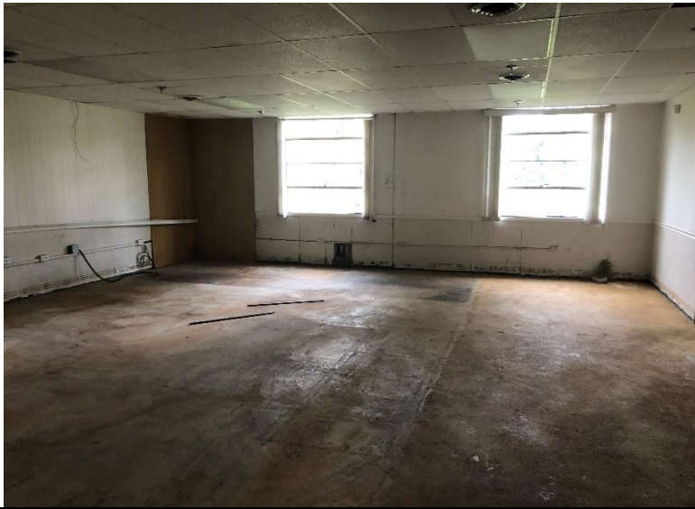
View of the office area.
