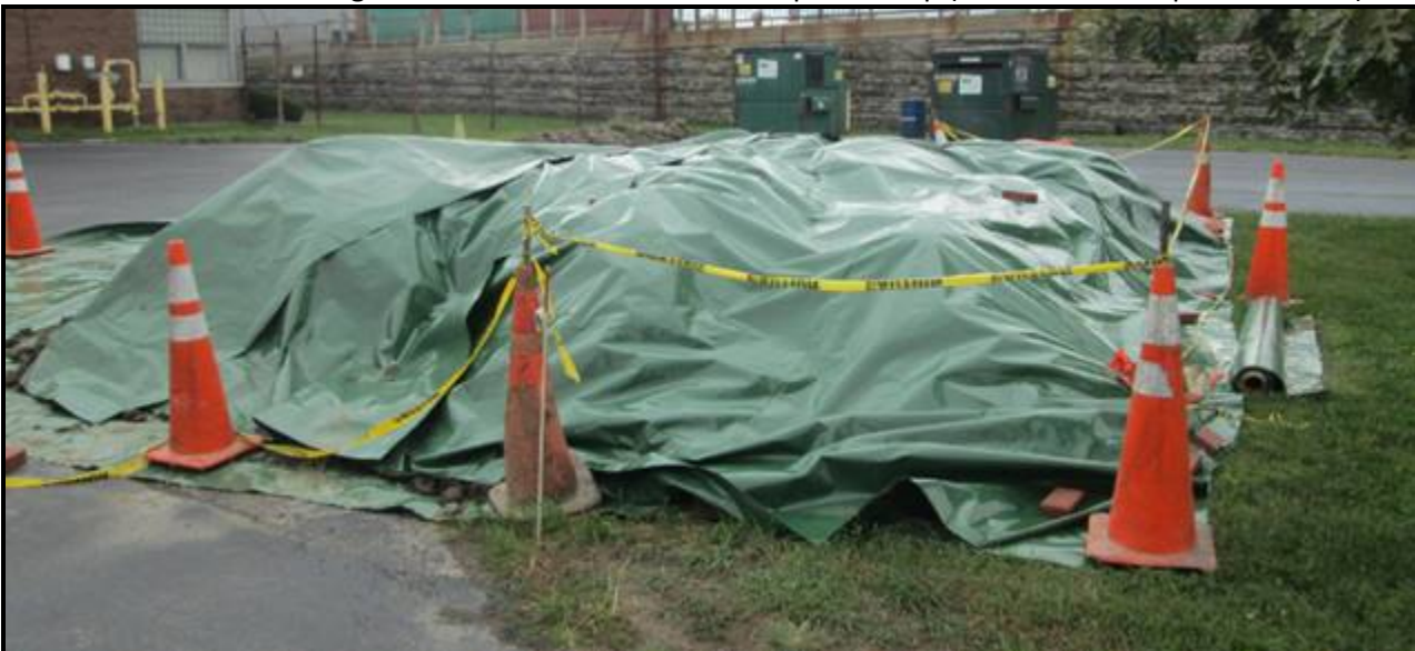
The excavated soil was staged on and covered with a 15-mil plastic tarp (as shown in the picture below).
