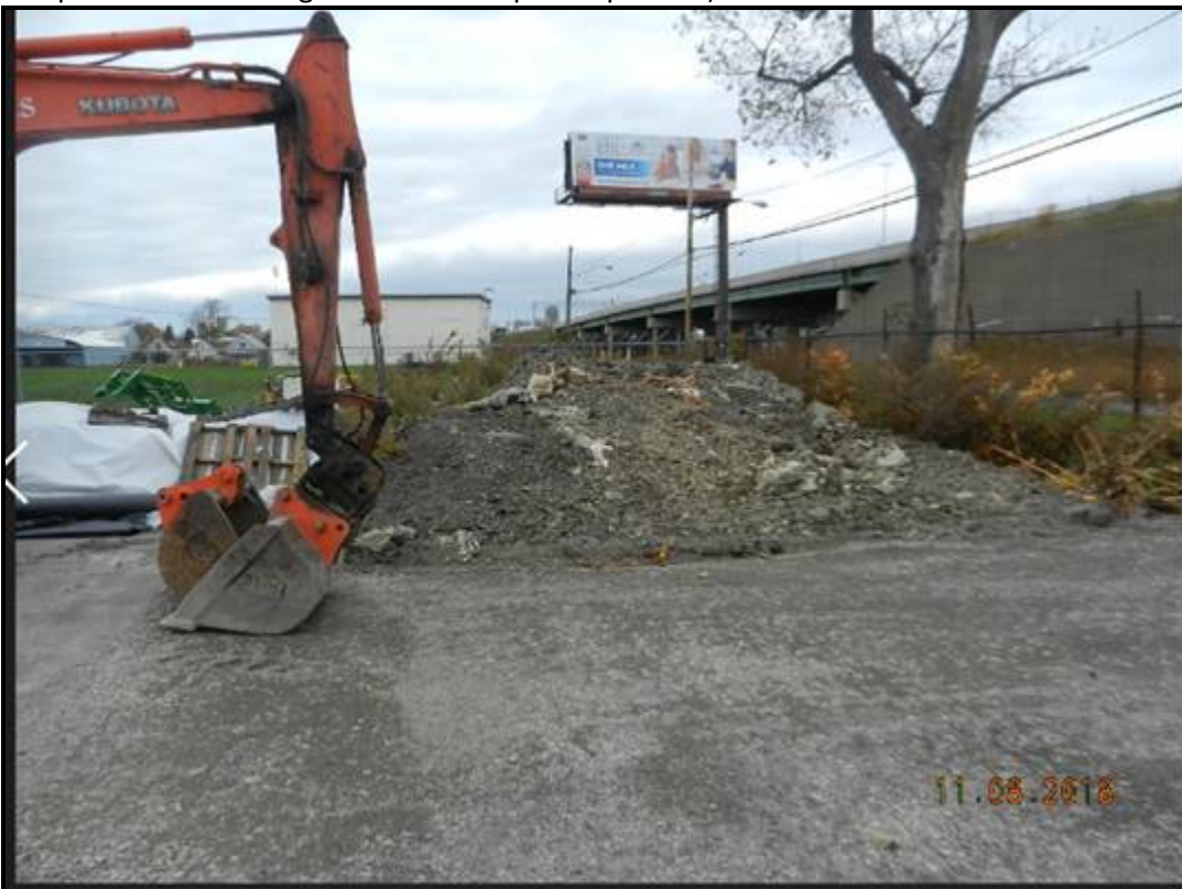
Picture #3: The soil pile shown in the picture below is residual soil from past projects, previously sampled, analyzed and approved for re-use on-site. The plan is to send this soil to the Chaffee Landfill (will be sampled and analyzed again to complete Waste Management's waste profile process).
