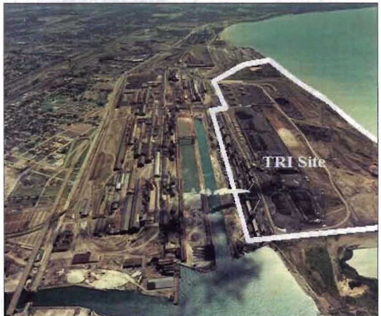
Former Bethlehem Steel Lackawanna (TRI) Site
