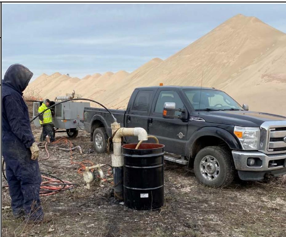
A photograph showing two workers in safety gear (one in a dark suit and one in a yellow vest) operating an air lift pump system. They are connected to a truck-mounted pump unit. A black drum is being filled with liquid from the pump. In the background, there are large piles of brown material, likely sand or soil, under a clear sky. |  |
