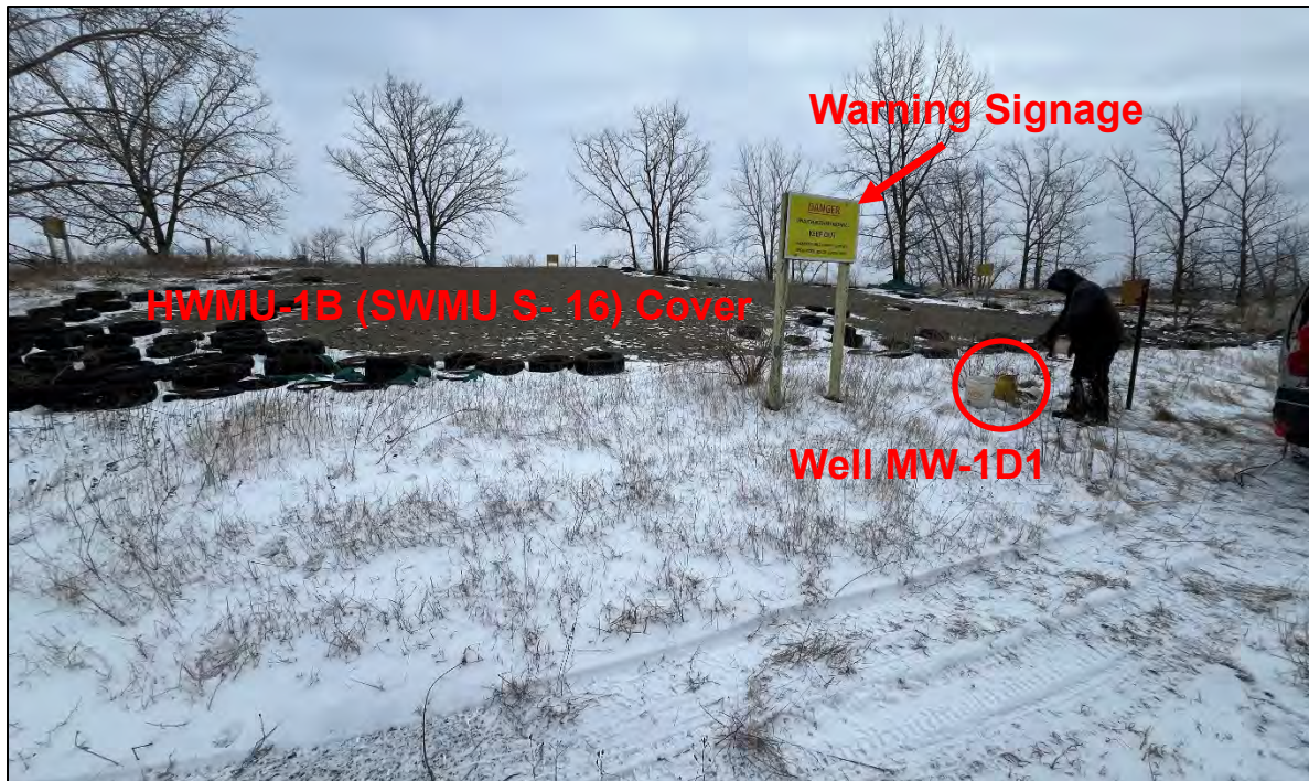
Eastward view of temporary cover on HWMU-1B (SWMU S-16) and purging/sampling at well MW-1D1.
