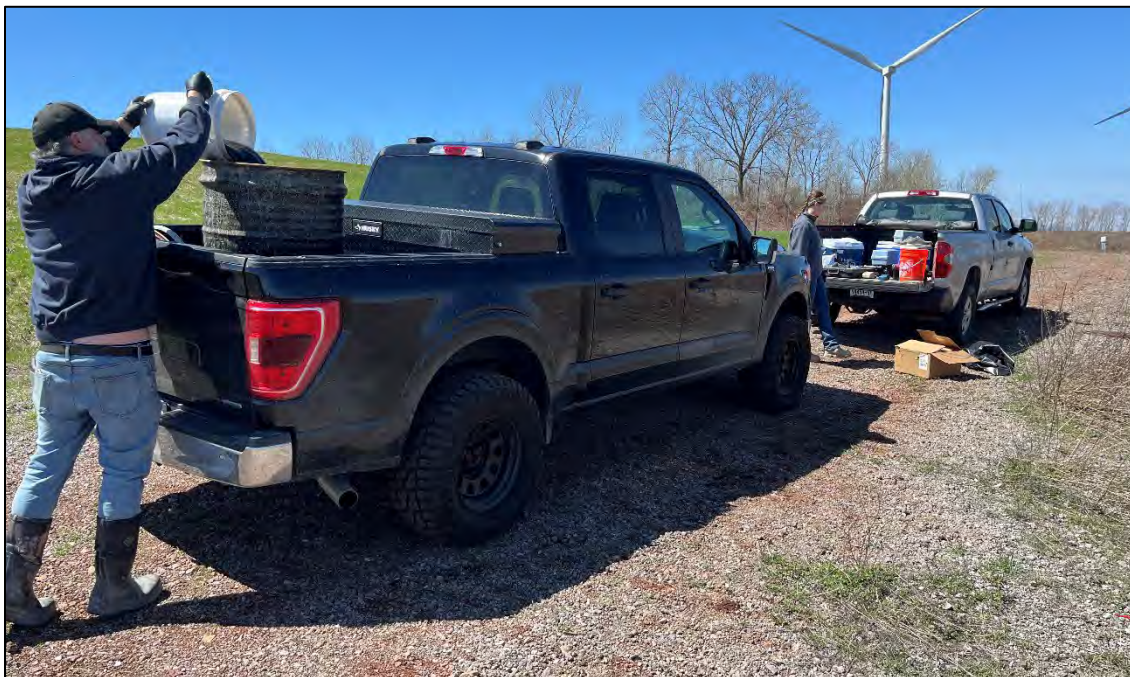
Pouring collected purge water into a 55-gallon drum for transport to the ATP Pretreatment System for processing. Grassy ATP-ECM containment cell in background.
