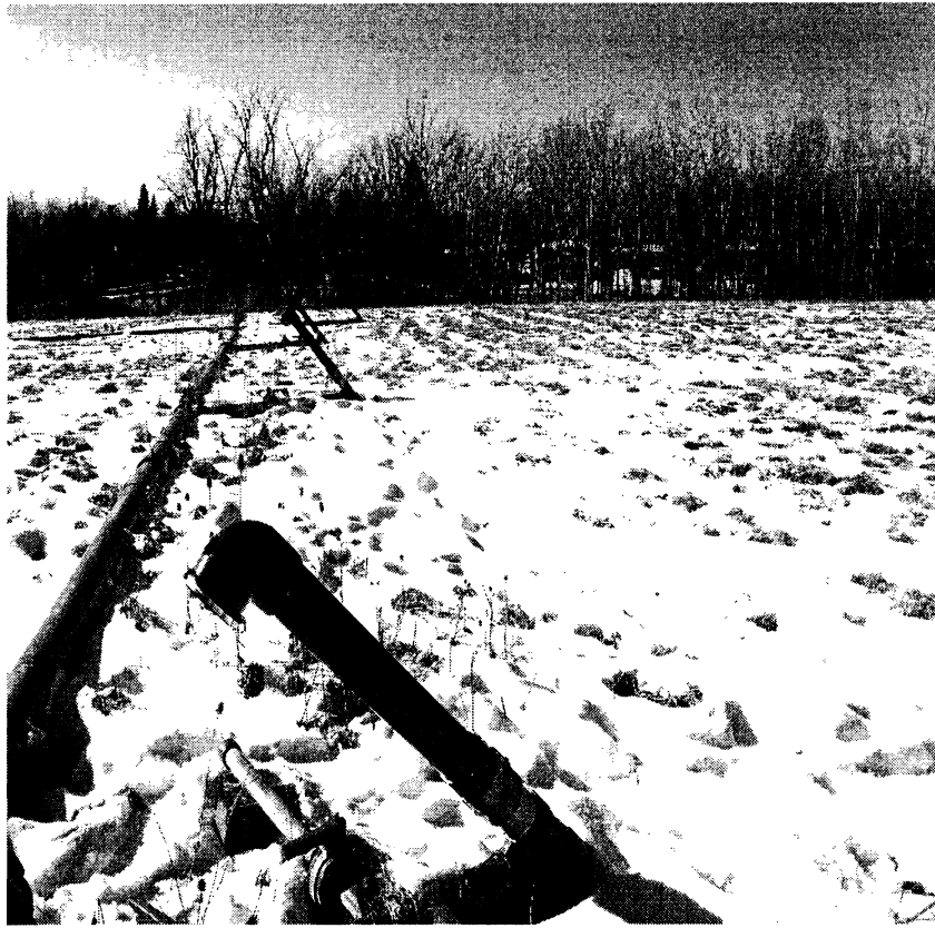
Photo 4 – First five installed vent risers
