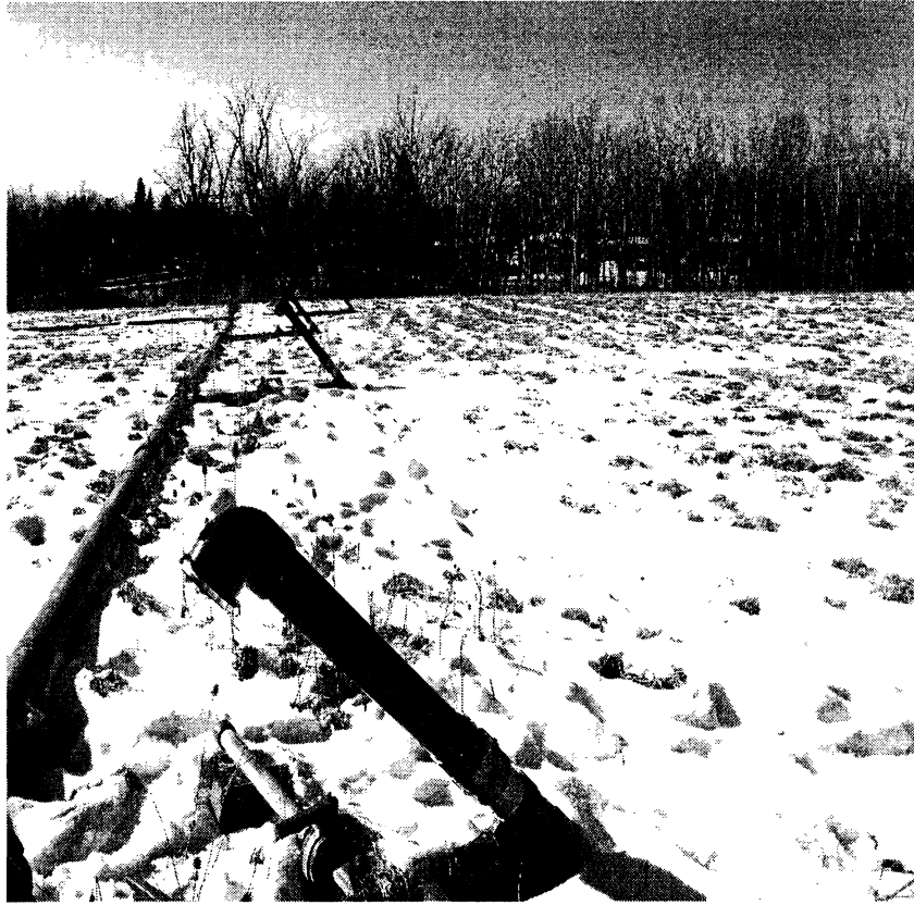
Photo 4 – First five installed vent risers
