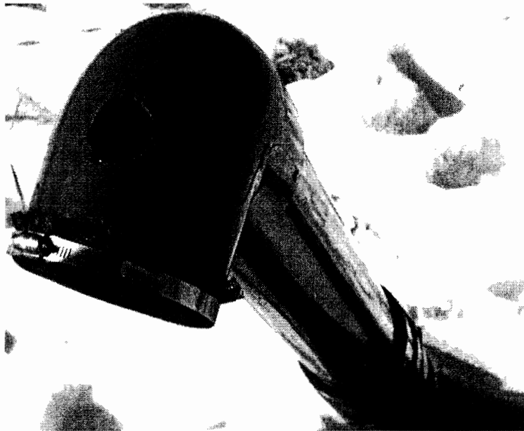
Photo 2 – Drilled sample port w/o expandable plug
