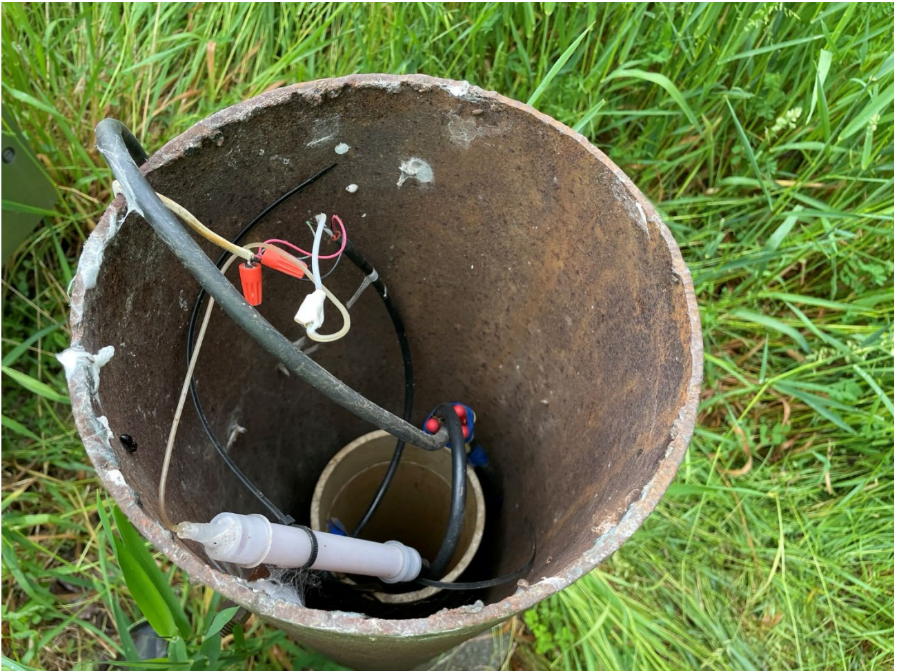
Inside of extraction well EW-1.
