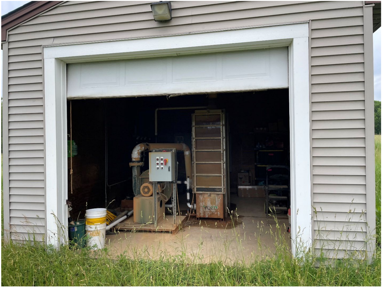
Water treatment building.
