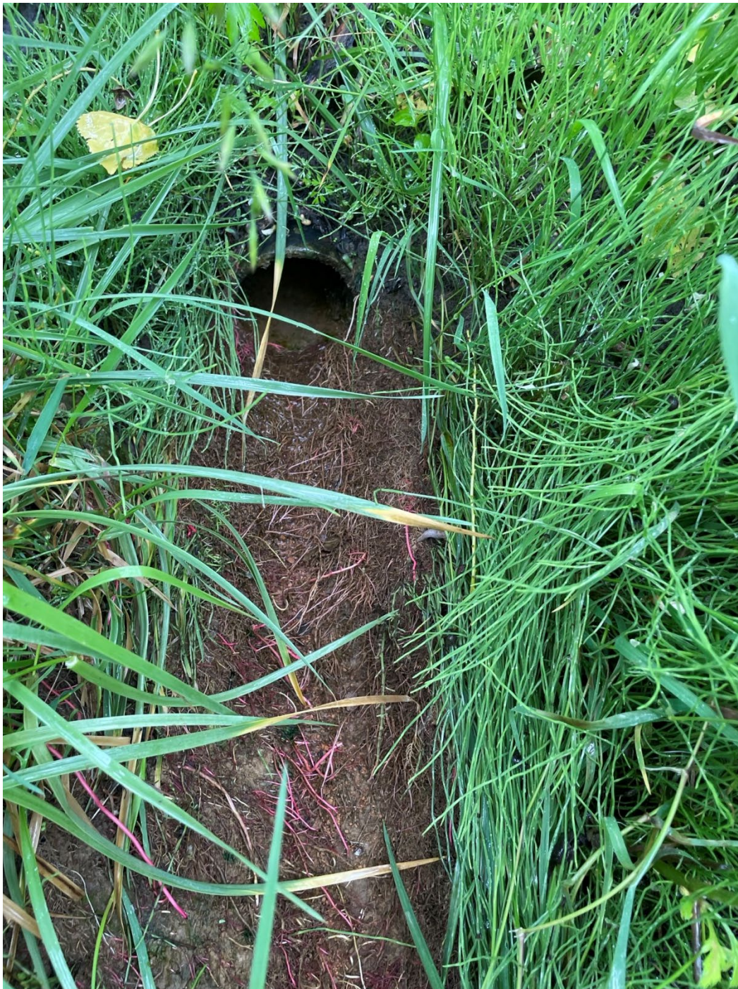
Site treatment system outfall line.
