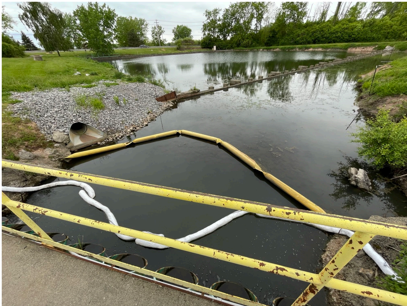
Oil boom (precautionary measure) leading to settling pond between Areas A and B.
