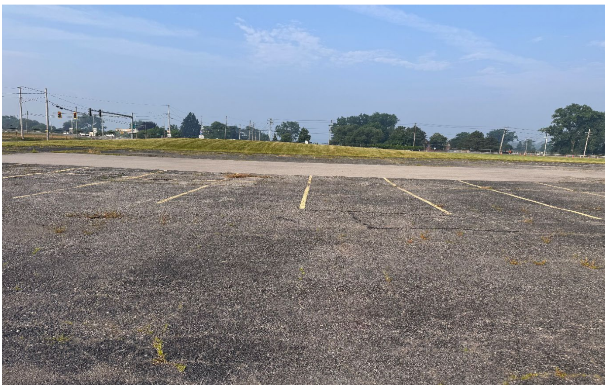
Area B Facing West
