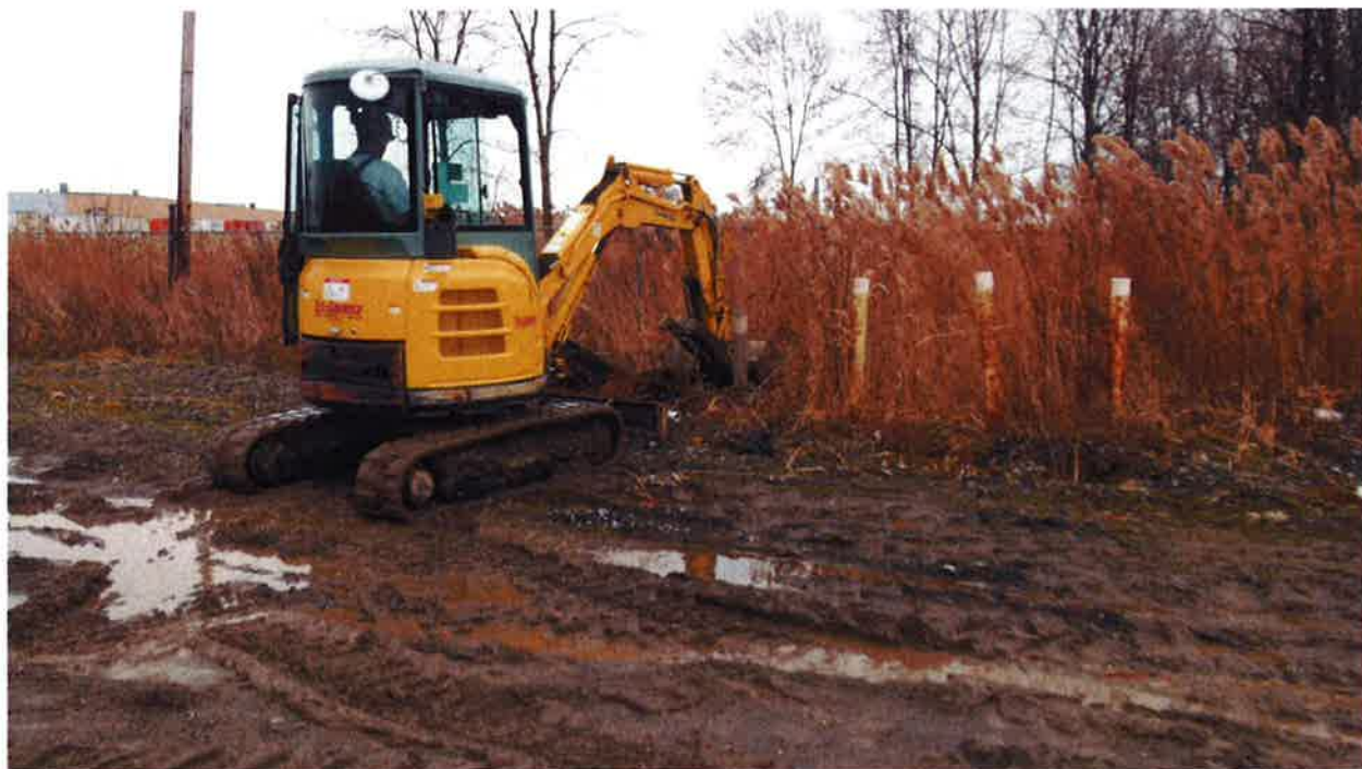
Photo #19: View of the removal of wells MW-04S and MW-03D.
