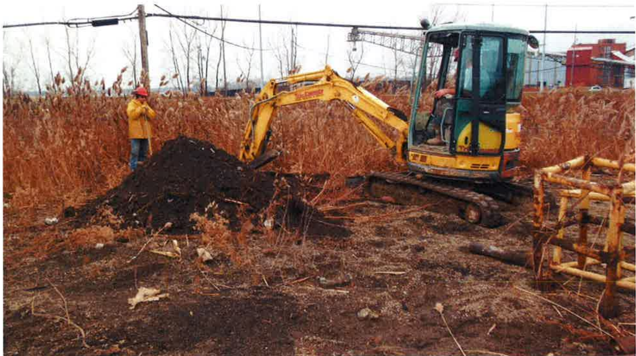
Photo #16: Excavator continuing to dig to remove MW-06DD.
