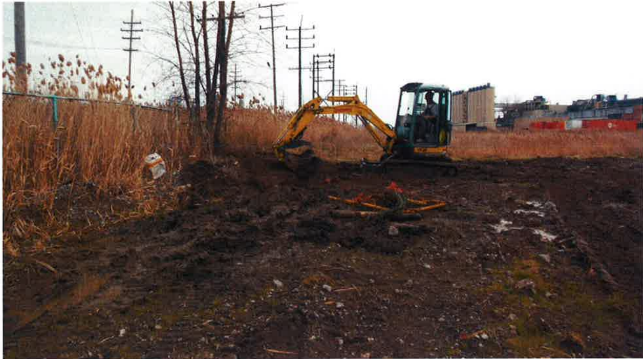
Photo #14: Excavator removing the remaining portion of MW-05S.
