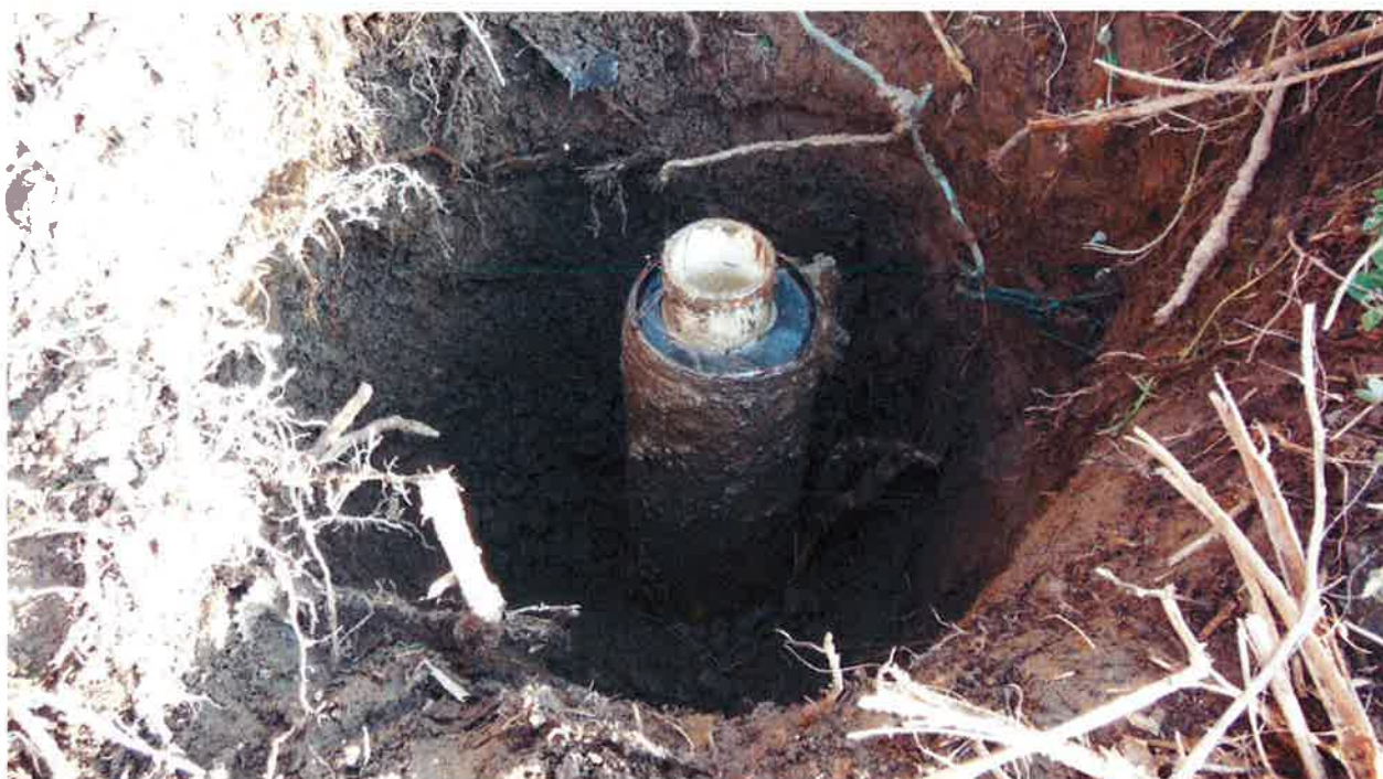
Photo #12: View of MW-05S before it was removed with excavator.
