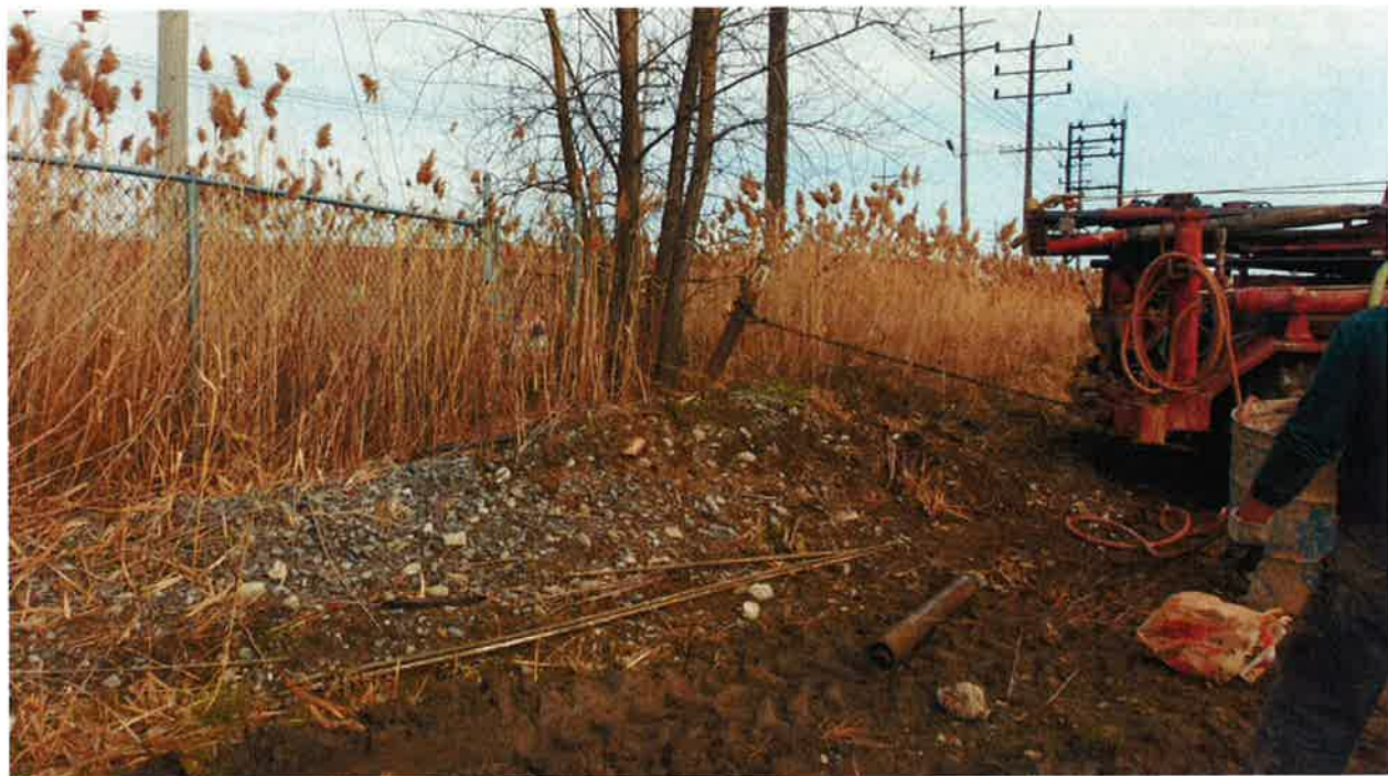
Photo #10: Drilling rig pulling MW-06D.
