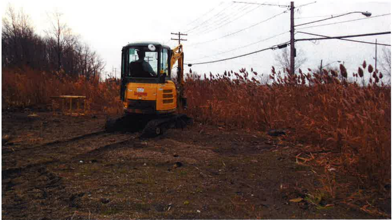
Photo #15: Excavator removing MW-06DD.
