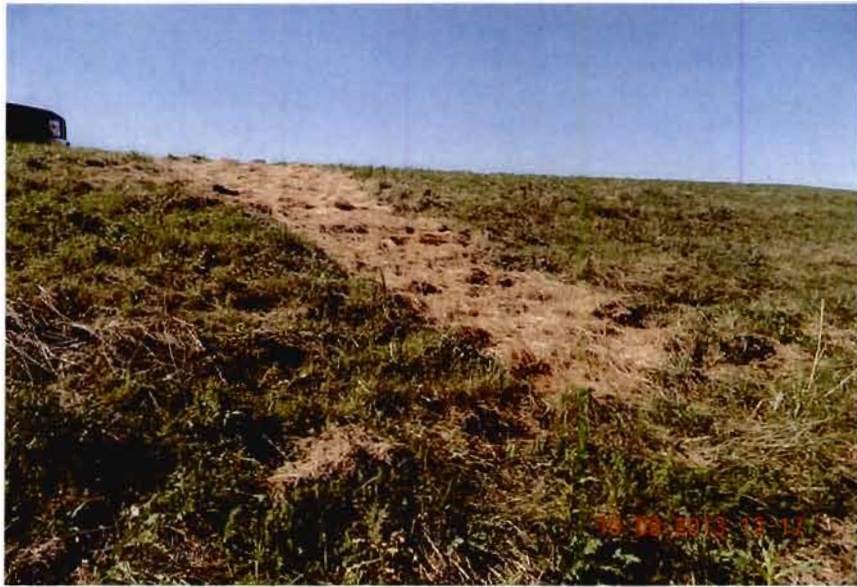
BACKFILLED, SEEDED AND MULCHED BURROW LOCATION (on slope)
