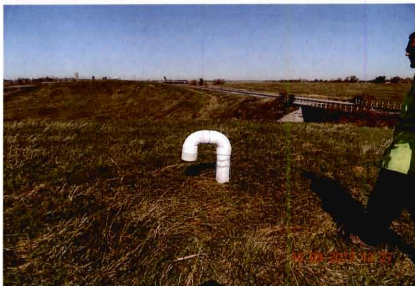
REPAIRED GAS VENT GOOSE NECK (west)
