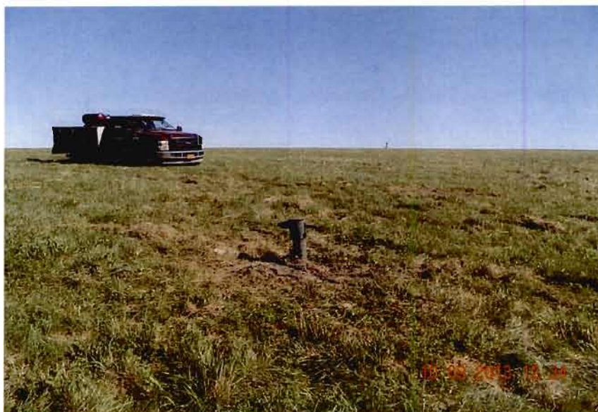
STRAIGHTENED CASING AT MW-14BR
