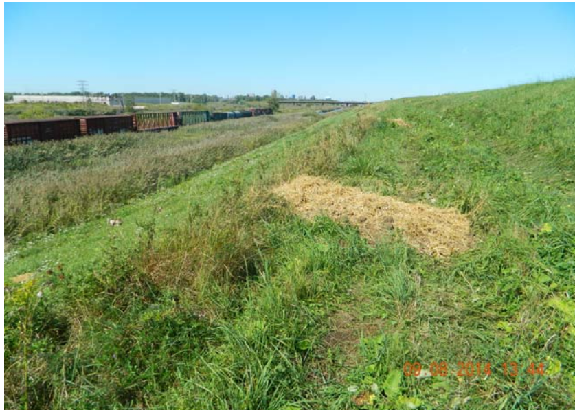
Backfilled, seeded, and mulched animal burrow hole along west side of BOF Dust Area between MW-7B and MW-10B
