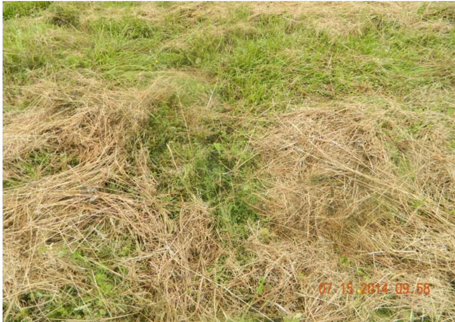
Start of small erosion gullies along northeast side of Miscellaneous Debris Area between access road and MW-12B
