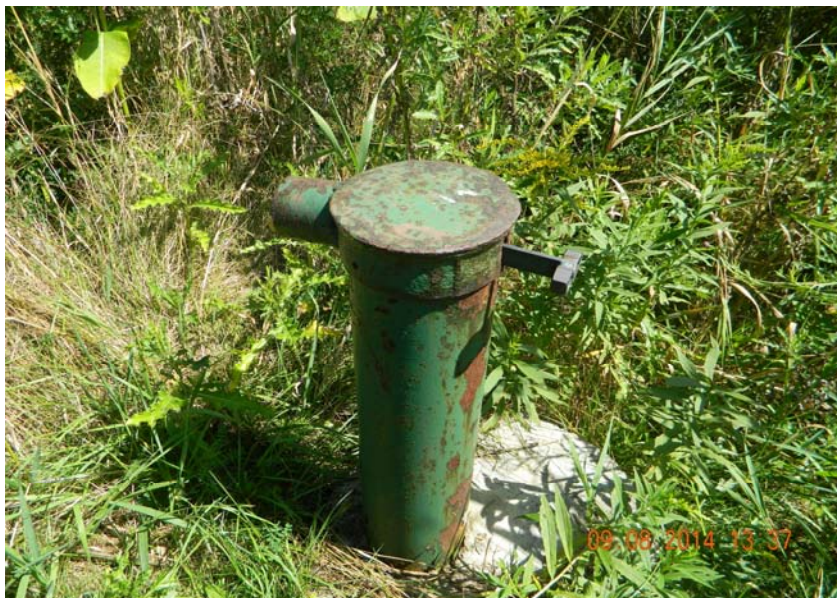
Repaired well cap anchor bolt on MW-4A
