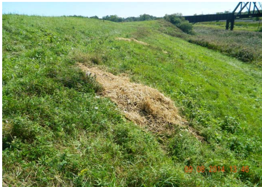
Backfilled, seeded, and mulched animal burrow hole along west side of BOF Dust Area. Approximately 40 feet south of PVC gas vent
