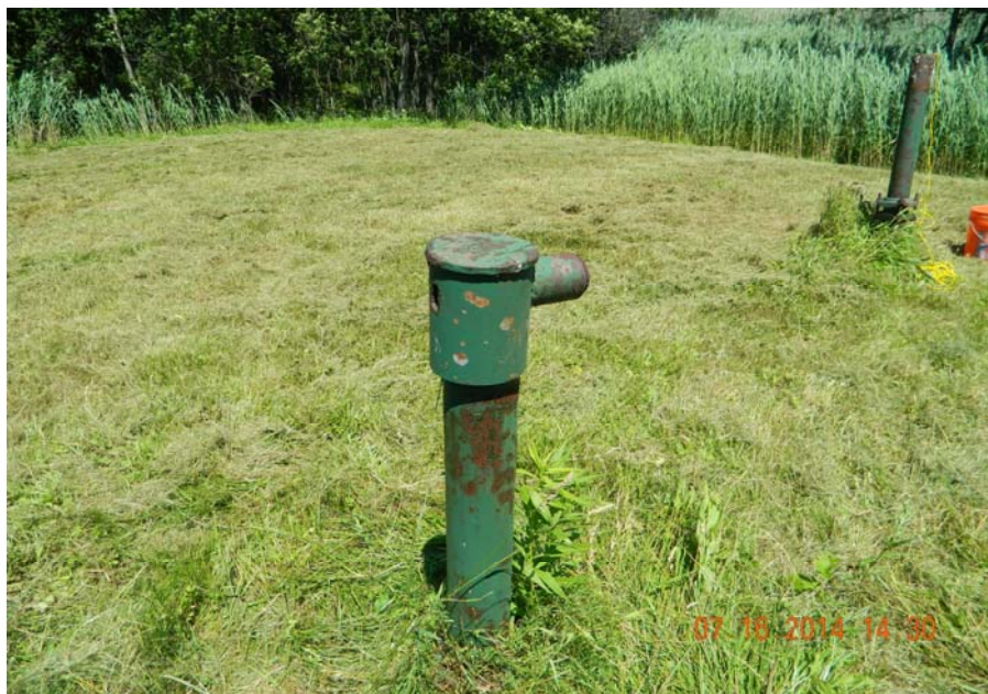
No well cap anchor bolt or lock on MW-6B
