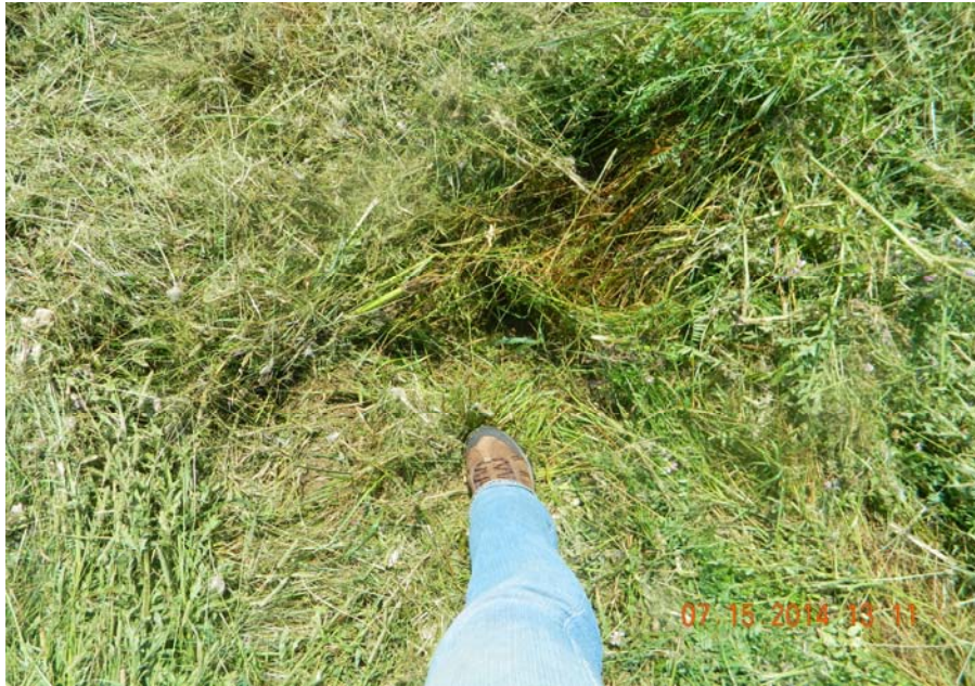
Animal burrow hole along west side of BOF Dust Area. Approximately 40 feet south of PVC gas vent
