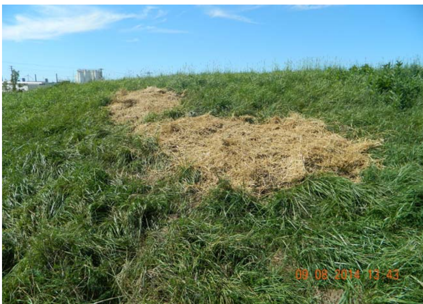
Backfilled, seeded, and mulched animal burrow hole along southeast side of BOF Dust Area
