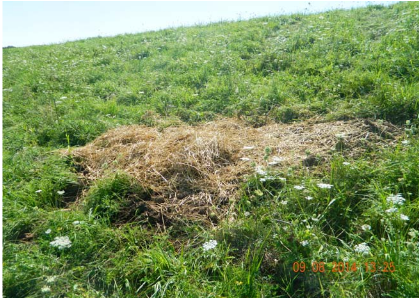
Backfilled, seeded, and mulched animal burrow hole along northeast side of Miscellaneous Debris Area between access road and MW-12B
