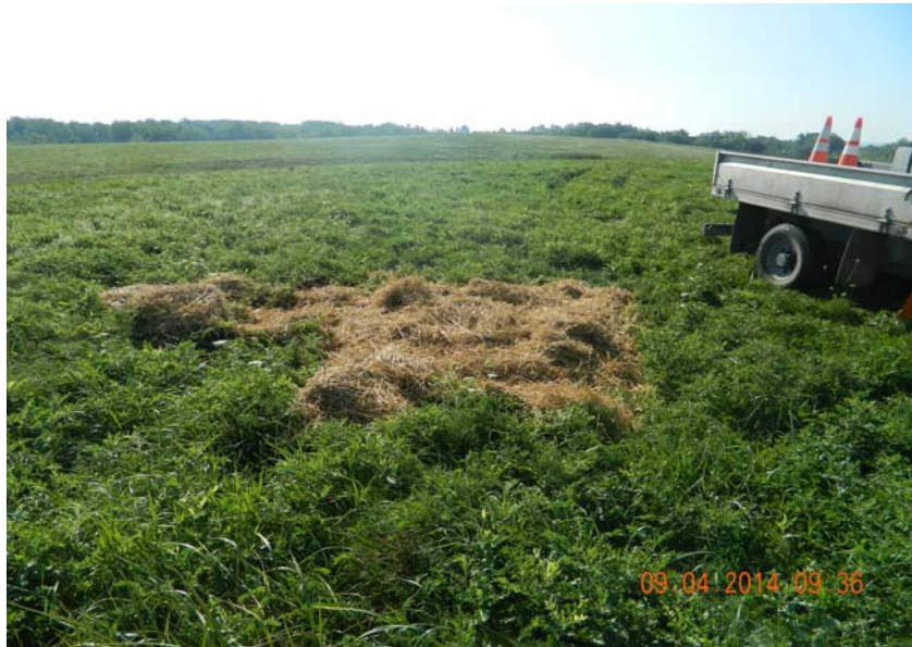
Backfilled, seeded, and mulched 2 holes on top of BOF Dust Area. Approximately 40 feet south of PVC gas vent
