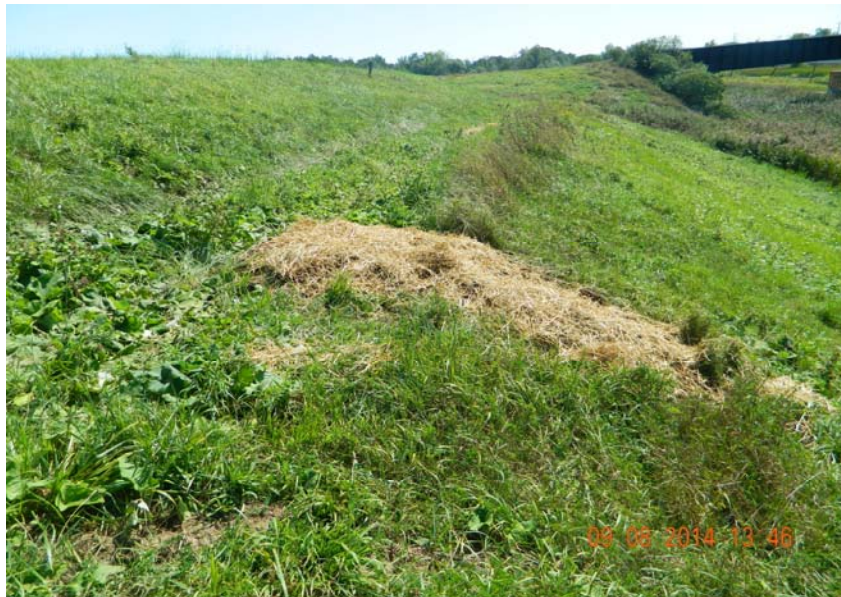
Backfilled, seeded, and mulched erosion along west side of BOF Dust Area where grade becomes steeper
