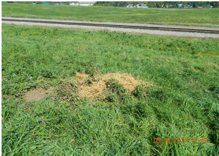
Backfilled, seeded, and mulched animal burrow hole along northeast side of BOF Dust Area. Approximately 40 feet south of PVC gas vent
