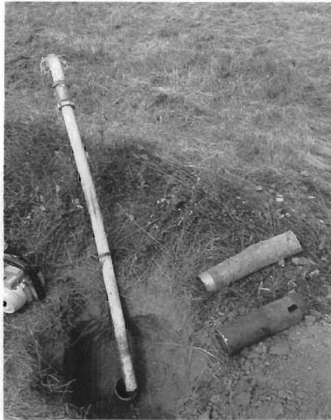
Investigation of MW-14BR
