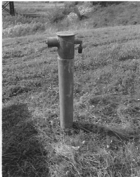
Repaired Cap at MW-14BR
