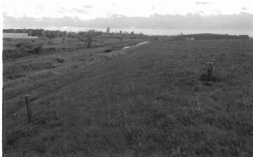
Looking Northwest at MW18A and MW-18B
