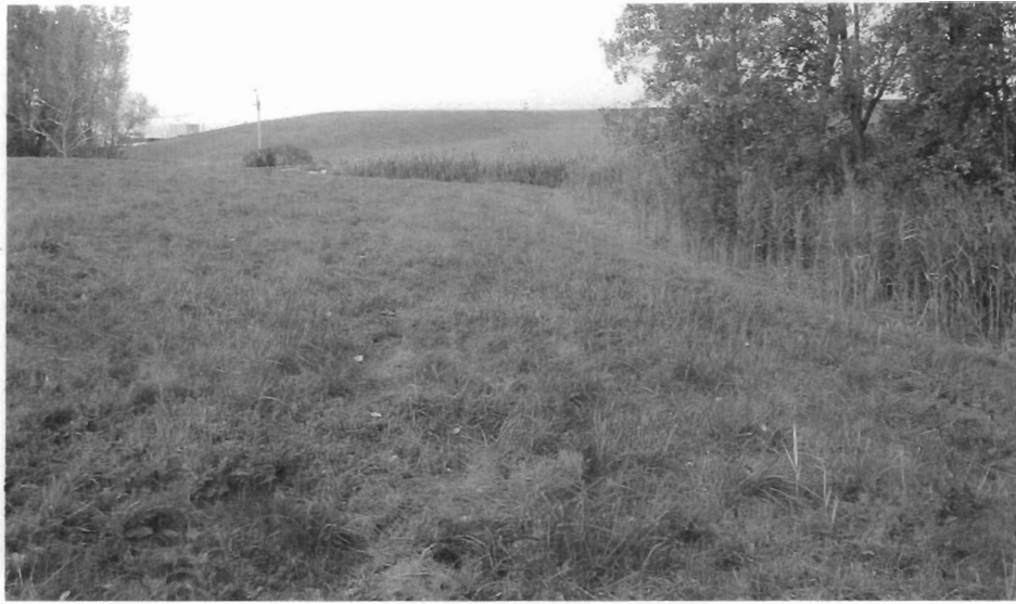
Looking West at the North Slope of the Miscellaneous Debris Area
