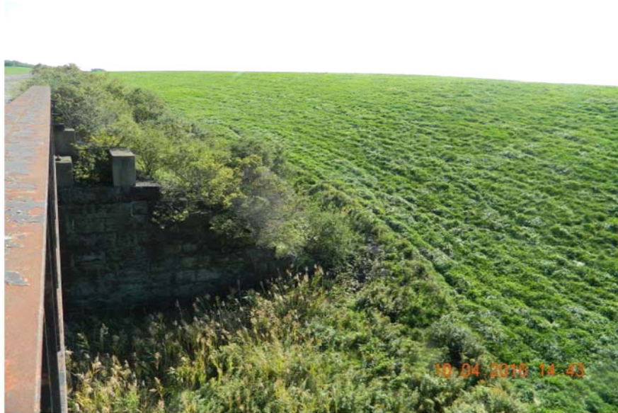
NORTHWEST SLOPE OF CLARIFIER SLUDGE AREA
