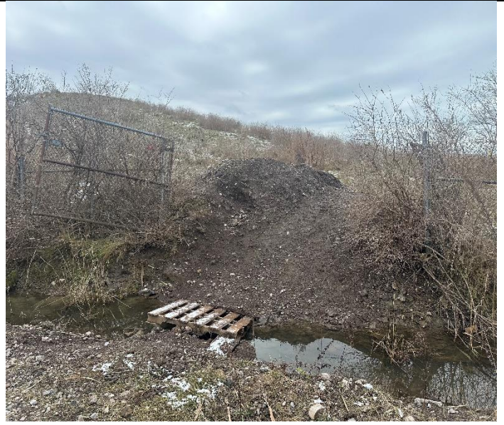
Opened/Damaged gate near northern ponds
