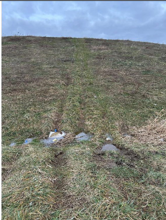
Rutting near MW-4A/B
