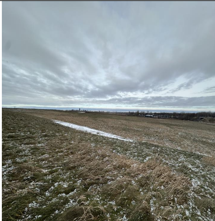
View of cover system looking North
