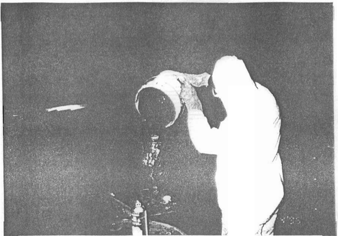
TRANSFER OF OIL TO DRUMS FOR DISPOSAL
