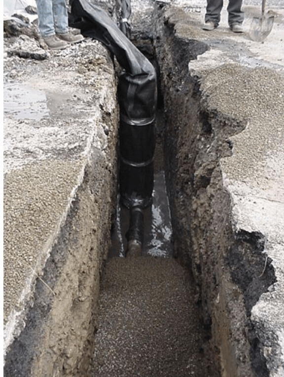
Figure 2-6. Photograph showing the dewatering pipe installed in the SWMU 38 excavation area. View looking southeast. Photograph taken by Glenn May on May 7, 2004.
