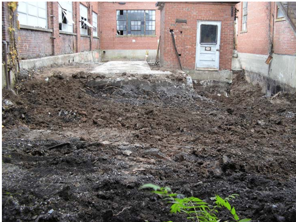
Figure 4-16. Photograph showing the east end of the courtyard following the removal of 1 foot of hazardous soils. View looking southwest. Photograph taken by Jim Tuk on October 19, 2005.
