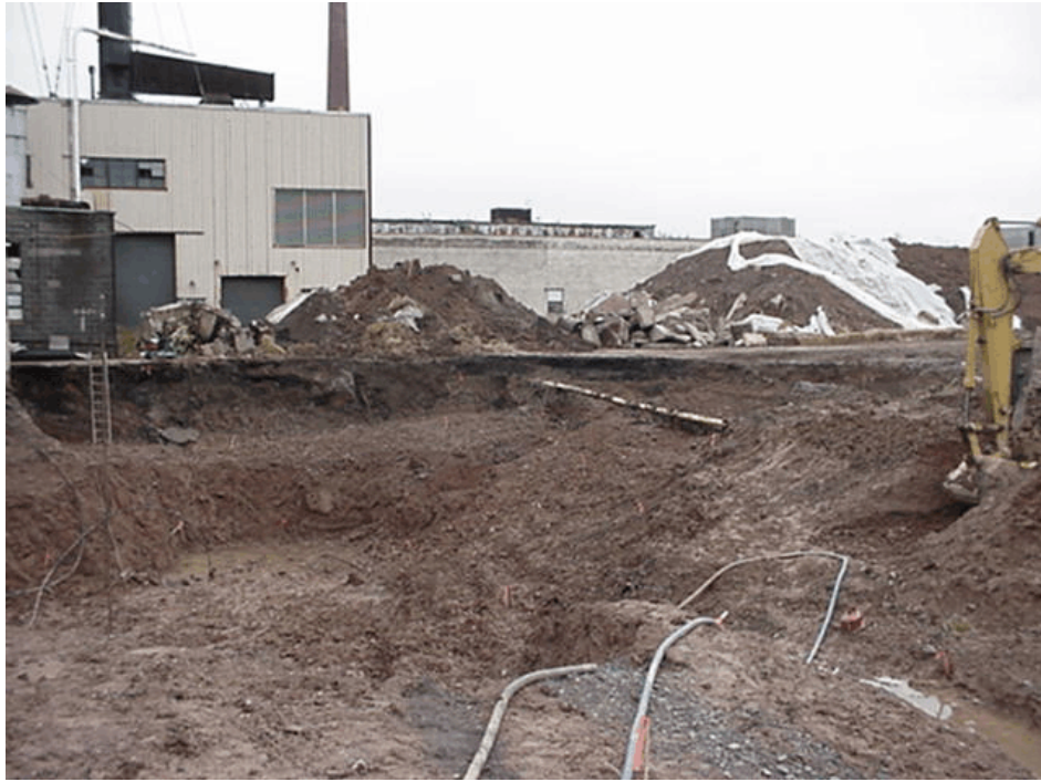
Figure 2-42. Photograph showing the excavation of the trench as part of the Roadway Ditch remediation. The SWMU 38 excavation is located to the left of the excavator, while the contaminated soil stockpile can be observed in the background. View looking east. Photograph taken by Glenn May on October 22, 2004.
