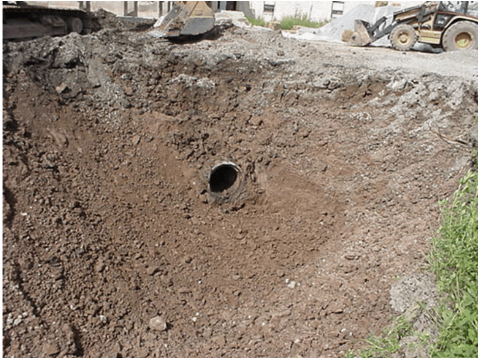
Figure 2-25. Photograph showing the outflow pipe from the south arm of the “U” shaped Settling Lagoon (SWMU 12) to the K-Line sewer. View looking north. Photograph taken by Glenn May on August 6, 2004.
