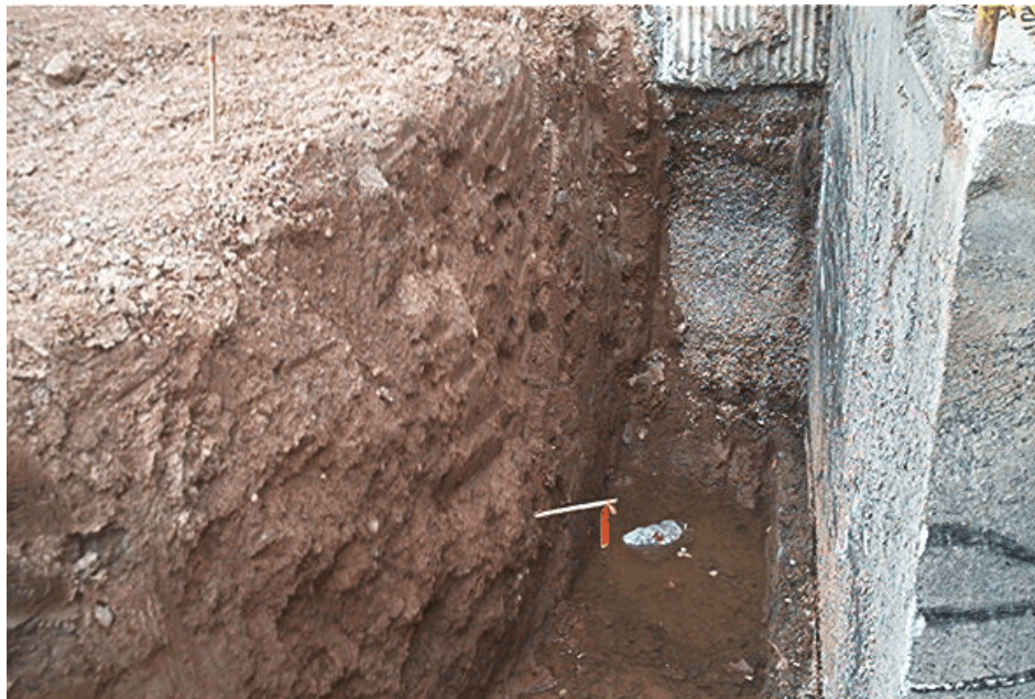
Figure 2-61. Photograph showing the final excavation along the Spauldite Sheet basement stairwell. The crushed stone in the background contains NAPL, but could not be removed during the Phase 1 IRM due to an adjacent building. View looking west. Photograph taken by Glenn May on October 11, 2004.
