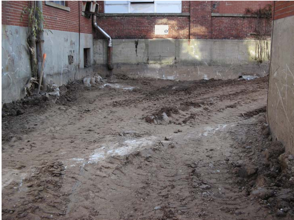
Figure 4-27. Photograph showing the completed backfilling of the deep excavation at the east end of the courtyard. View looking southeast. Photograph taken by Jim Tuk on November 3, 2005.
