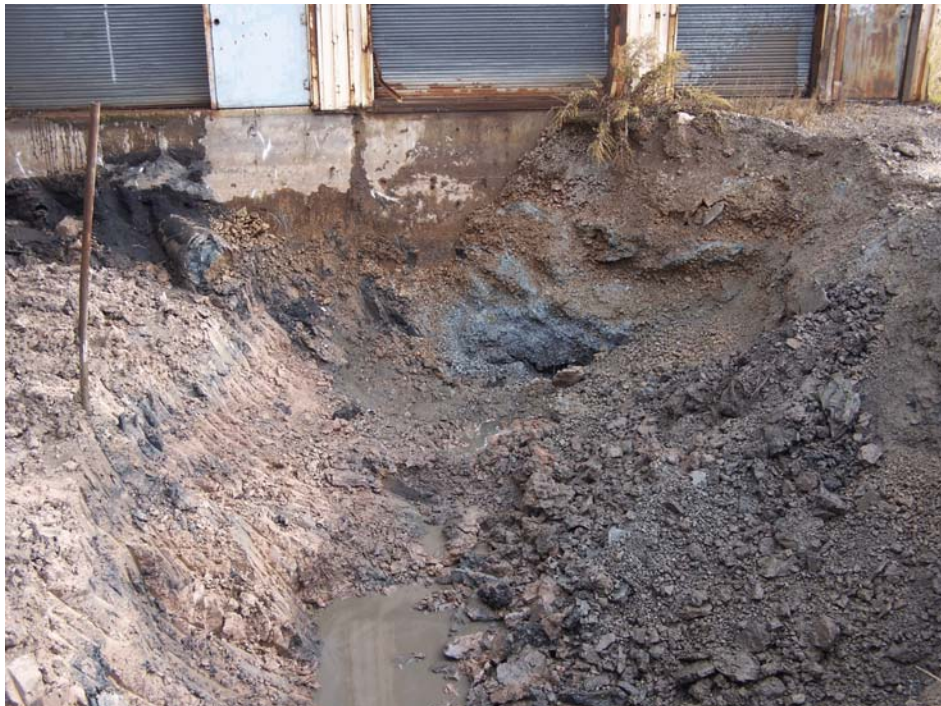
Figure 4-73. Photograph showing the SWMU 11 excavation. Note the inflow pipe to the lagoon and the fill material under the Boiler House. View looking northeast. Photograph taken by Glenn May on October 24, 2006.
