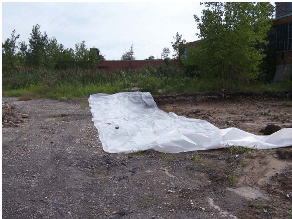
Figure 4-30. Photograph showing the placement of poly over the sidewalls of the excavation to form a demarcation layer. View looking northeast. Photograph taken by Glenn May on September 6, 2006.
