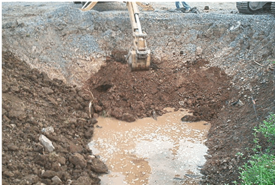
Figure 2-32. Photograph showing the outflow pipe from the south arm of the “U” shaped Settling Lagoon (SWMU 12) being plugged with native silty clay. View looking northeast. Photograph taken by Glenn May on August 27, 2004.
