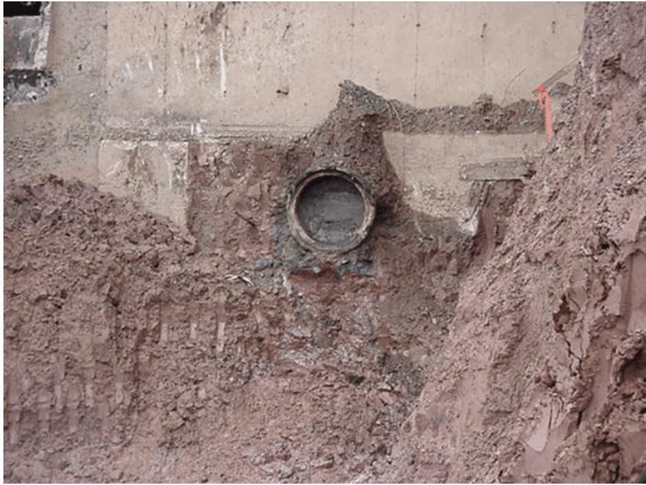
Figure 2-54. Photograph showing the K-Line storm sewer near the former Therminol Building after it was plugged with bricks and mortar. View looking northwest. Photograph taken by Glenn May on October 21, 2004.
