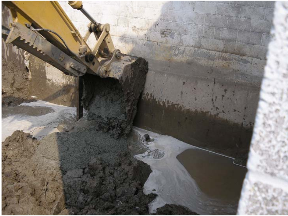
Figure 2-56. Photograph showing the concrete being poured into the form around the K-Line storm sewer. View looking northwest. Photograph taken by Glenn May on June 10, 2005.
