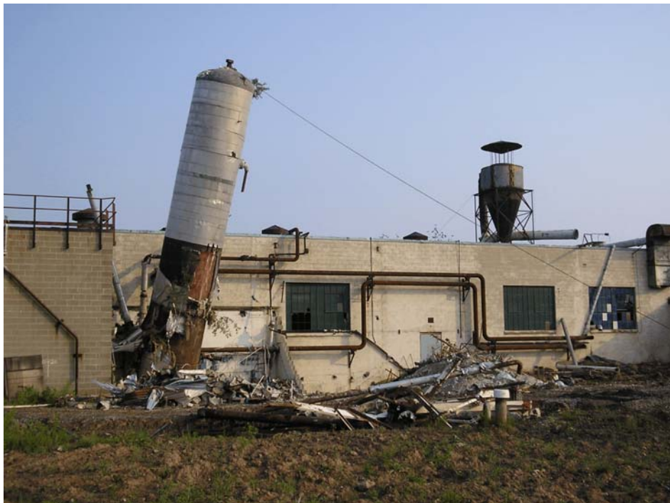
Figure 4-8. Photograph showing the last Supertherm Tank being pulled to the ground. View looking north. Photograph taken by Glenn May on August 3, 2005.
