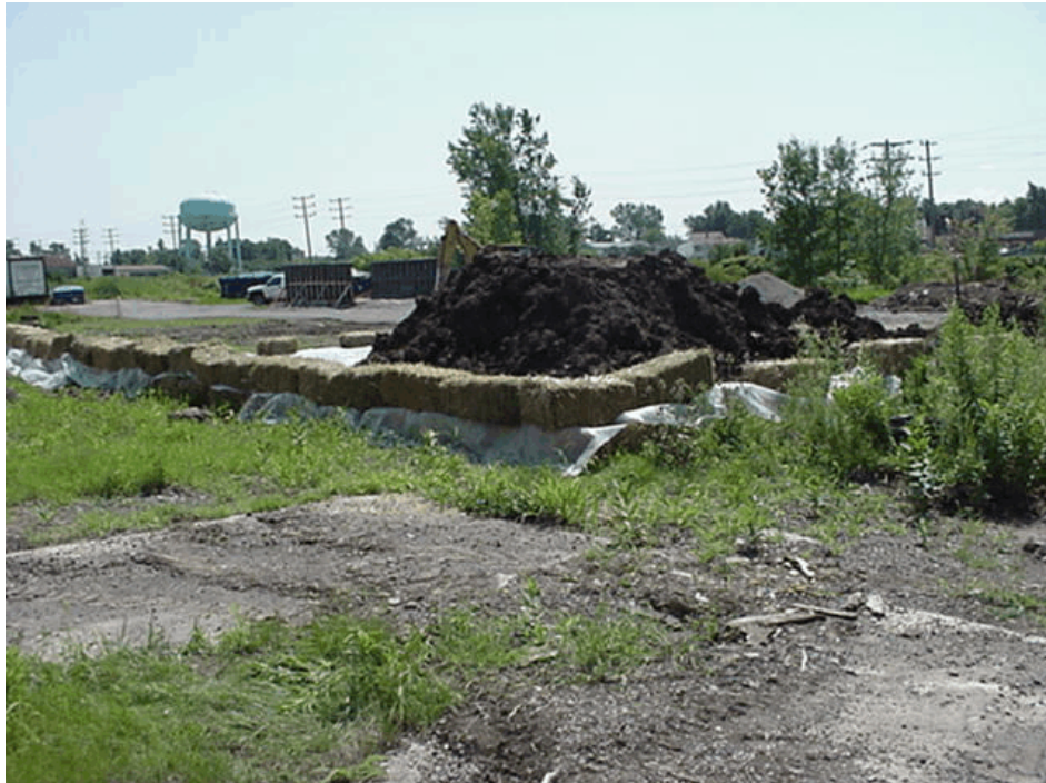
Figure 2-29. Photograph showing the soil staging pad being constructed over the SWMU 23 area. View looking south. Photograph taken by Glenn May on August 3, 2004.
