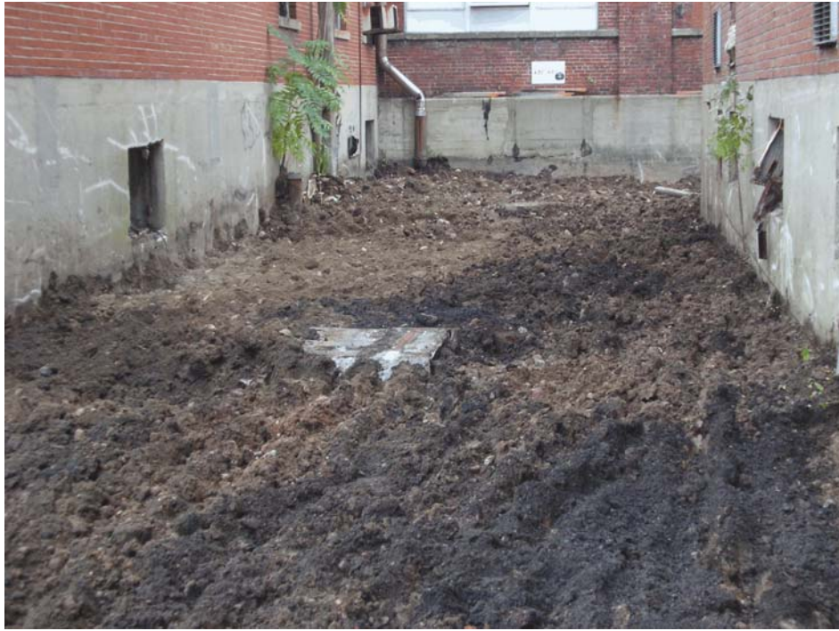
Figure 4-17. Photograph showing the alleyway following the removal of 1 foot of hazardous soils. View looking southeast. Photograph taken by Jim Tuk on October 20, 2005.
