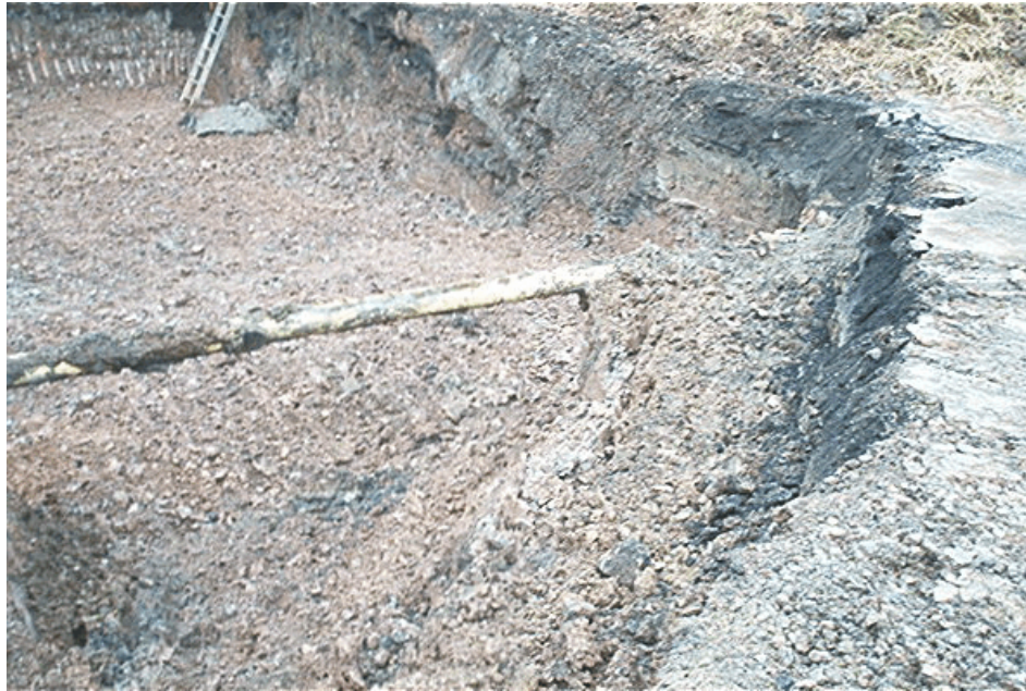
Figure 2-67. Photograph showing the fill material in the east wall of the Therminol Building excavation. This fill is associated with the SWMU 11 Settling Lagoon. View looking north. Photograph taken by Glenn May on October 22, 2004.
