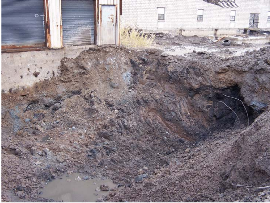
Figure 4-74. Photograph showing the SWMU 11 excavation. Note the fill material in the south sidewall, which was the location of a former ditch. View looking east. Photograph taken by Glenn May on October 24, 2006.
