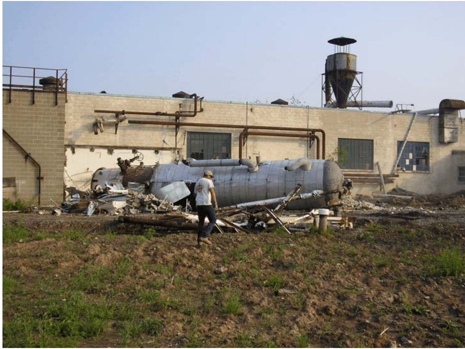
Figure 4-9. Photograph showing the last Supertherm Tank after being pulled to the ground. View looking north. Photograph taken by Glenn May on August 3, 2005.
