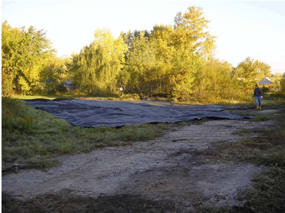
Figure 4-25. Photograph showing the placement of geofabric on the ground surface during construction of the truck turnaround. View looking north. Photograph taken by Jim Tuk on October 28, 2005.
