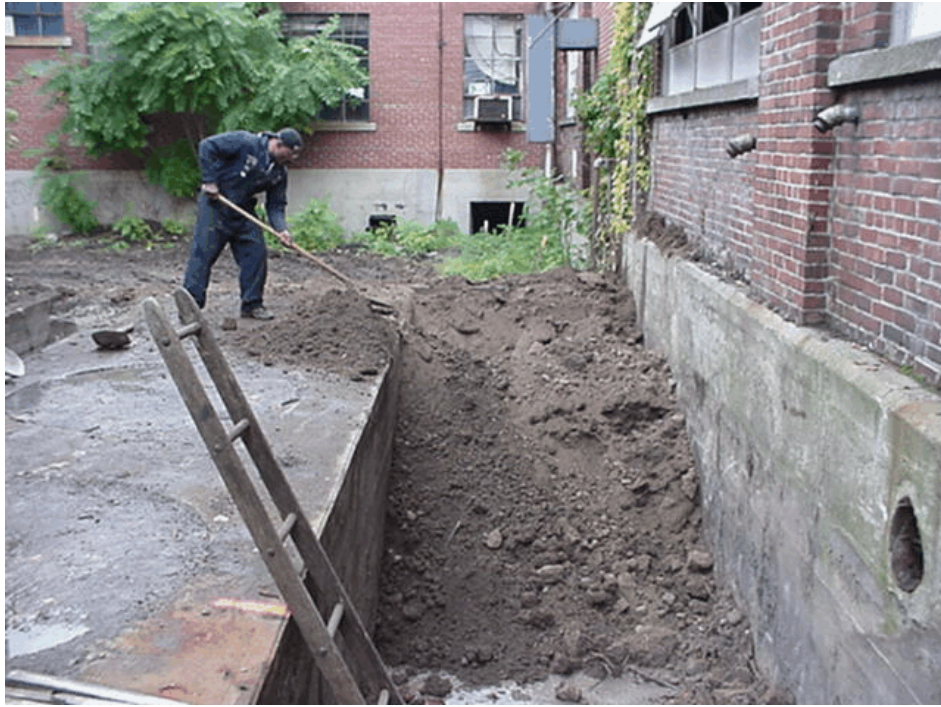
Figure 4-13. Photograph showing the initial backfilling around the concrete pad. View looking northeast. Photograph taken by Glenn May on October 12, 2005.
