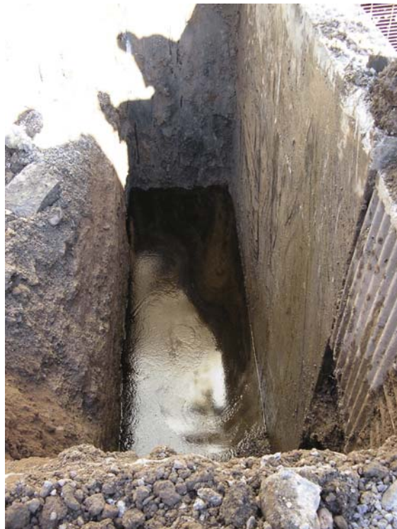
Figure 4-33. Photograph showing NAPL in the excavation along the Spauldite Sheet basement stairwell. View looking slightly northwest. Photograph taken by Glenn May on October 5, 2006.
