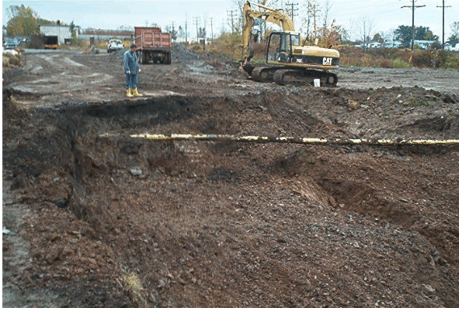
Figure 2-66. Photograph showing the southeastern limit of the Therminol Building excavation. Note the black cinders and ash underlying the roadway. View looking southeast. Photograph taken by Glenn May on October 22, 2004.
