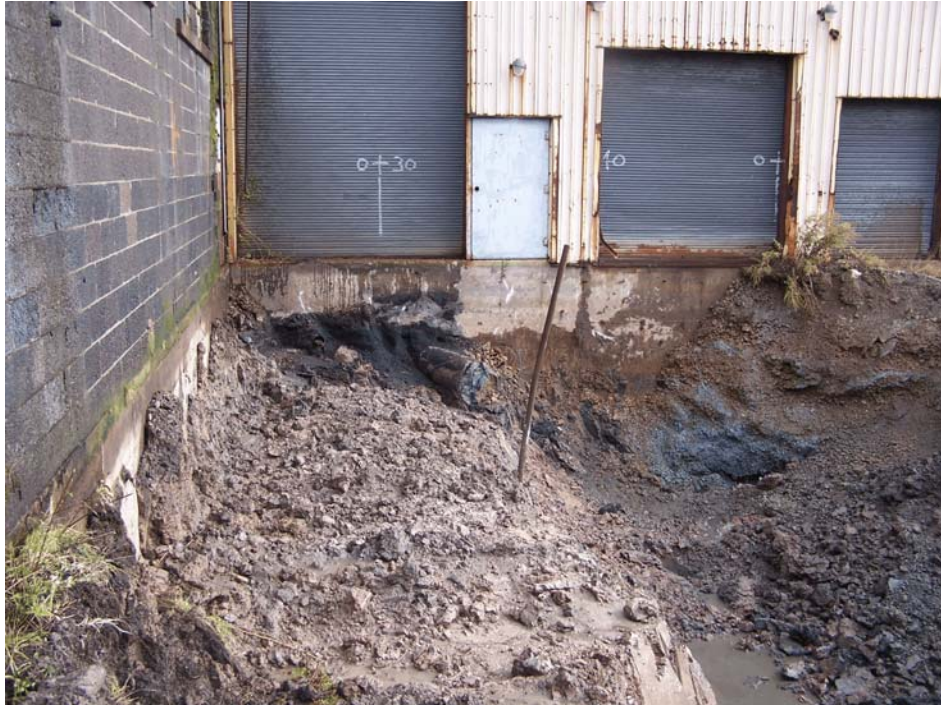
Figure 4-72. Photograph showing the SWMU 11 excavation. Note the inflow pipe to the Small Settling Lagoon and the fill material under the Boiler House. View looking northeast. Photograph taken by Glenn May on October 24, 2006.
