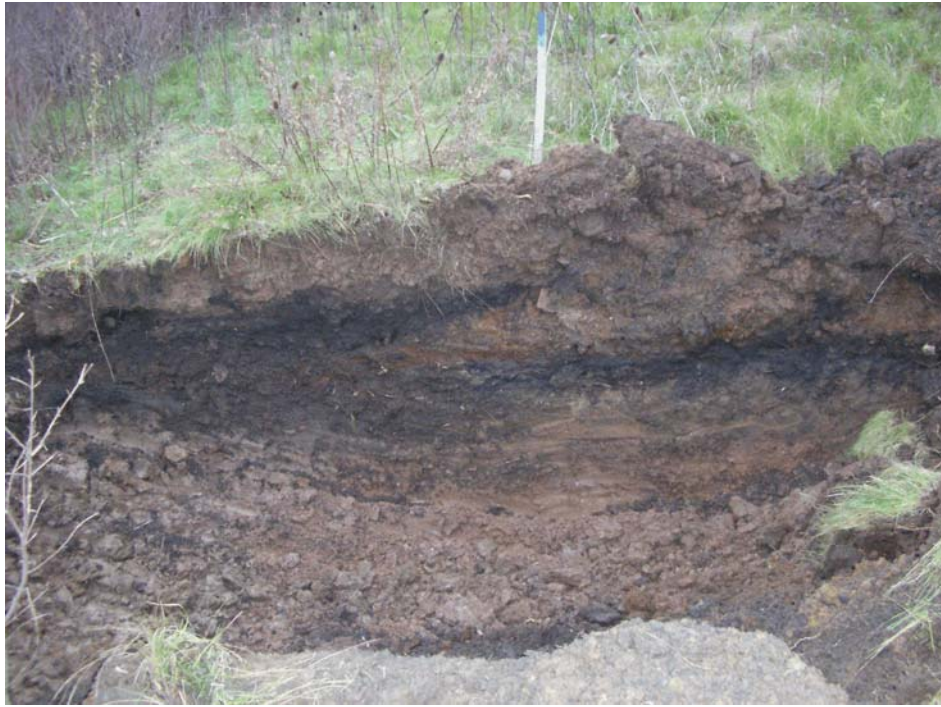
Figure 4-45. Photograph showing the fill material encountered in the SWMU 13 excavation. The mounded area in the background is the Resin Drum Landfill (SWMU 7). View looking southwest. Photograph taken by Jim Tuk on November 21, 2005.
