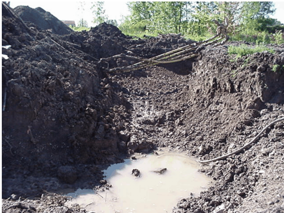
Figure 2-34. Photograph showing the continued excavation of the Southeast Ditch. The pipes in the background conveyed fuel oil from a tank farm located to the right of this photo to the Boiler House. View looking southeast. Photograph taken by Glenn May on September 1, 2004.
