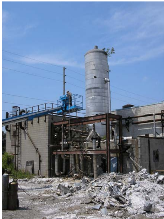
Figure 4-4. Photograph showing the remaining piping, pipe supports and Supertherm Tank. View looking northwest. Photograph taken by Glenn May on August 1, 2005.
