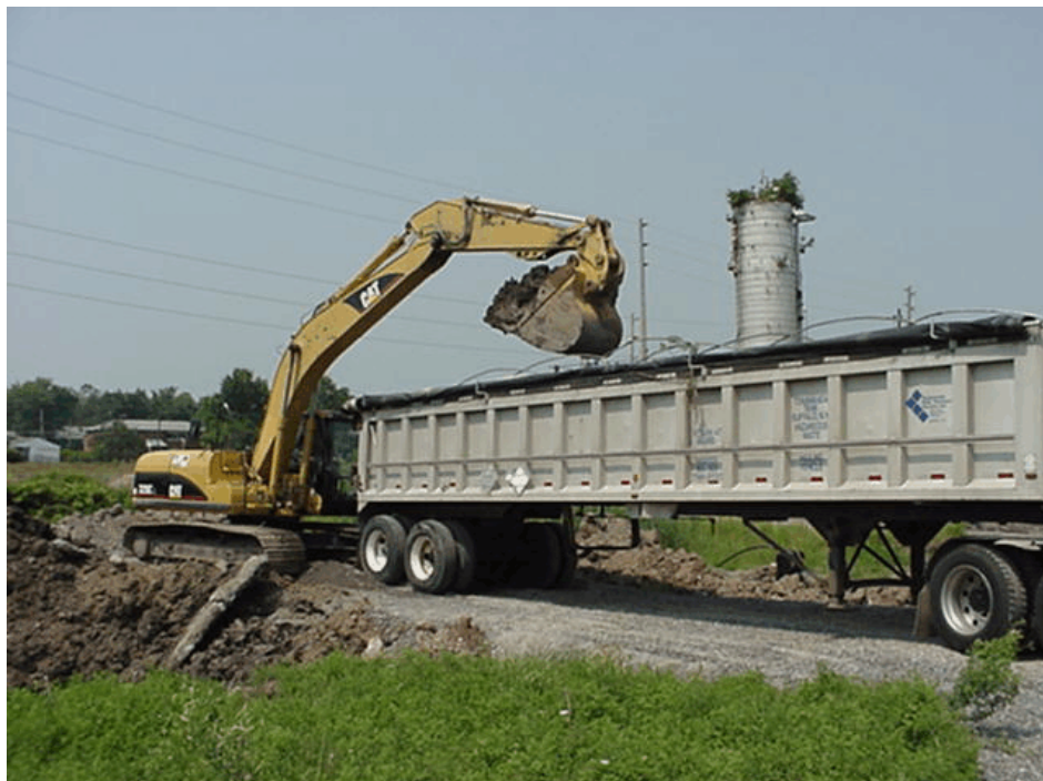
Figure 2-28. Photograph showing the direct loading of trucks during the initial excavation of SWMU 12. View looking northwest. Photograph taken by Glenn May on July 21, 2004.
