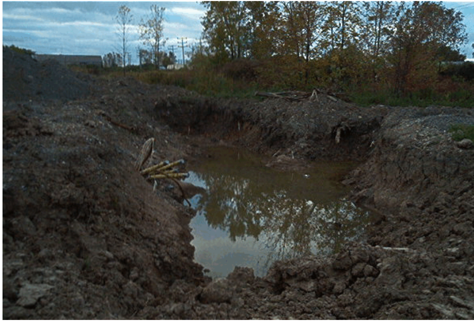
Figure 2-35. Photograph showing the final excavation of the Southeast Ditch. Note that the pipes have been cut and capped. View looking southeast. Photograph taken by Glenn May on October 11, 2004.
