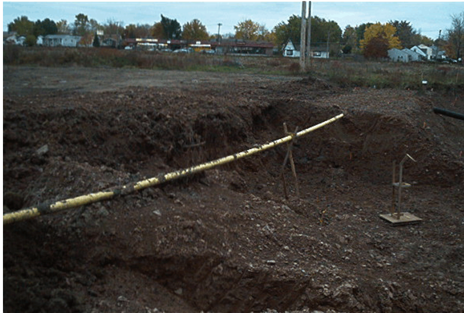
Figure 2-43. Photograph showing the final excavation of the trench associated with the Roadway Ditch. Note the bracing utilized to support the high pressure natural gas pipeline. View looking southwest. Photograph taken by Glenn May on November 1, 2004.
