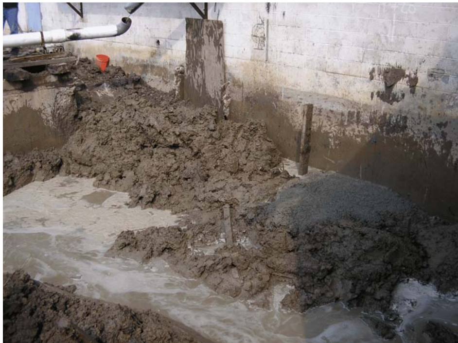
Figure 2-57. Photograph showing the completed concrete plug around the K-Line storm sewer near the former Therminol Building. View looking northwest. Photograph taken by Glenn May on June 10, 2005.
