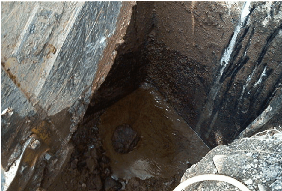
Figure 2-59. Photograph showing the NAPL encountered along the outside wall of the Spauldite Sheet basement. View looking west. Photograph taken by Glenn May on September 28, 2004.
