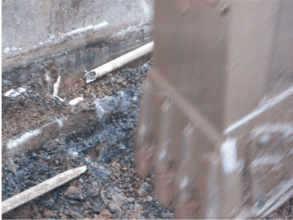
Figure 2-5. Photograph showing NAPL contaminated fill along the west foundation wall of the Spauldite Sheet Basement. Photograph taken by Brian Hutzler on February 12, 2010.
