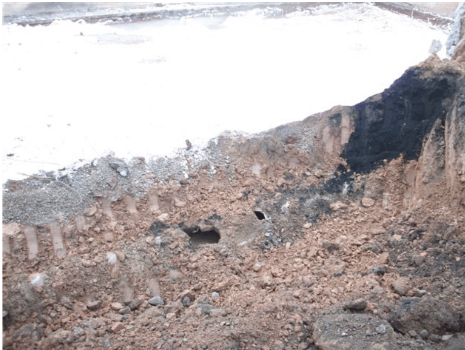
Figure 2-18. Photograph showing the K-Line Storm Sewer and the black fill material overlying the sewer. View looking west. Photograph taken by Brian Hutzler on February 19, 2010.
