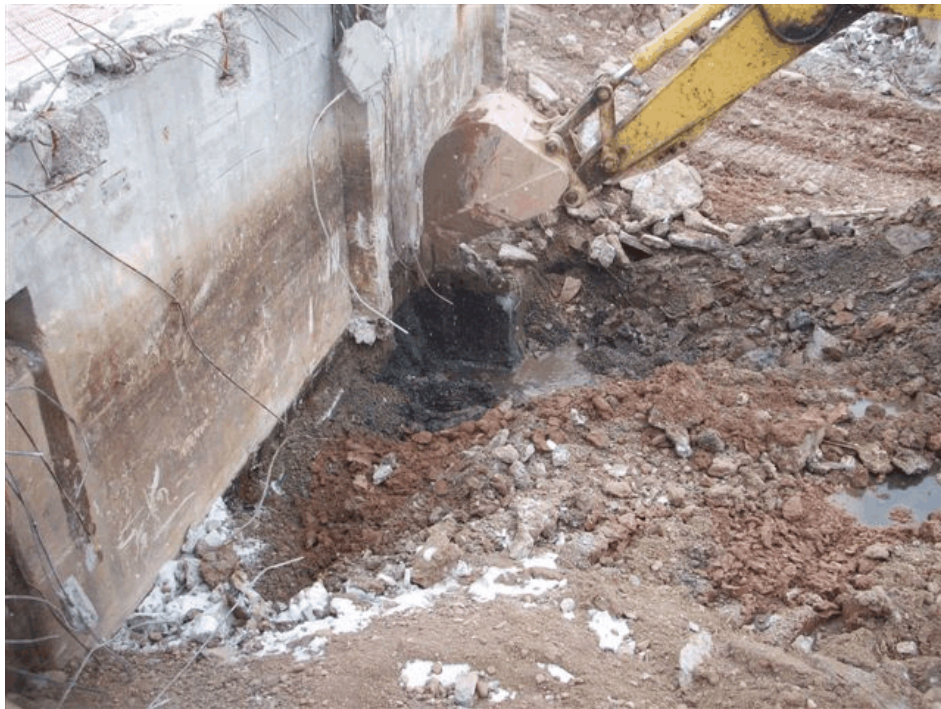
Figure 2-8. Photograph showing the excavation of the basement sump along the south foundation wall of the Spauldite Sheet Basement. View looking southwest. Photograph taken by Brian Hutzler on February 16, 2010.
