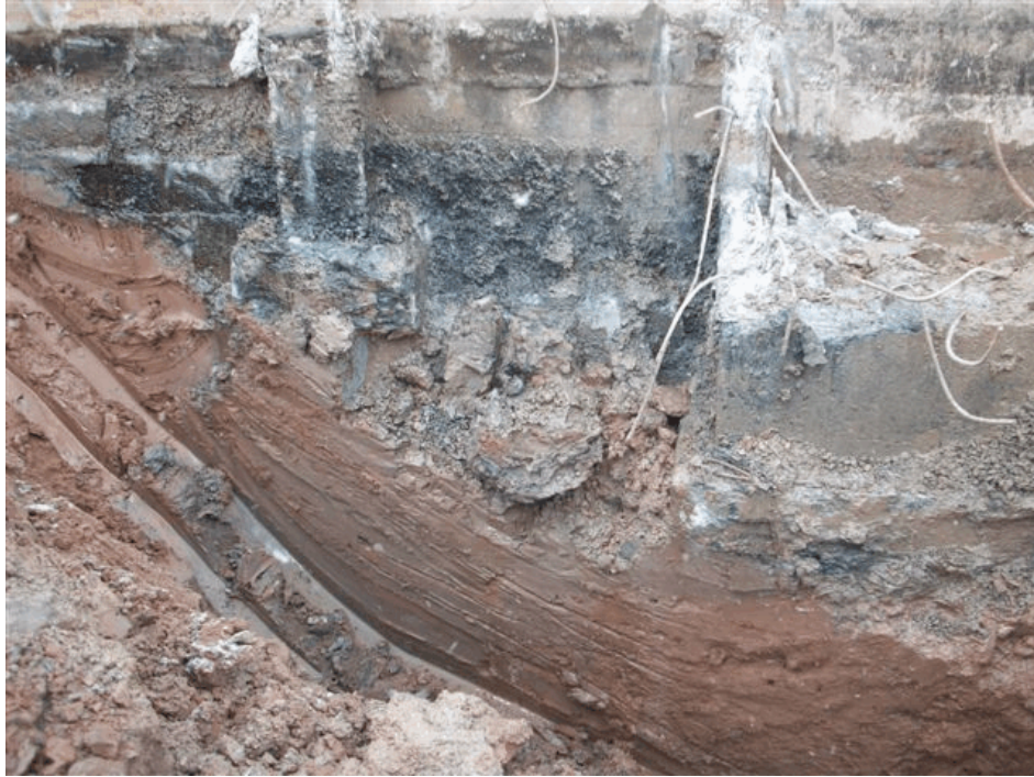
Figure 2-9. Photograph showing the native silty clay underlying the former basement sump along the south foundation wall of the Spauldite Sheet Basement. View looking southeast. Photograph taken by Brian Hutzler on February 16, 2010.
