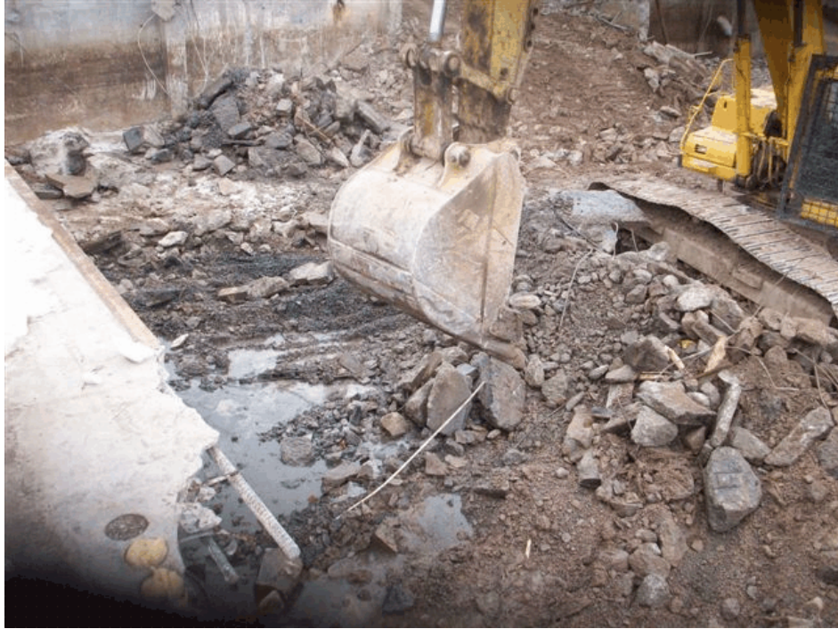
Figure 2-1. Photograph showing the removal of the concrete floor of the Spauldite Sheet Basement. View looking south. Photograph taken by Brian Hutzler on February 9, 2010.
