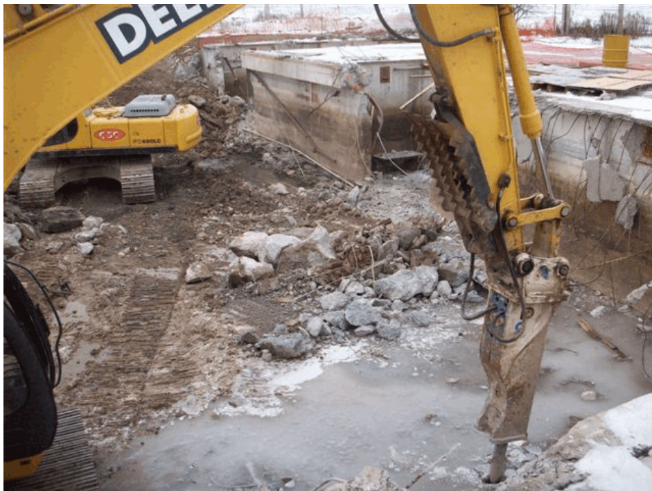
Figure 2-2. Photograph showing the removal of the concrete floor of the Spauldite Sheet Basement. View looking south. Photograph taken by Brian Hutzler on February 9, 2010.
