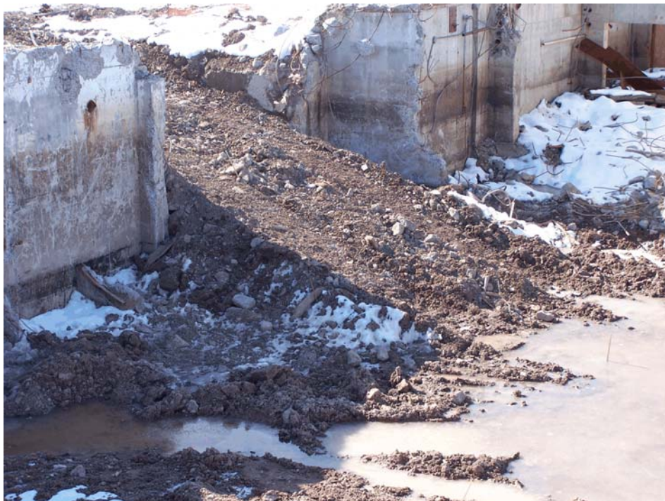
Figure 2-16. Photograph showing the ramp into the Spauldite Sheet Basement for excavator access. This ramp was left in place following remedial activities. View looking southwest. Photograph taken by Glenn May on March 4, 2010.
