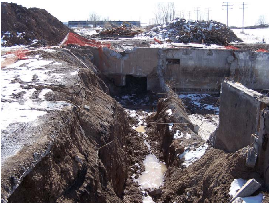
Figure 2-4. Photograph showing the portion of the east foundation wall that was removed during the Spauldite Sheet Basement and K-Line Storm Sewer remediation. View looking southwest. Photograph taken by Glenn May on March 4, 2010.
