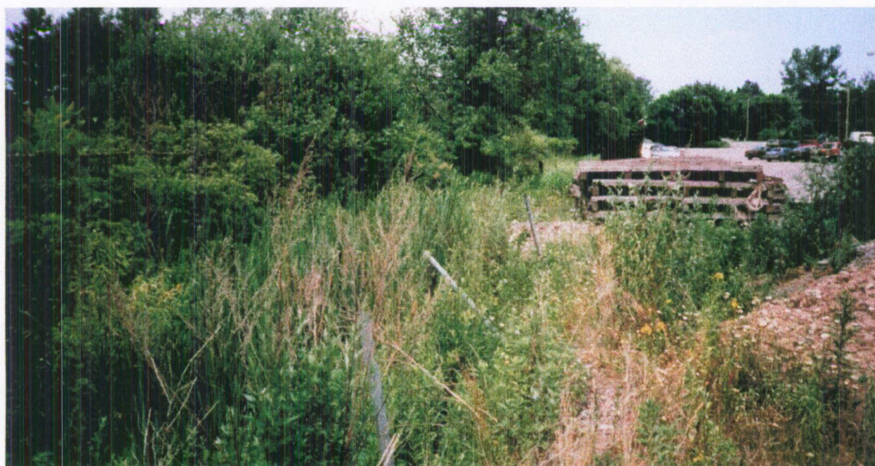
Sedimentation basin over grown with vegetation.
