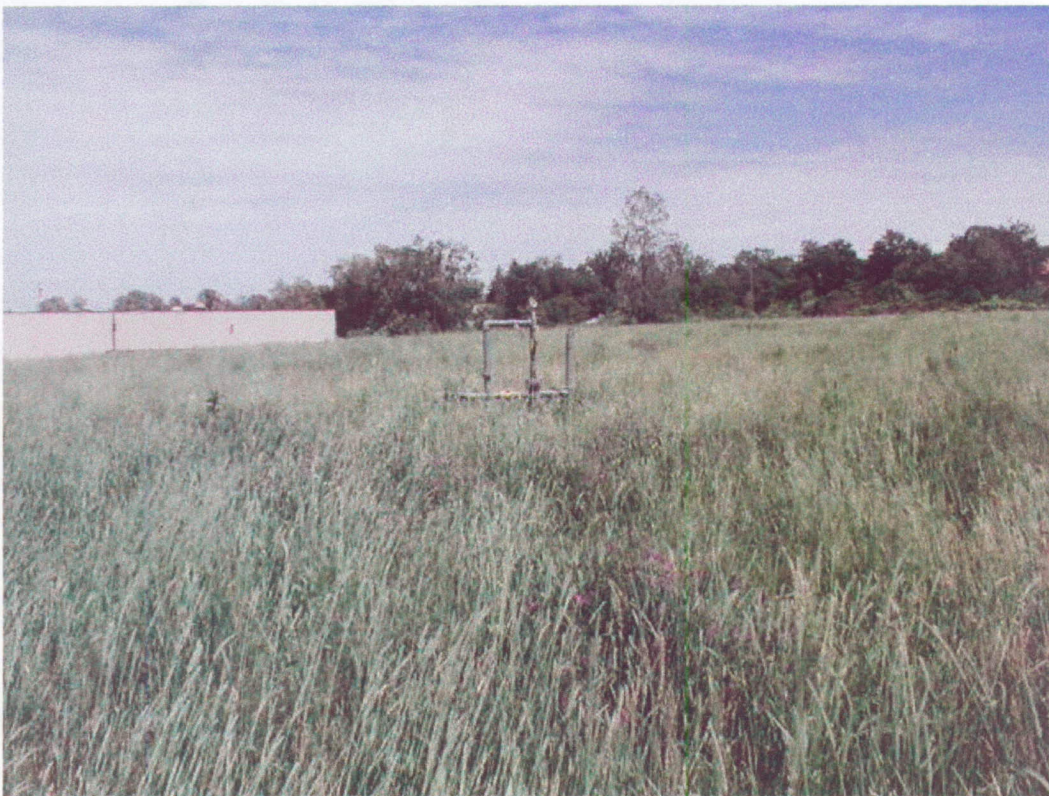
View looking north at landfill cap; gas well in center of photograph.
