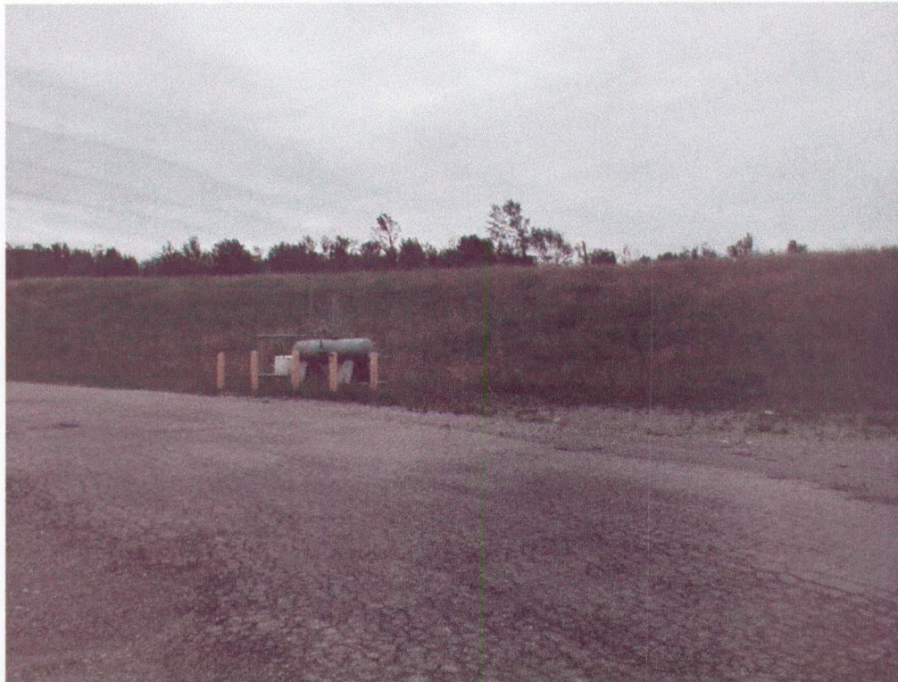
View looking south at northern edge of IRM closure area.
