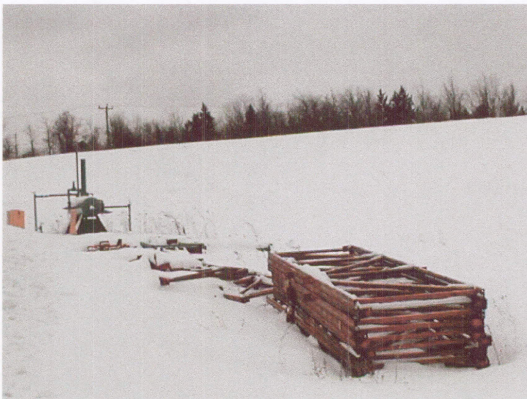
View of gas well along north face of IRM, facing southeast
