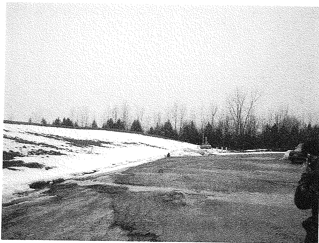
View of the northern end of the closure cover, looking west.
