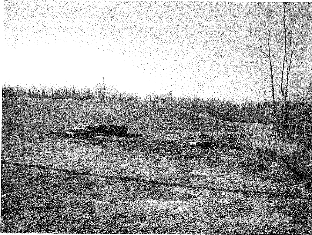
View of northwest end of closure cover, looking southeast.
