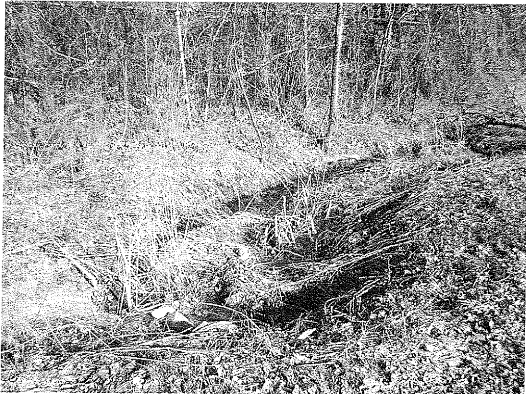
View of drainage swale on western side of parking lot, looking north.
