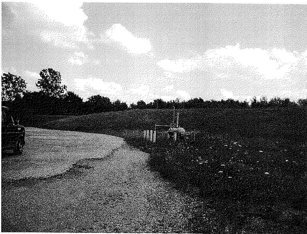
View of the north end of the closure cover looking east.
