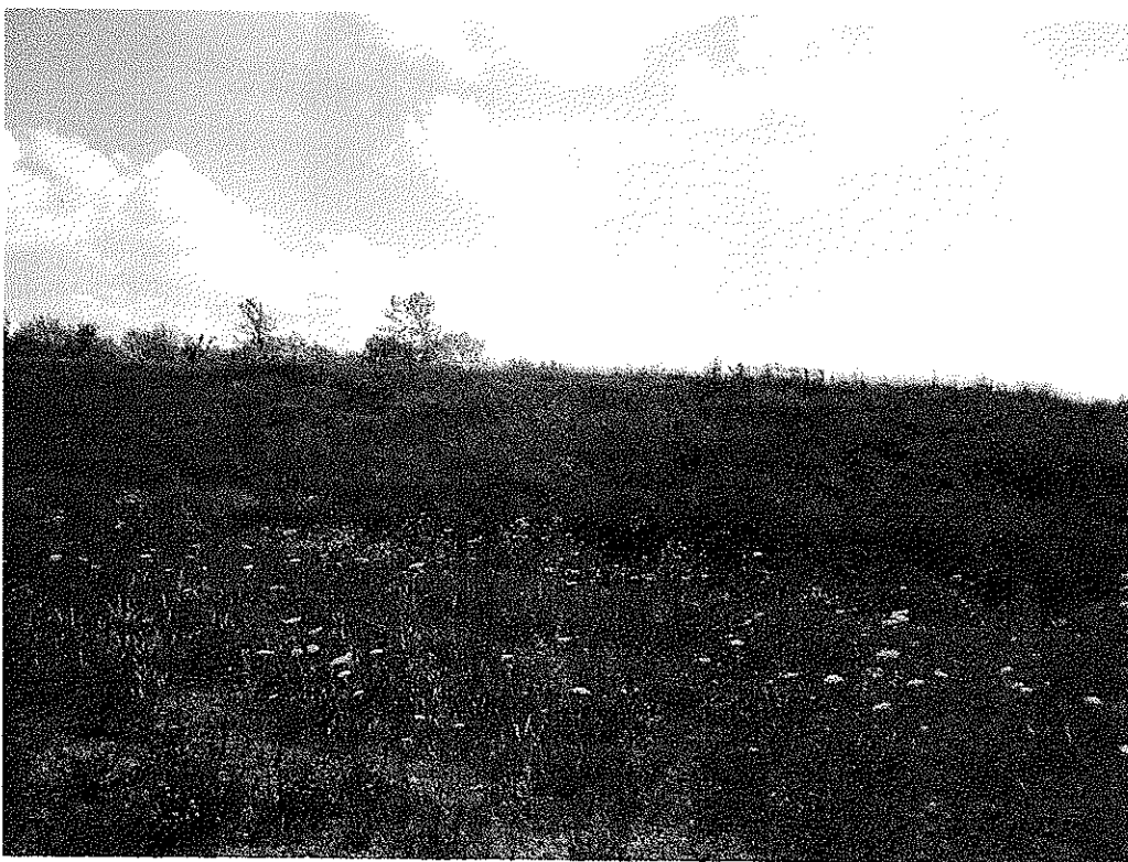
View of the closure cover looking south.
