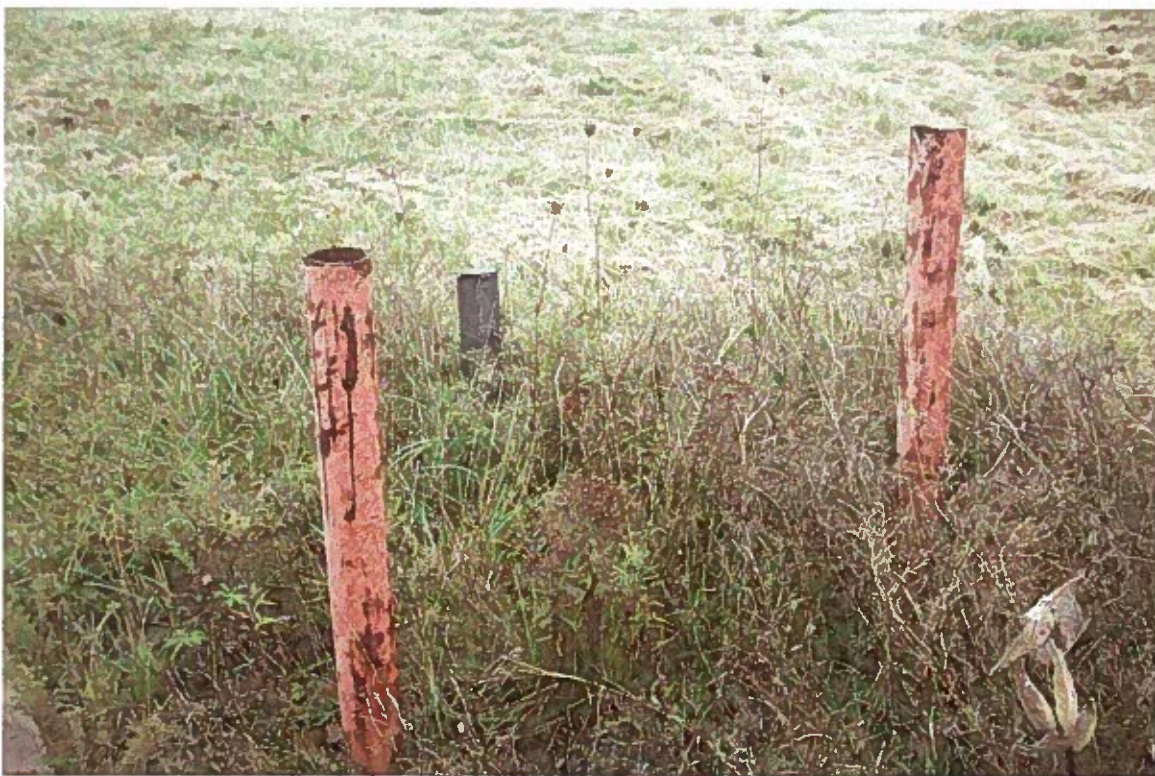
View of a typical monitoring well.
