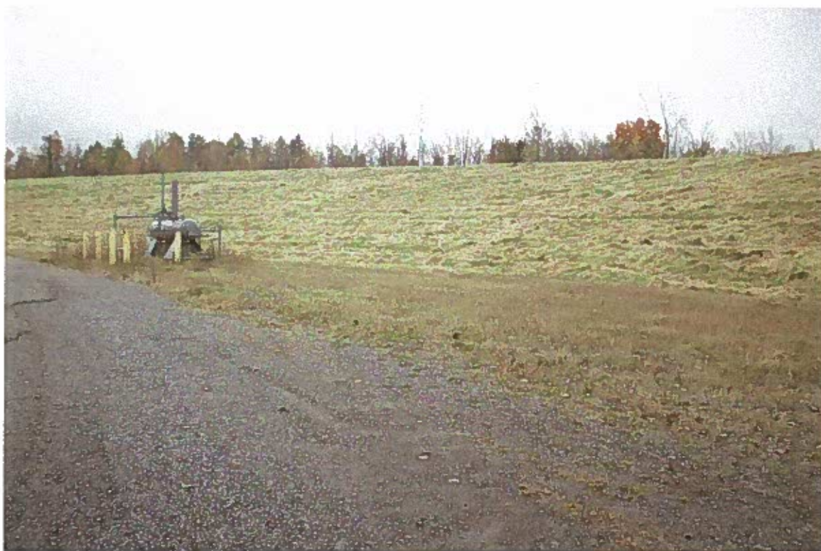
View of cover and gas well.
