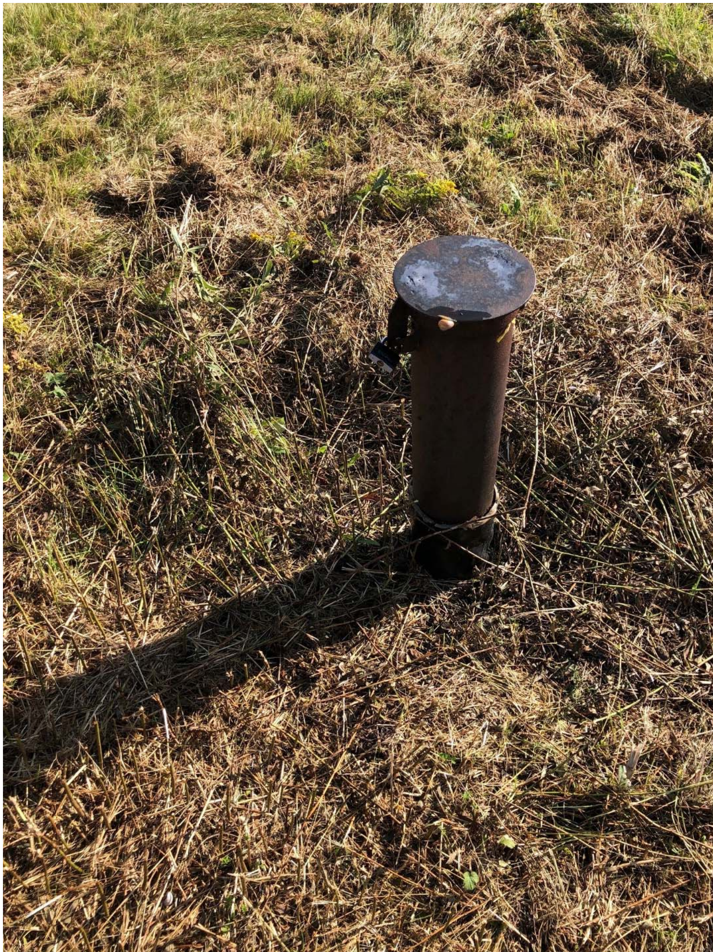
View of the monitoring well GW-5 protective steel casing and cover prior to decommissioning.
