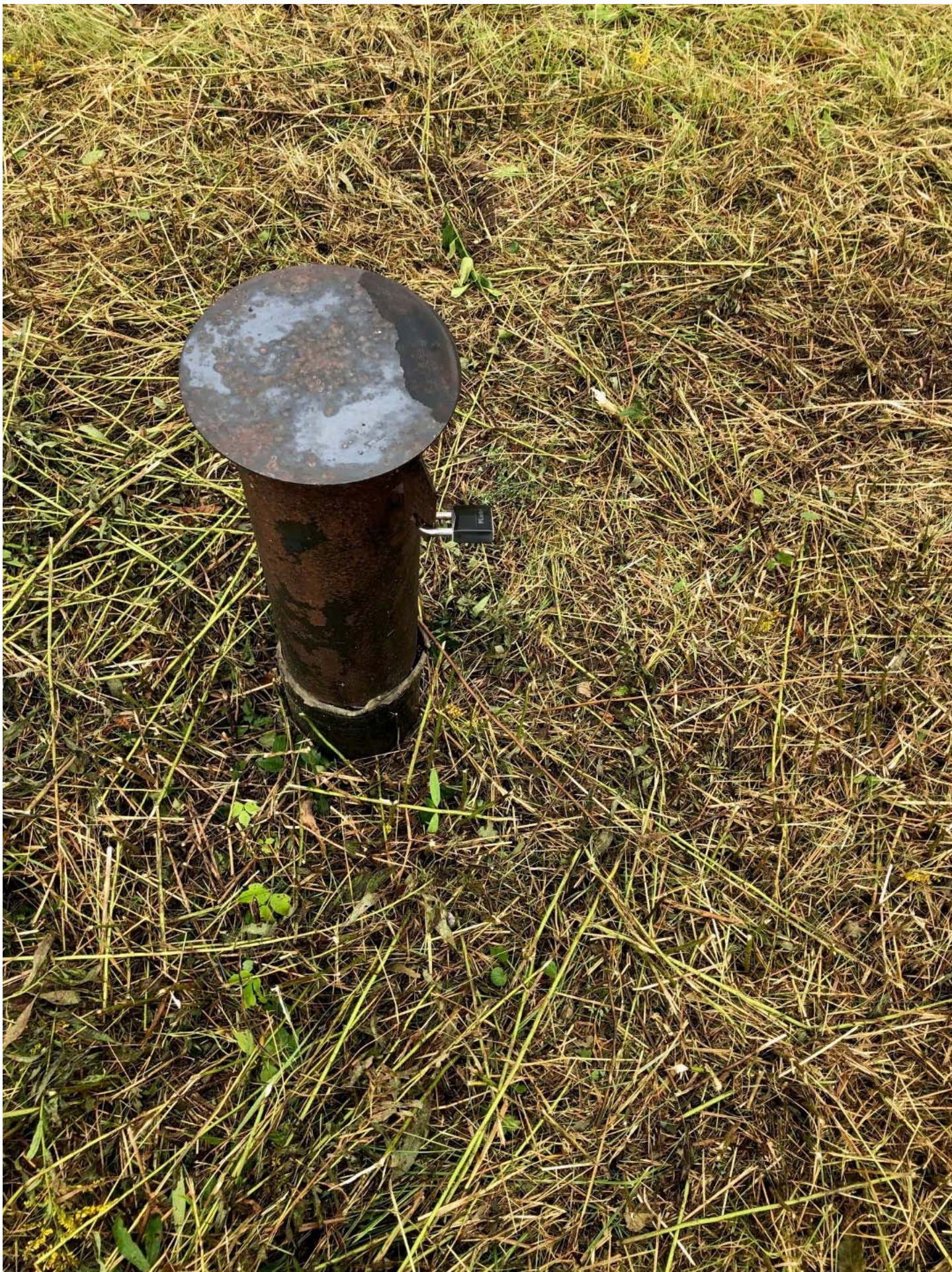
View of the monitoring well GW-2 protective steel casing and cover prior to decommissioning.
