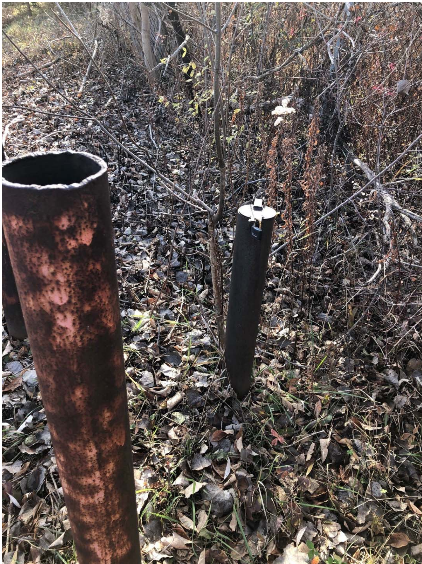
View of the stick-up, steel, protective casing and cover for groundwater monitoring well GW-3, and protective bollards, facing southwest.
