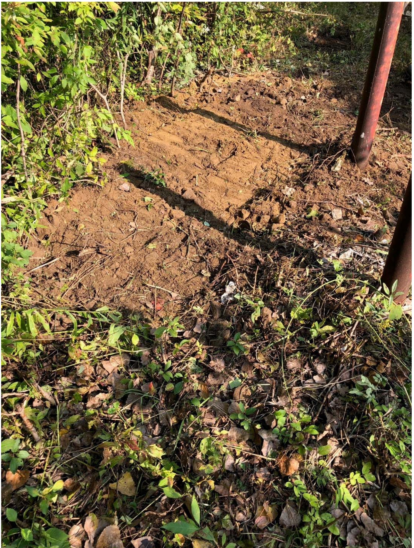
View of the restored ground surface following the removal of monitoring well GW-3 protective steel casing and associated well materials, facing northwest. (Note: the protective bollards were left in place.)
