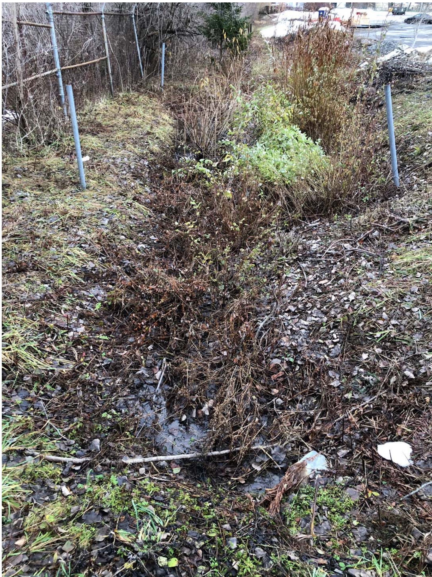
View of the drainage way (partially blocked by vegetation) located to the northwest of the landfill area facing northwest.
