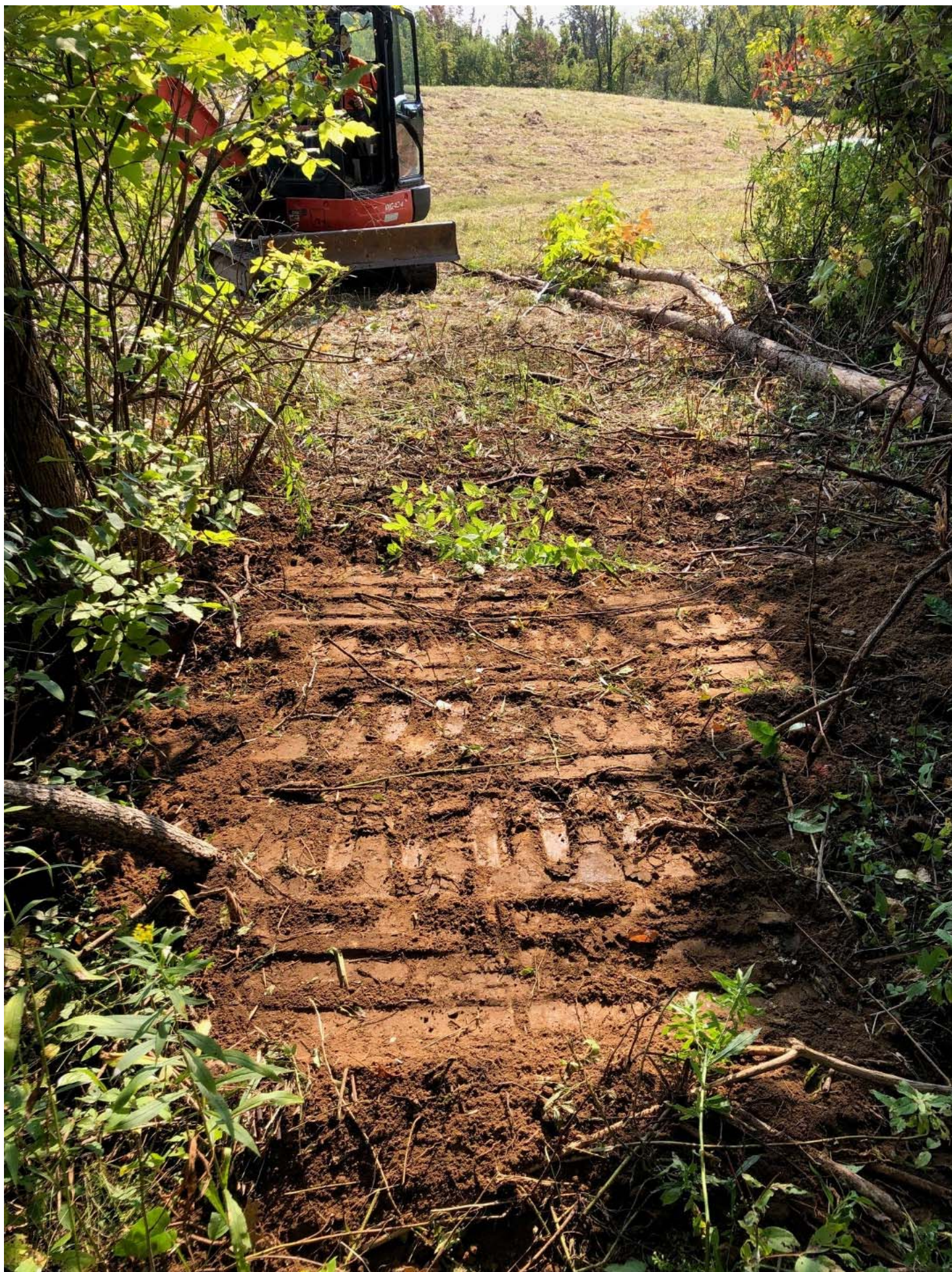
View of the restored ground surface following the removal of monitoring well GW-1 protective steel casing and associated well materials, facing east.
