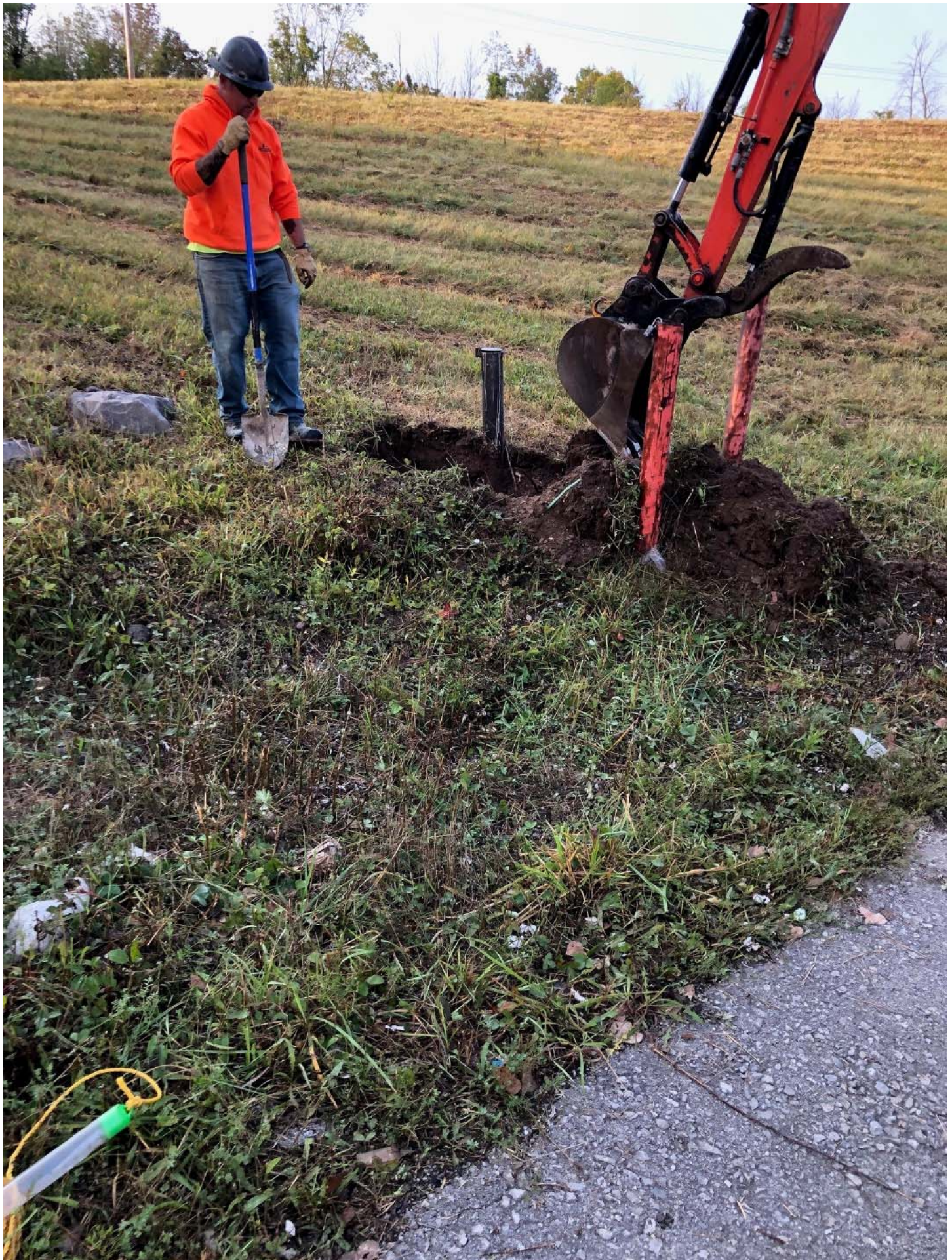
Representative view of the removal of a protective steel casing and well casing, using a mini-excavator, to a depth of approximately five feet below the ground surface.
