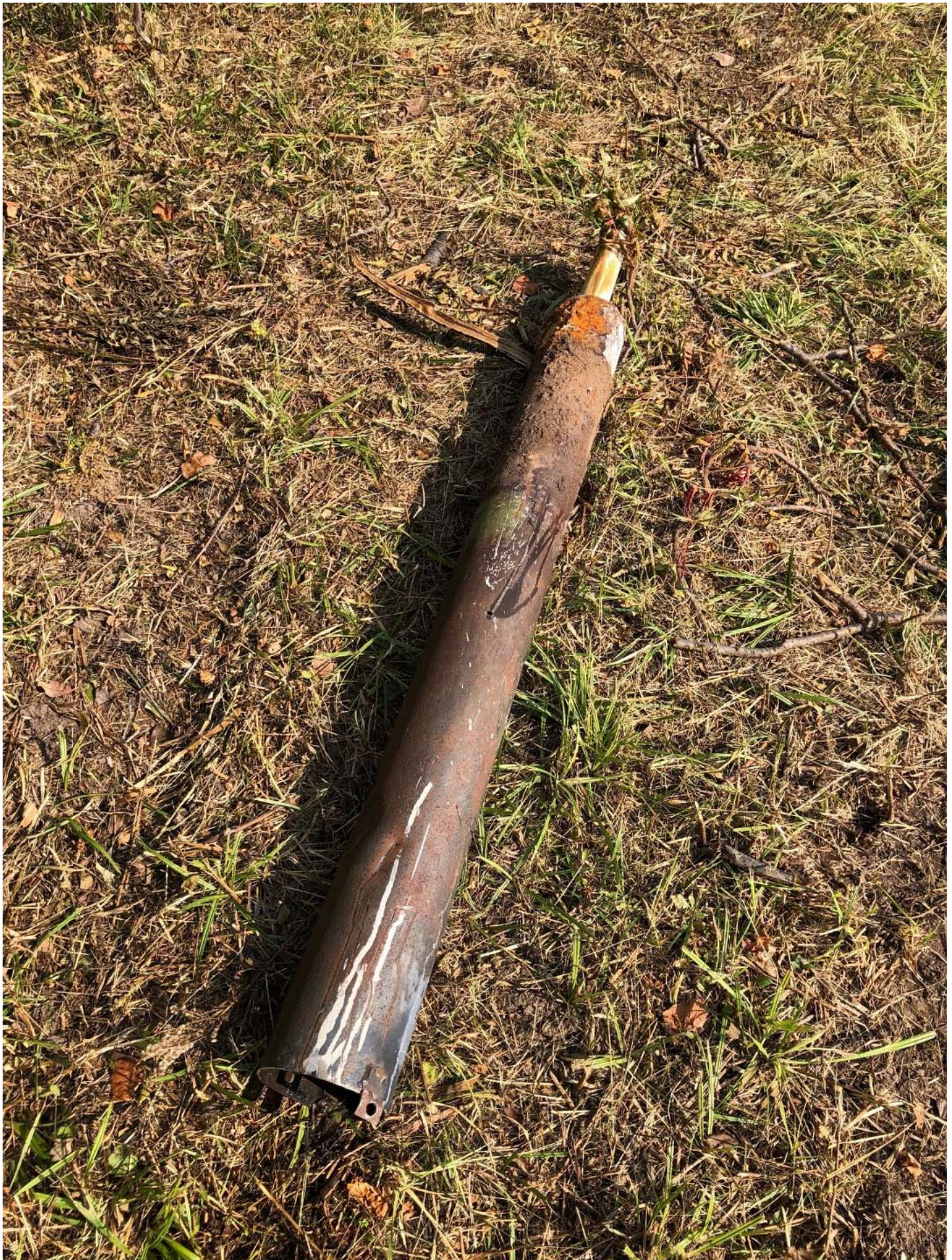
View of the monitoring well GW-1 protective steel casing and associated well materials that were removed from the ground following monitoring well decommissioning.
