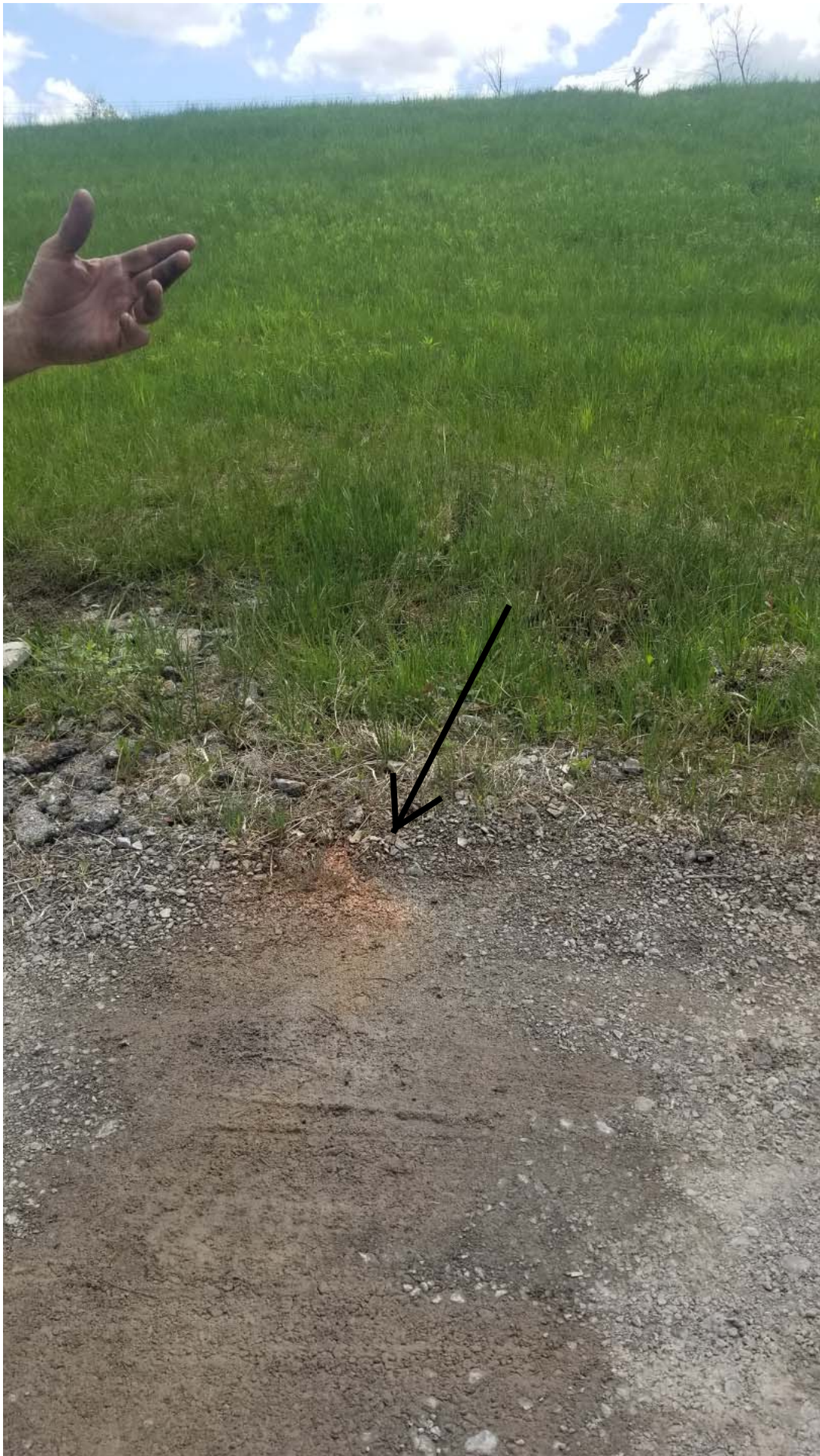
View of the mild, iron-stained seepage observed on the north side of the landfill, facing south
