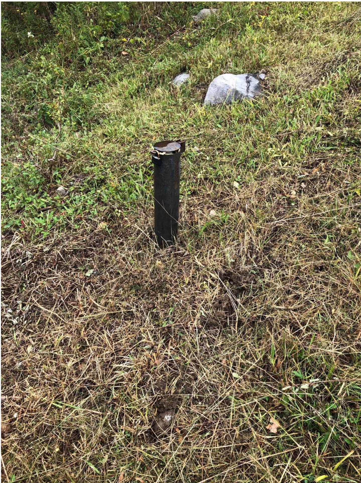
View of the monitoring well GW-4 protective steel casing prior to decommissioning, facing east.
