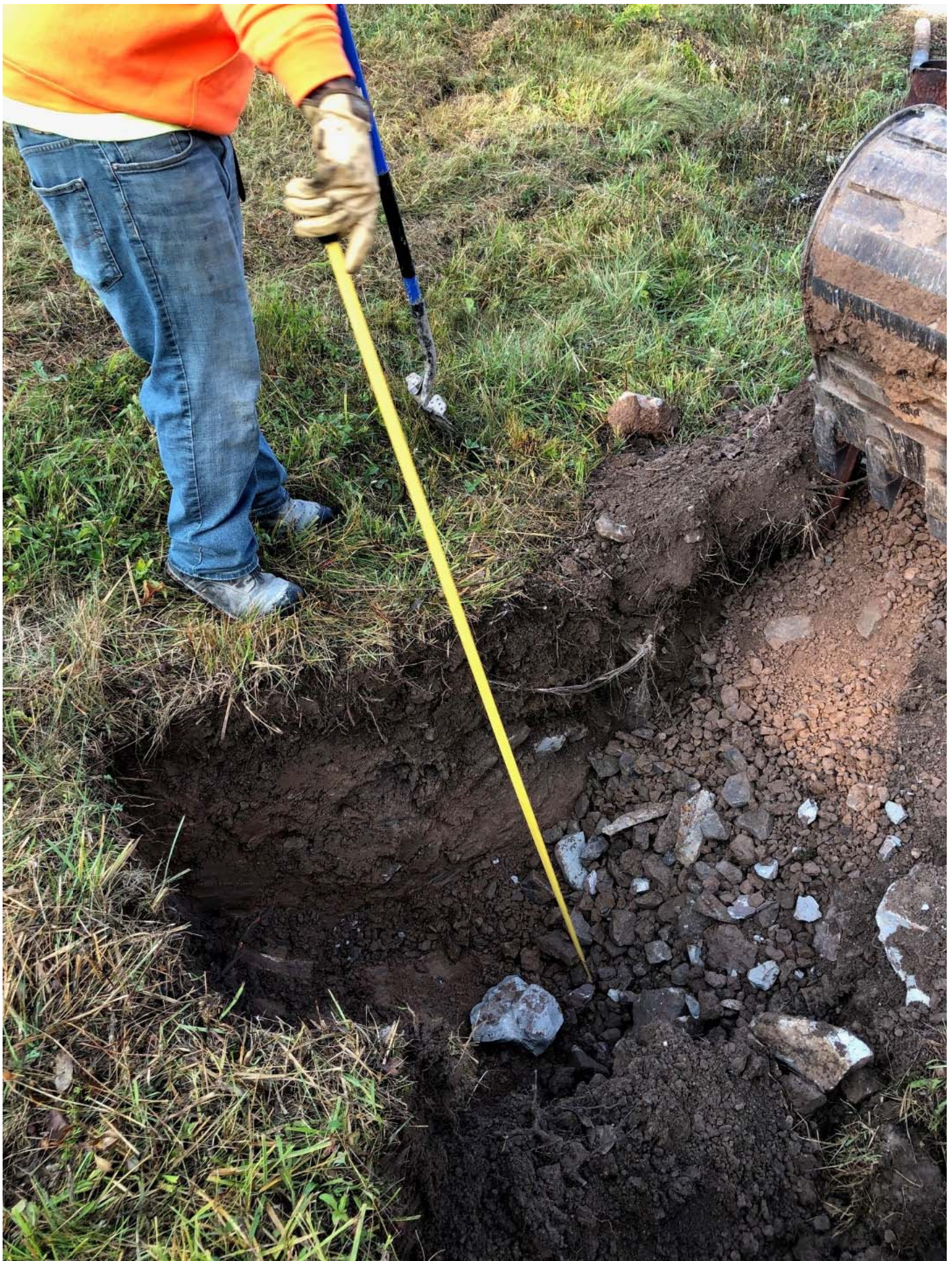
View of the drilling contractor addressing the depth of the excavation during the work to excavate/remove the monitoring well GW-4 protective steel casing and well casing.
