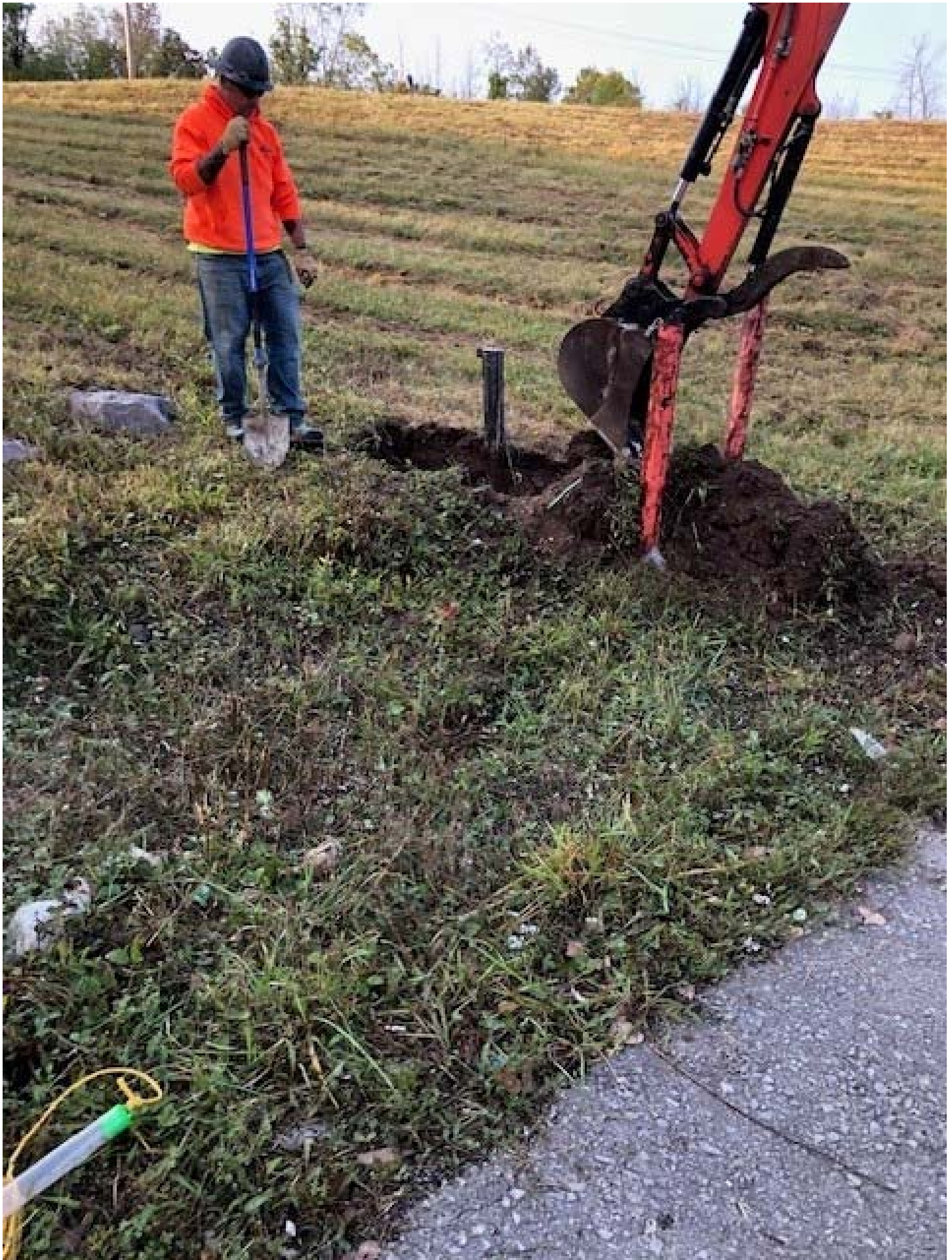
Representative view of monitoring well decommissioning work, completed in conjunction with the semi-annual landfill inspection.
