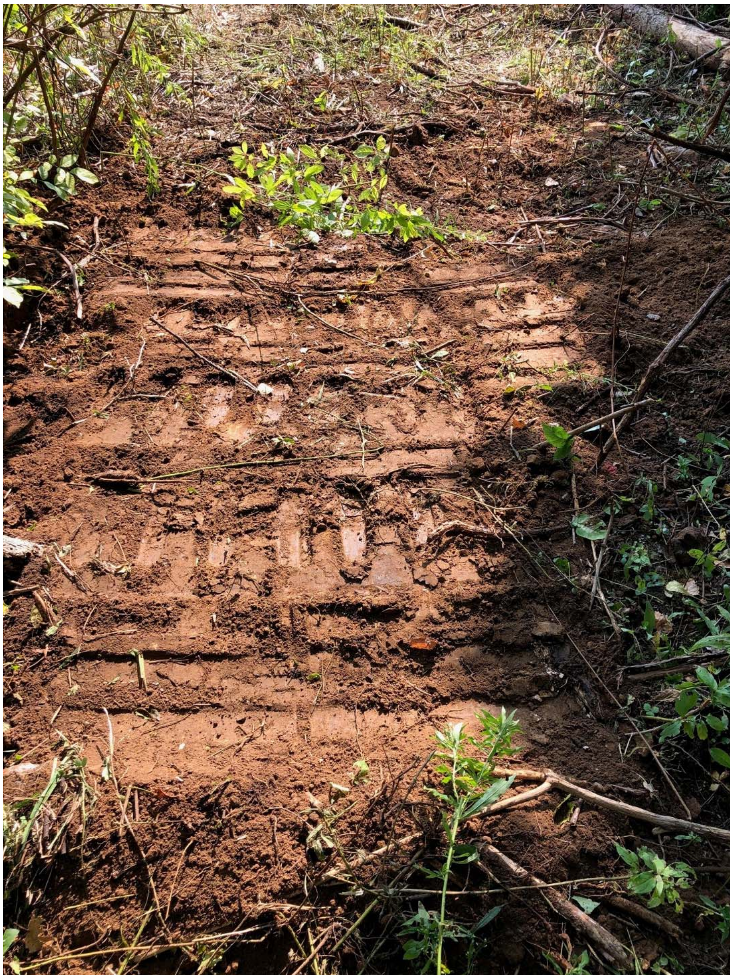
Close-up view of the restored ground surface following the removal of monitoring well GW-1 protective steel casing and associated well materials, facing east.
