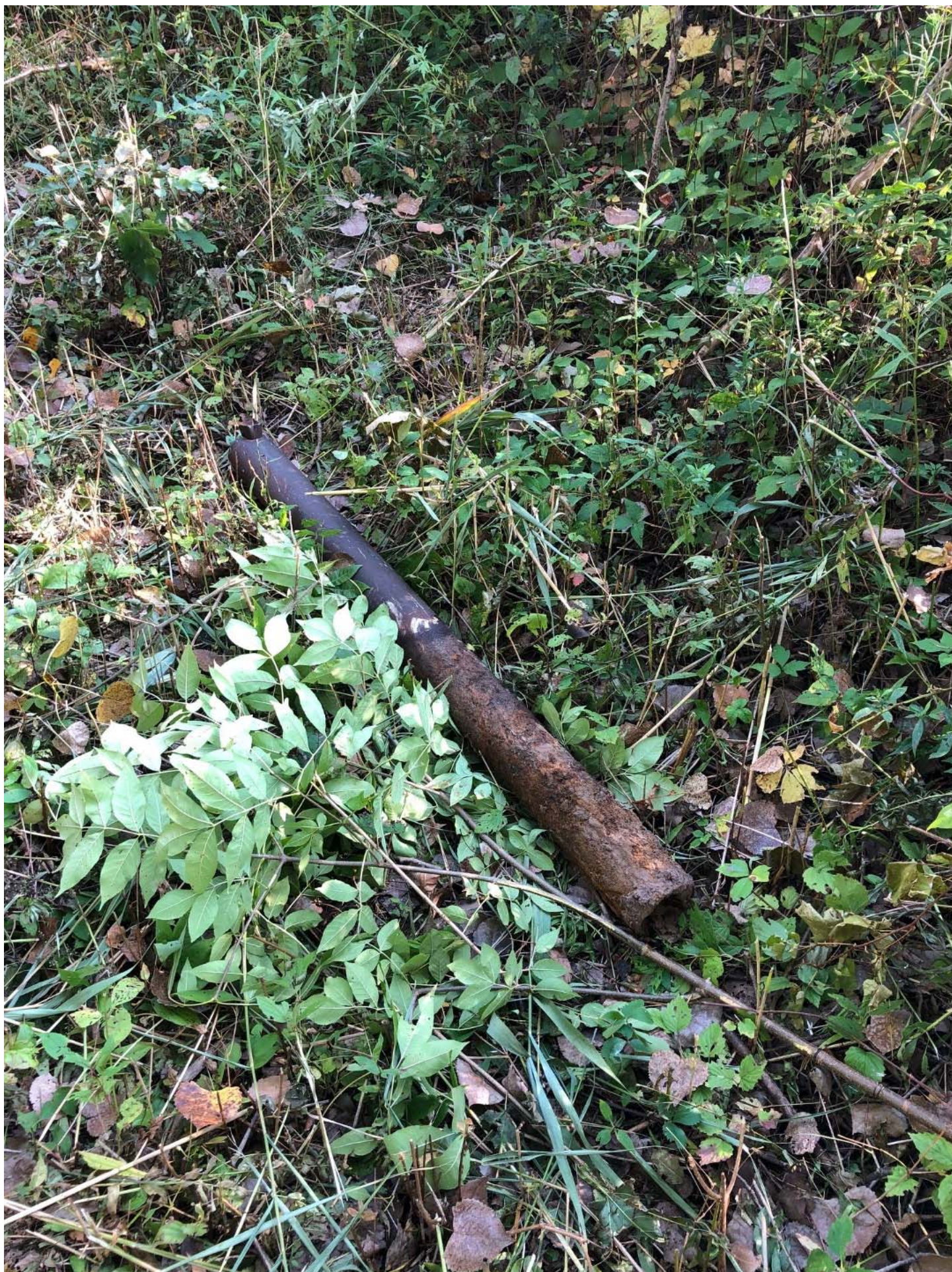
View of the monitoring well GW-3 protective steel casing that was removed from the ground following monitoring well decommissioning.
