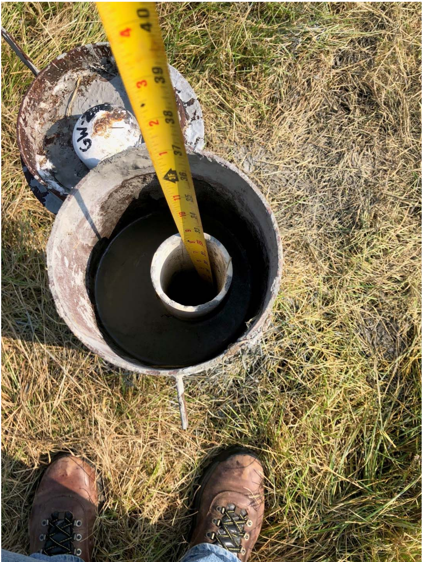
View showing the depth (below the top of PVC casing) to the top of the grout, tremmied into monitoring well GW-2, following monitoring well decommissioning activities.
