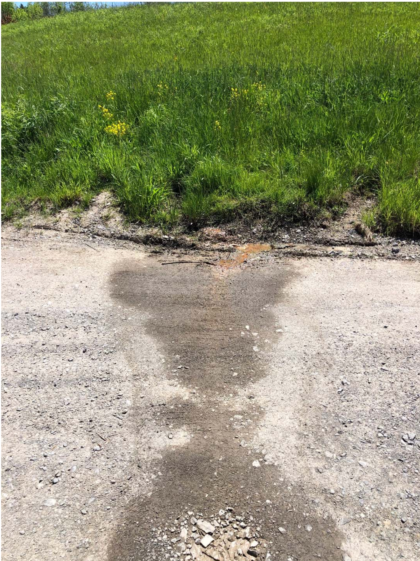
View of second area of water seepage observed exiting the toe of the northeastern slope of the landfill, facing southeast.
