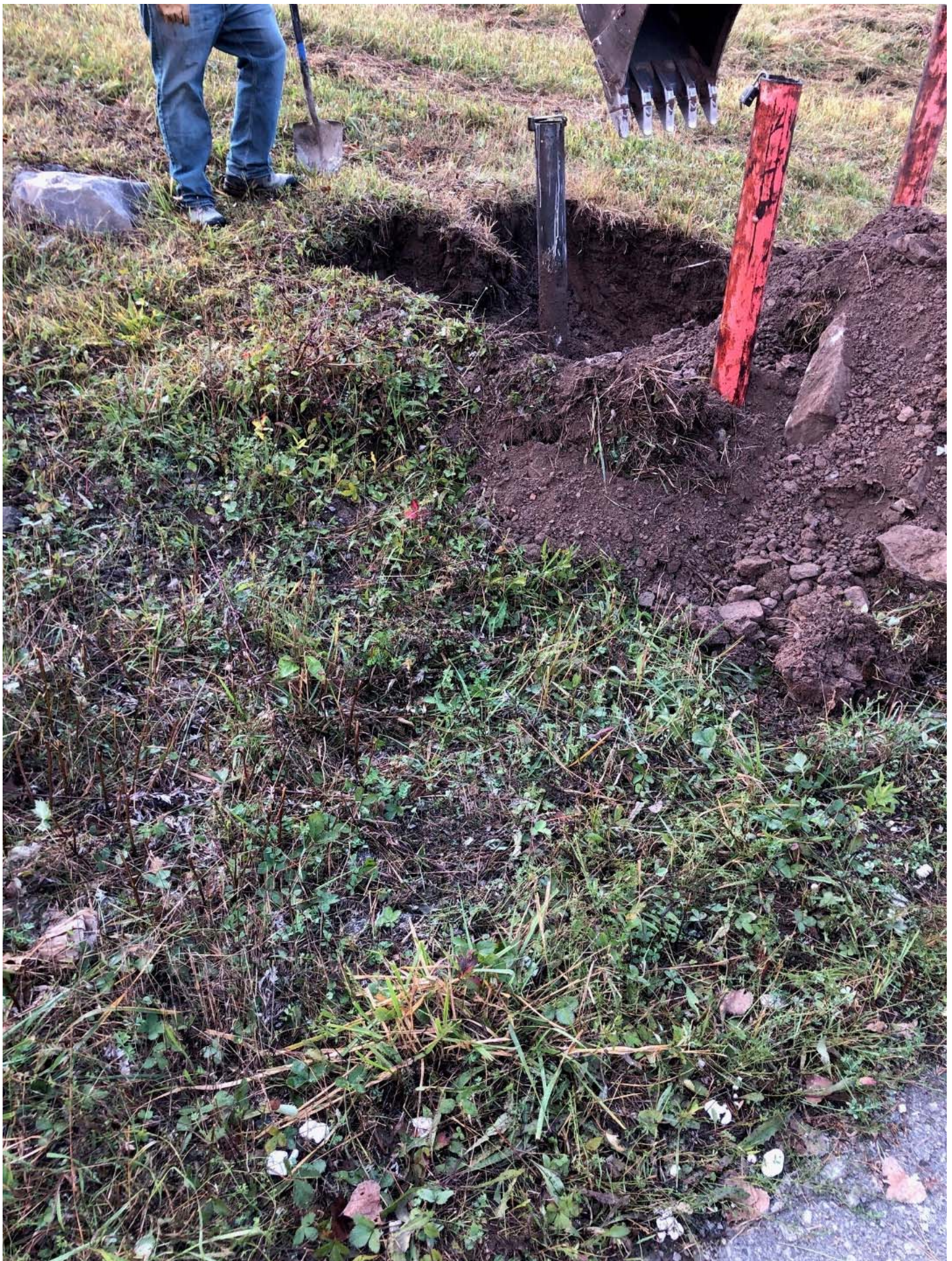
View of the mini-excavator during the work to excavate/remove the monitoring well GW-4 protective steel casing and well casing to a depth of approximately five feet below the ground surface.
