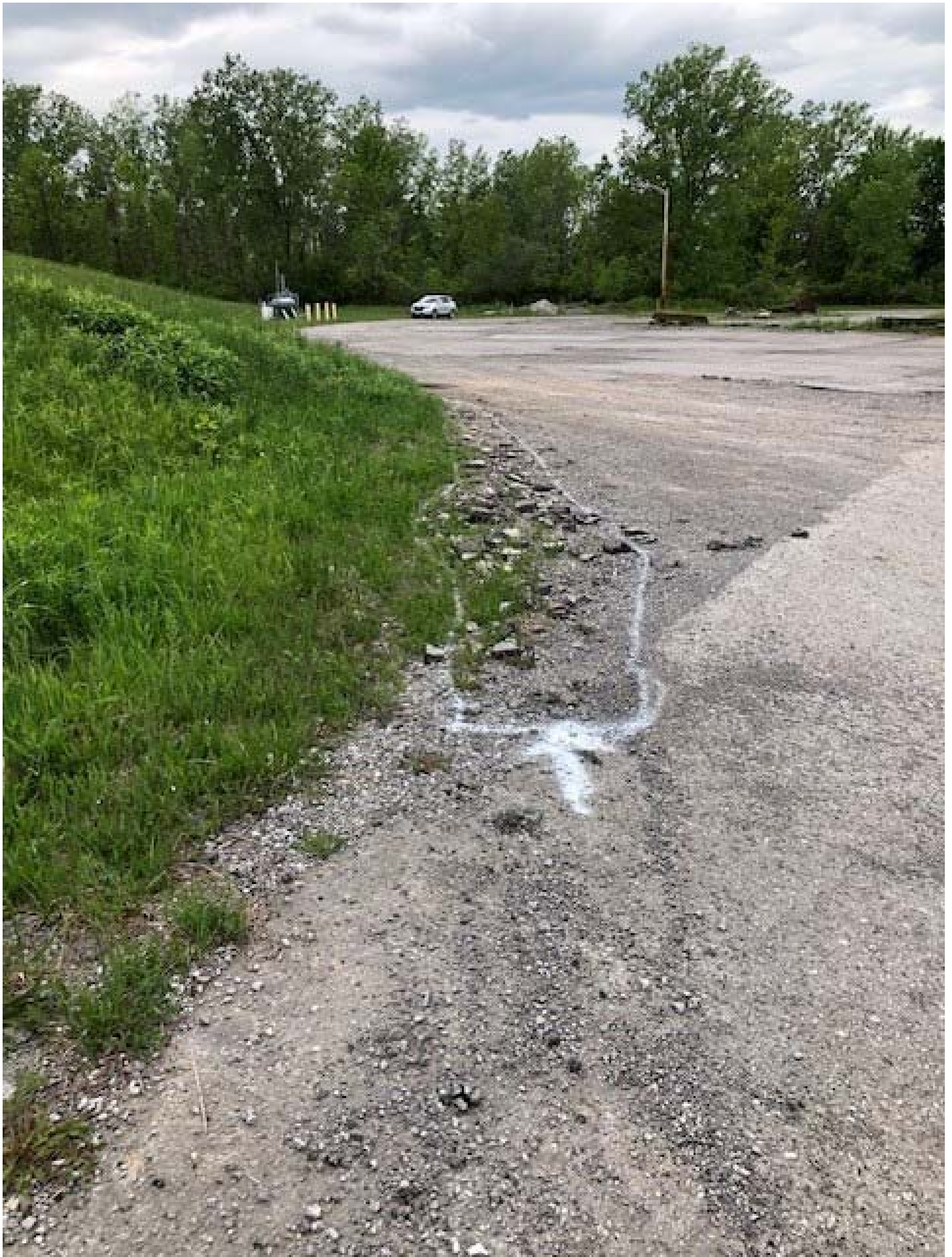
View of marking paint delineating an area of asphalt to be repaired at toe of the northern slope of the landfill area (center), and the repaired slough area adjacent (left) on the landfill slope, facing west.
