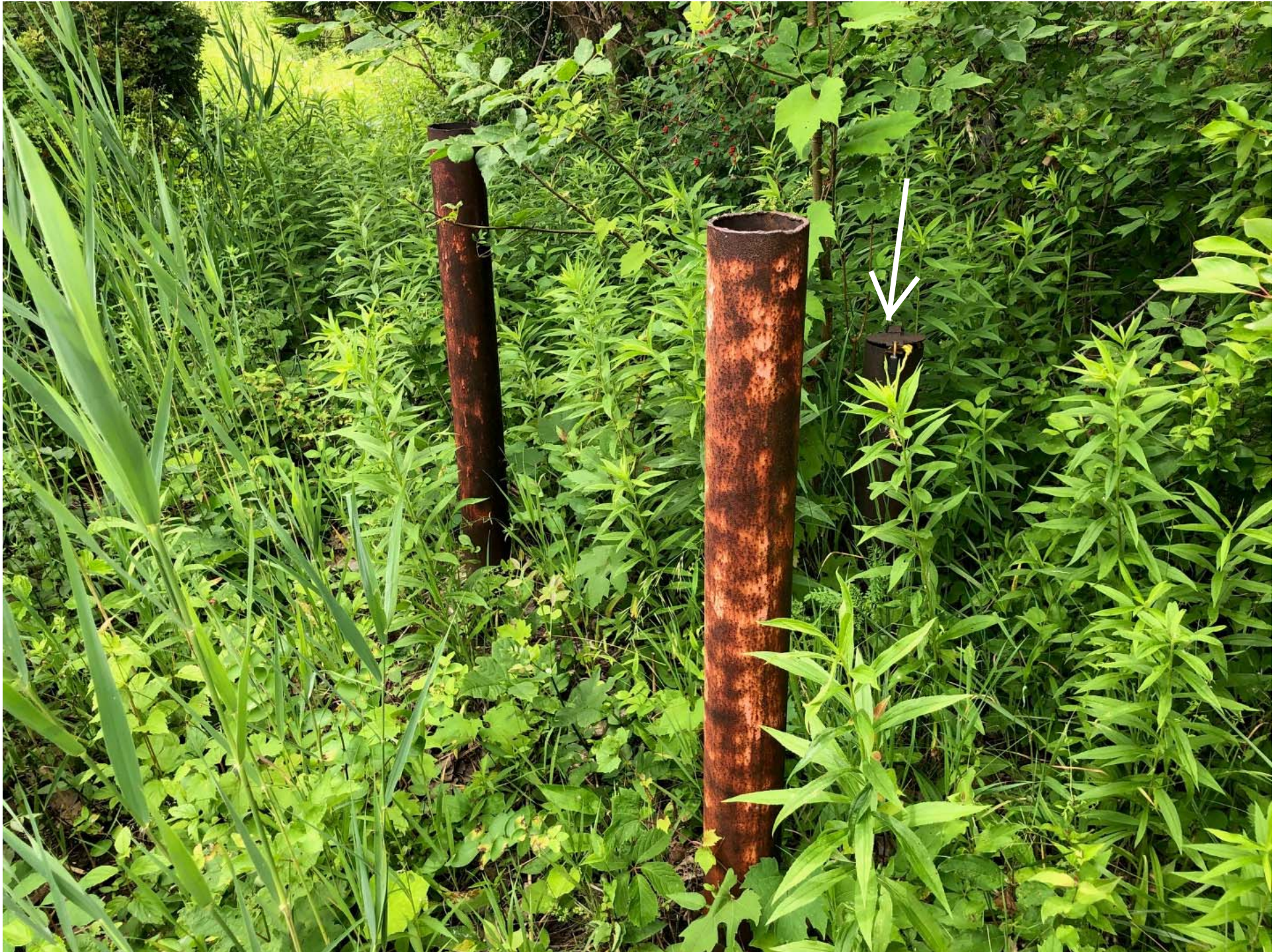
View of the stick-up, steel, protective casing and cover for groundwater monitoring well GW-3 (arrow), and protective bollards, facing southwest.
