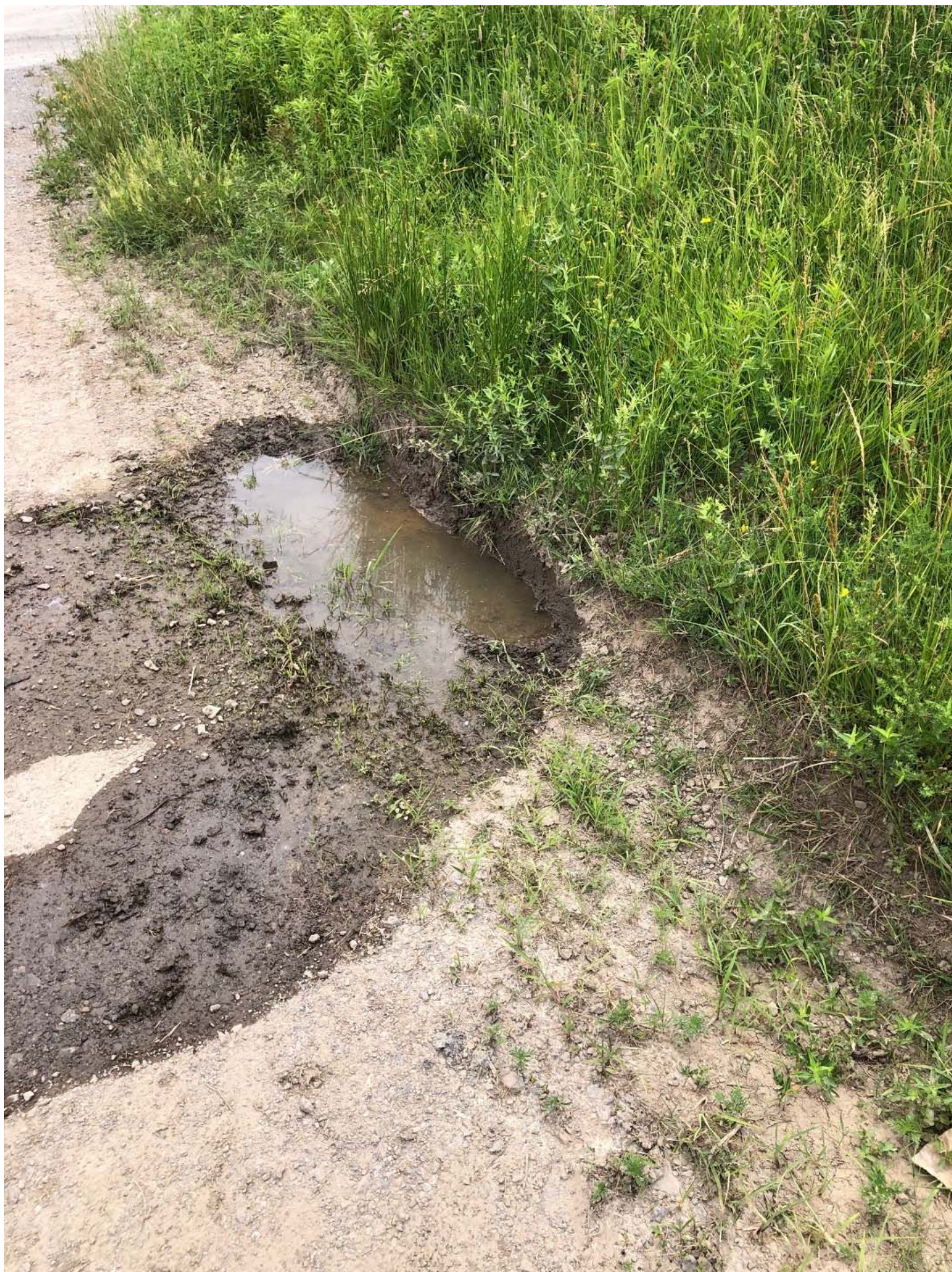
View of standing water, present at the base of the northeastern slope in an area where rutting from truck traffic is evident, facing southeast.
