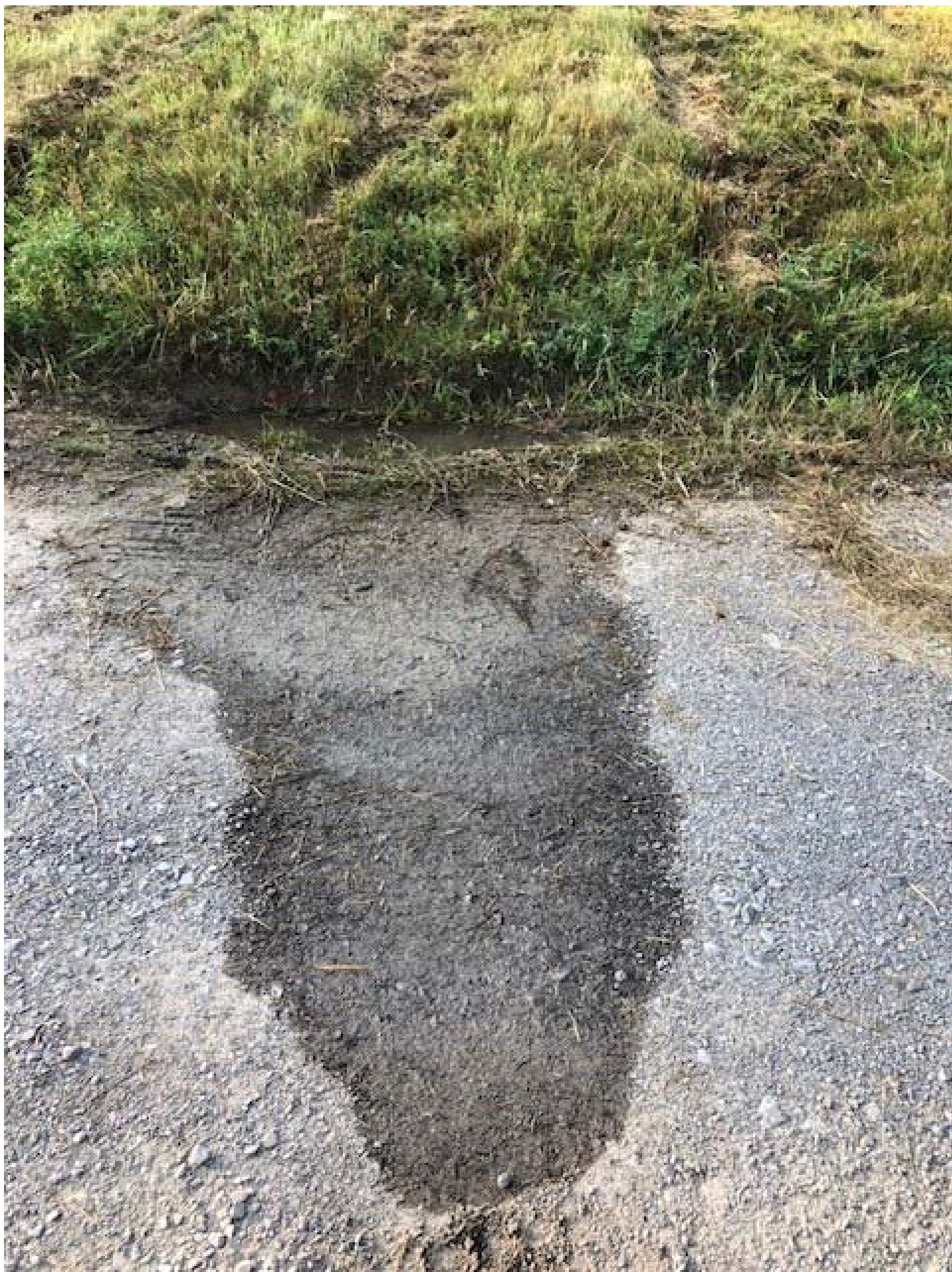
View of standing water present at the base of the northeastern slope of the landfill, facing south.
