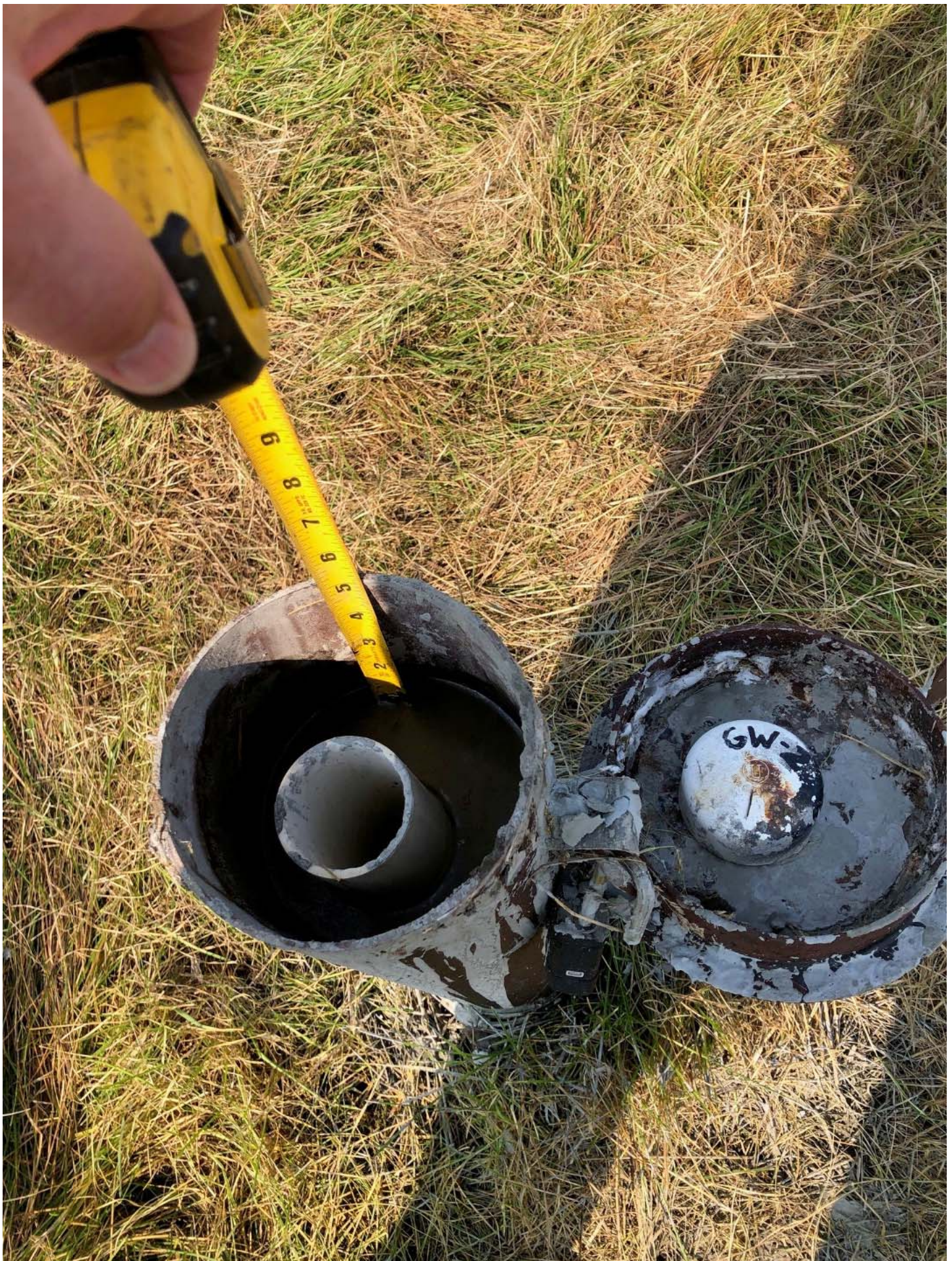
View showing the depth (below top of steel casing) of the grout placed between the monitoring well casing and protective steel casing for monitoring well GW-2, following decommissioning activities.
