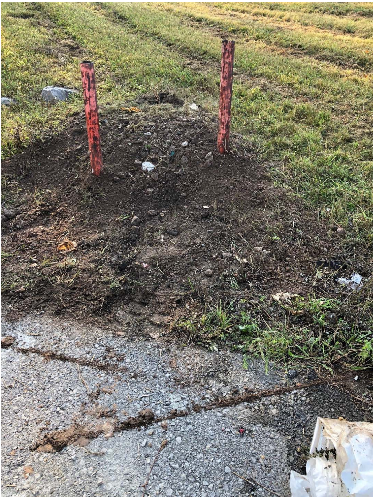
View of the restored ground surface following the removal of monitoring well GW-4 protective steel casing and associated well materials, facing south. (Note: the protective bollards were left in place.)
