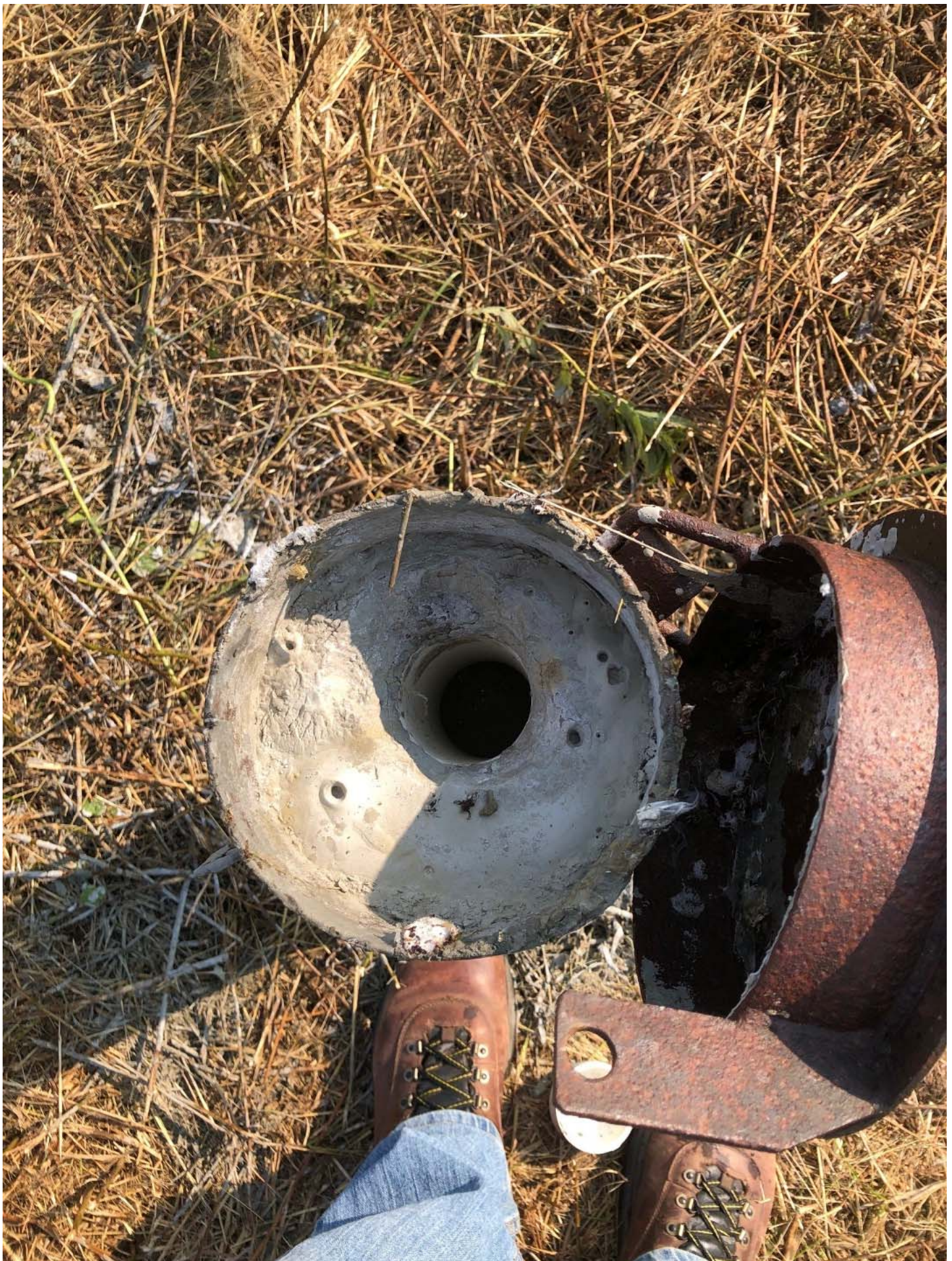
View showing the top of the grout, tremmied into monitoring well GW-5, and between the well casing and protective steel casing, following monitoring well decommissioning activities.
