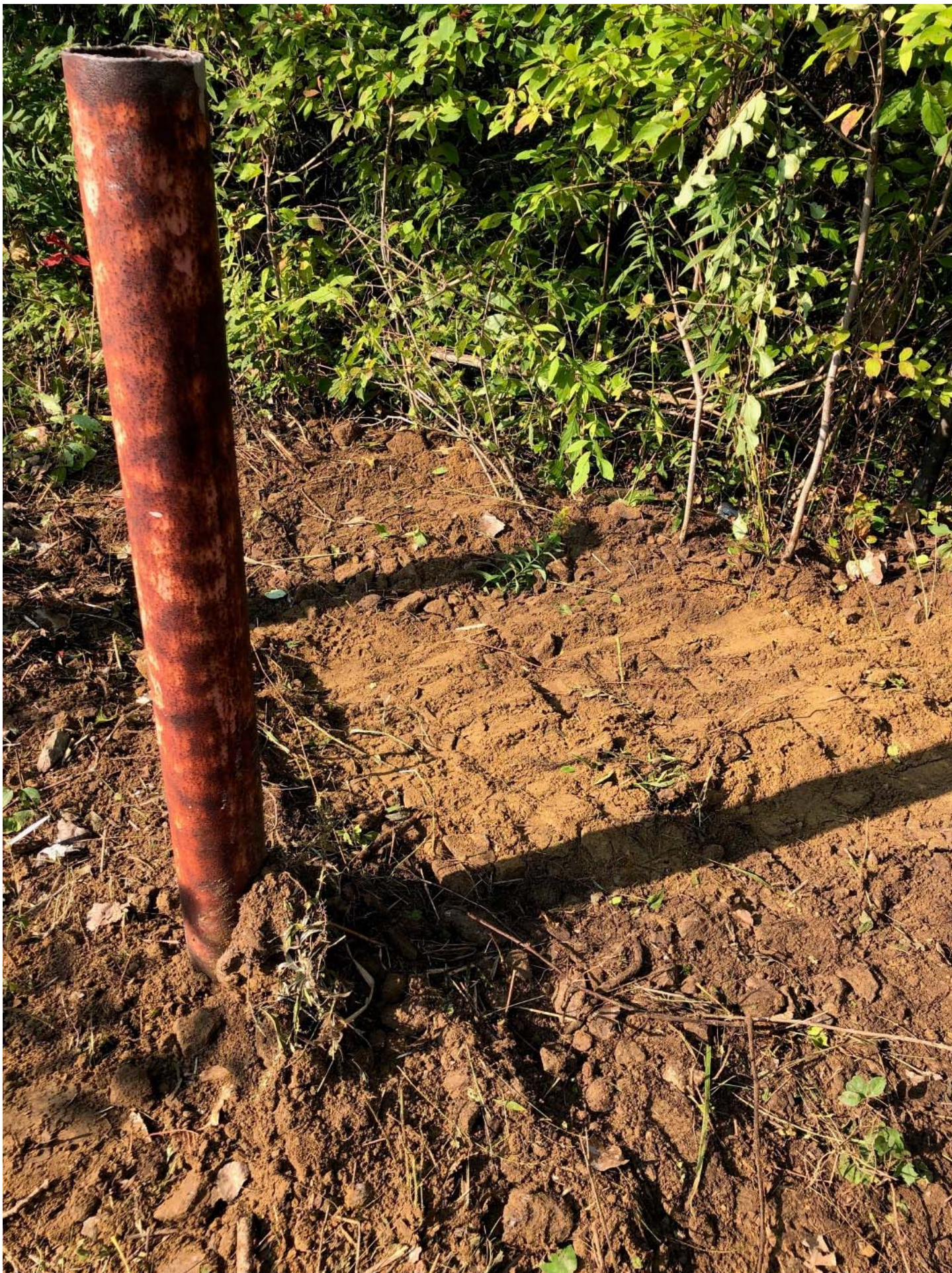
View of the restored ground surface following the removal of monitoring well GW-3 protective steel casing and associated well materials, facing southwest. (Note: the protective bollards were left in place.)
