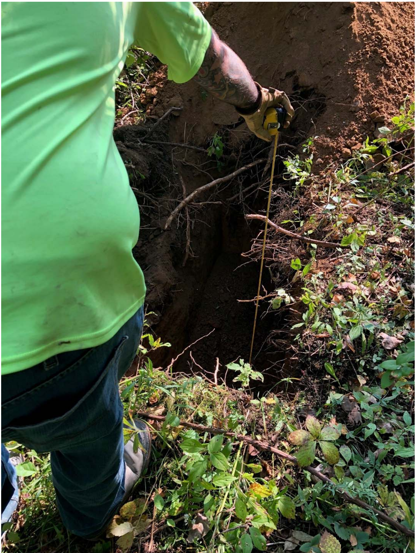
View of the excavation made to remove the monitoring well GW-1 protective steel casing and associated well materials from the ground.
