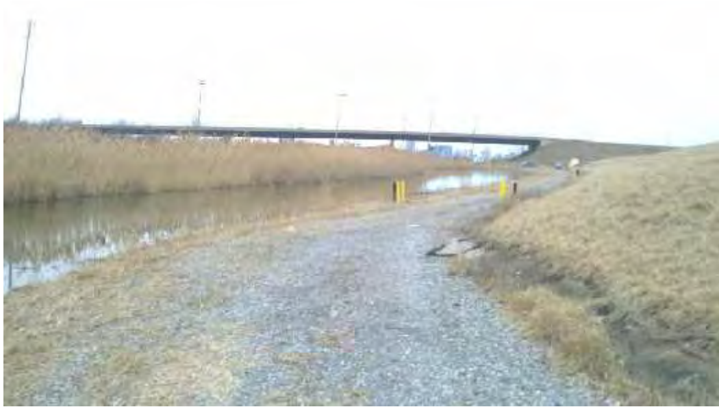
View along access road facing North
