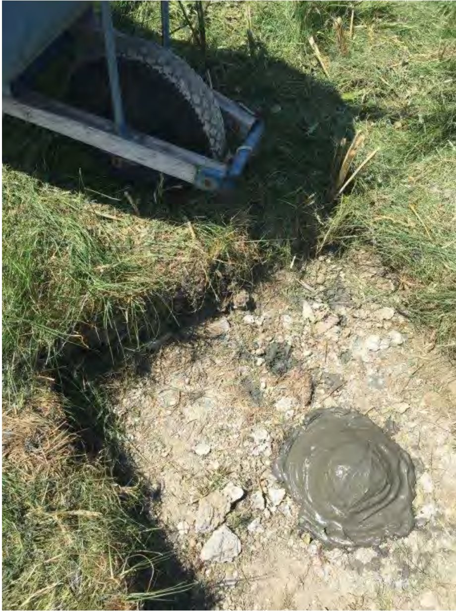
PZ-16 : PZ filled and abandoned
