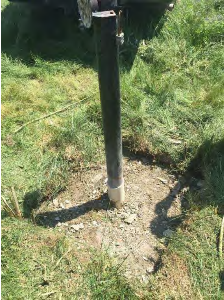
PZ-16 : Concrete pad removed
