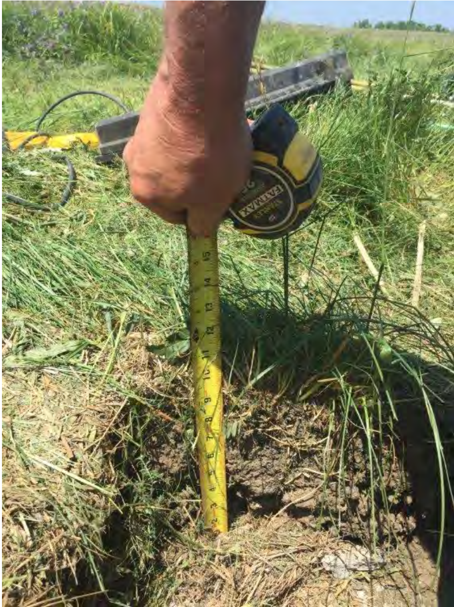
PZ-16 : removal of concrete pad and well to 12" below grade
