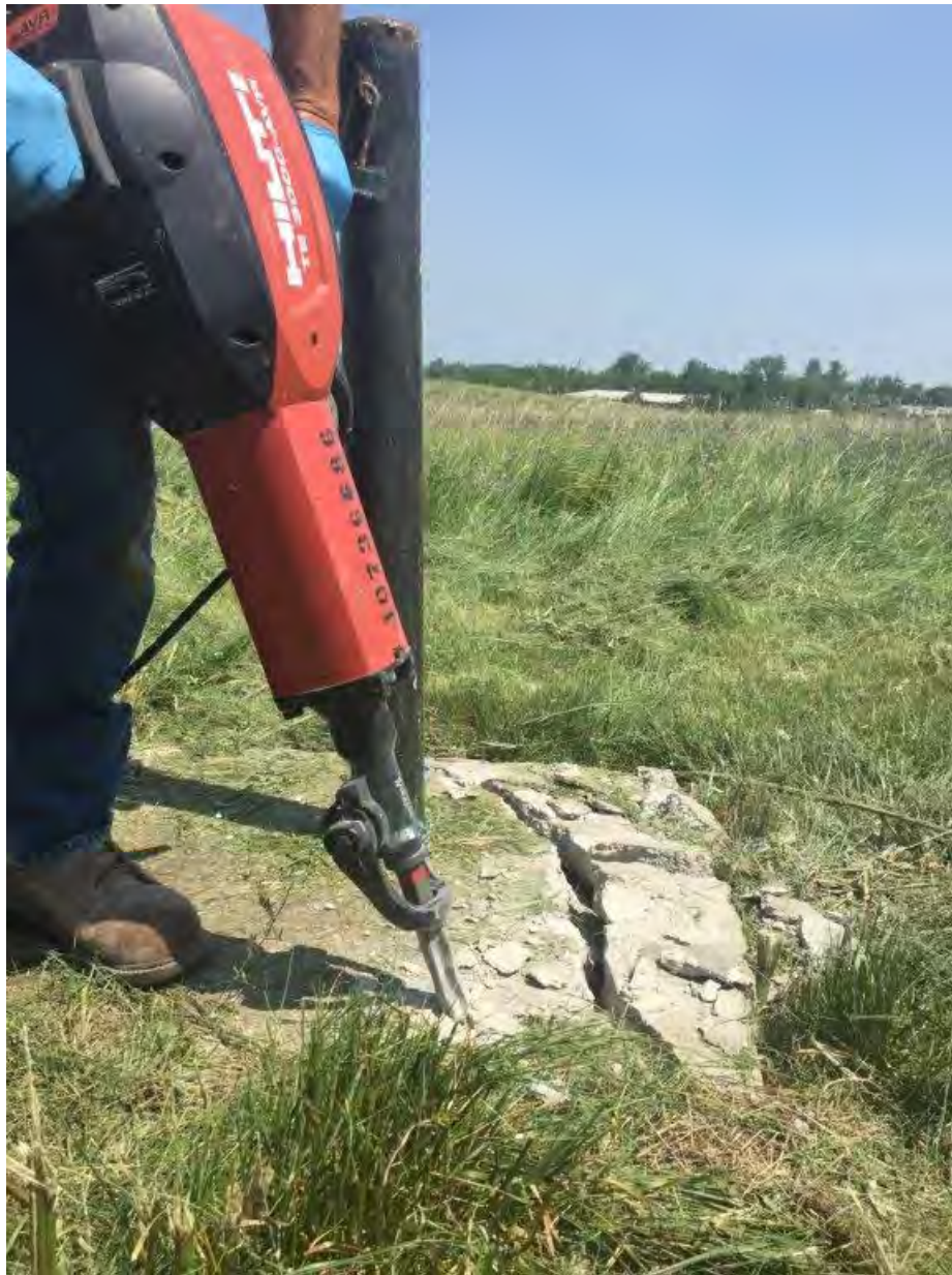
PZ-16 : removal of concrete pad
