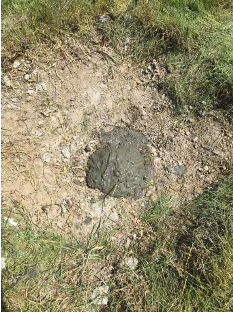
PZ-14 : Piezometer filled with concrete 12" below grade
