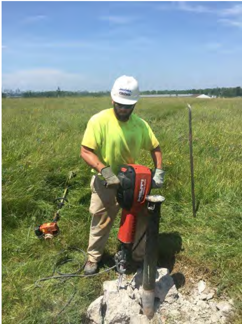
PZ-14 : removal of concrete pad
