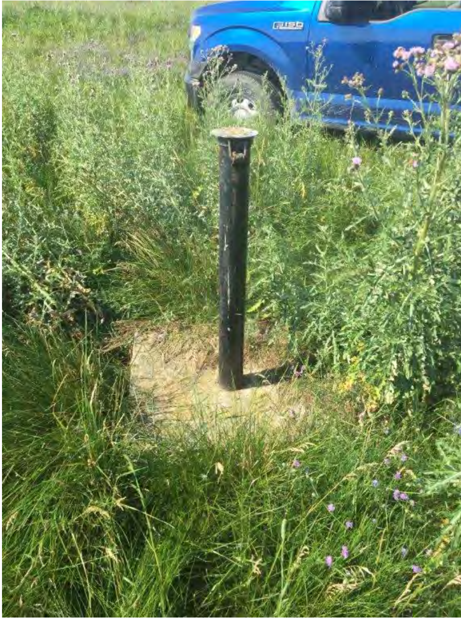
PZ-16 prior to removal
