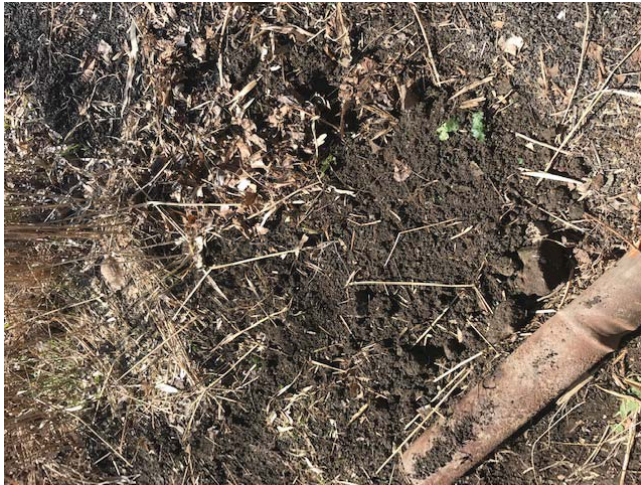
Honeywell Alltift MW#1 – Final covering of former MW#1 after being removed
