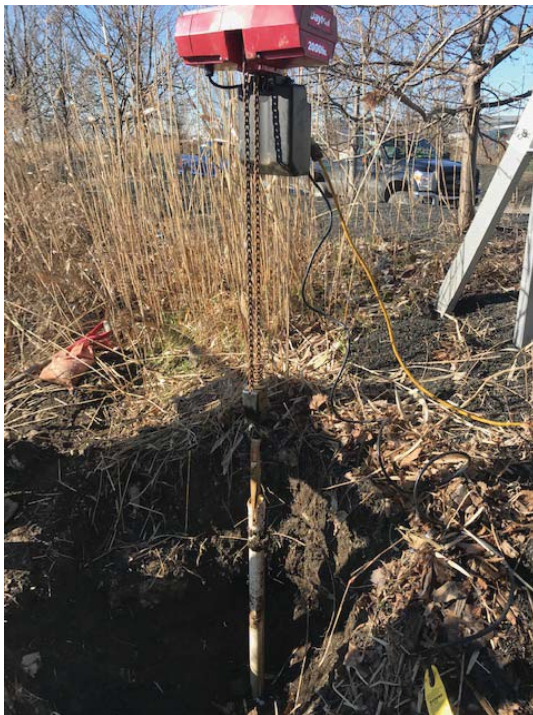
Honeywell Alltift MW#1 – Removal of MW#1
