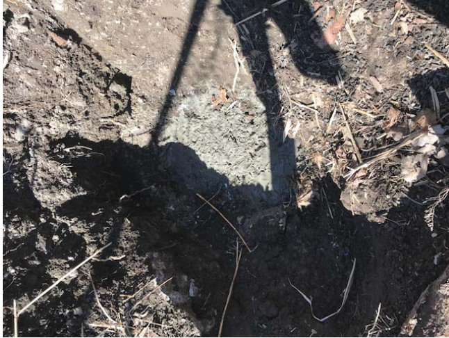
Honeywell Alltift MW#1 – MW#1 being grouted and abandoned
