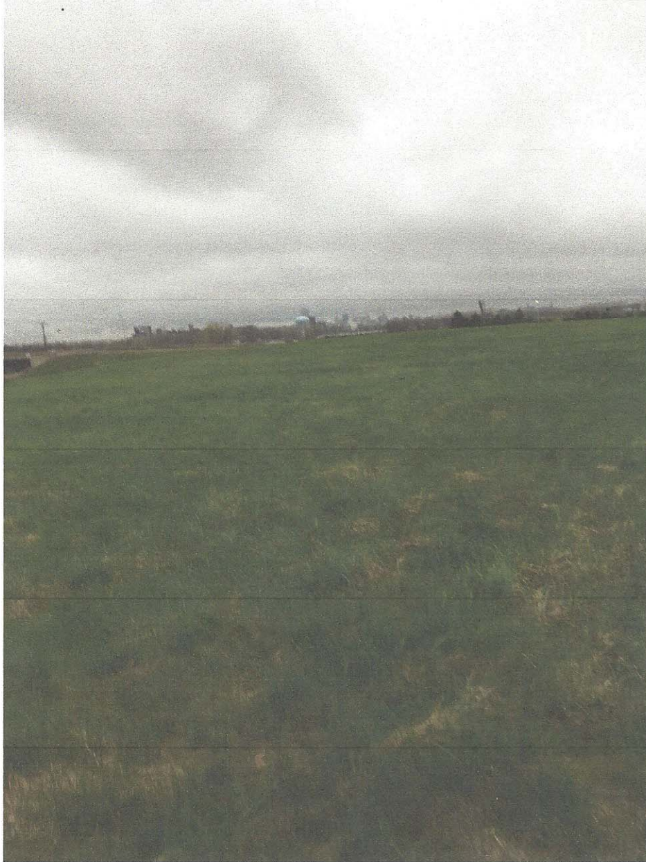
View of Alltft Landfill cap facing north
