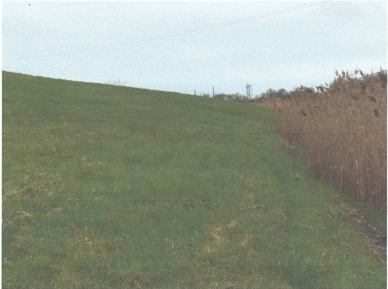
View of east side of Alltift Landfill cap facing north
