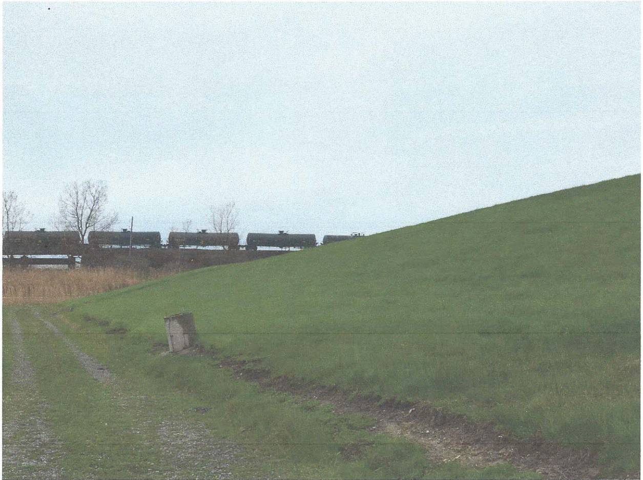
View of south side of Alltift facing west along access road.
