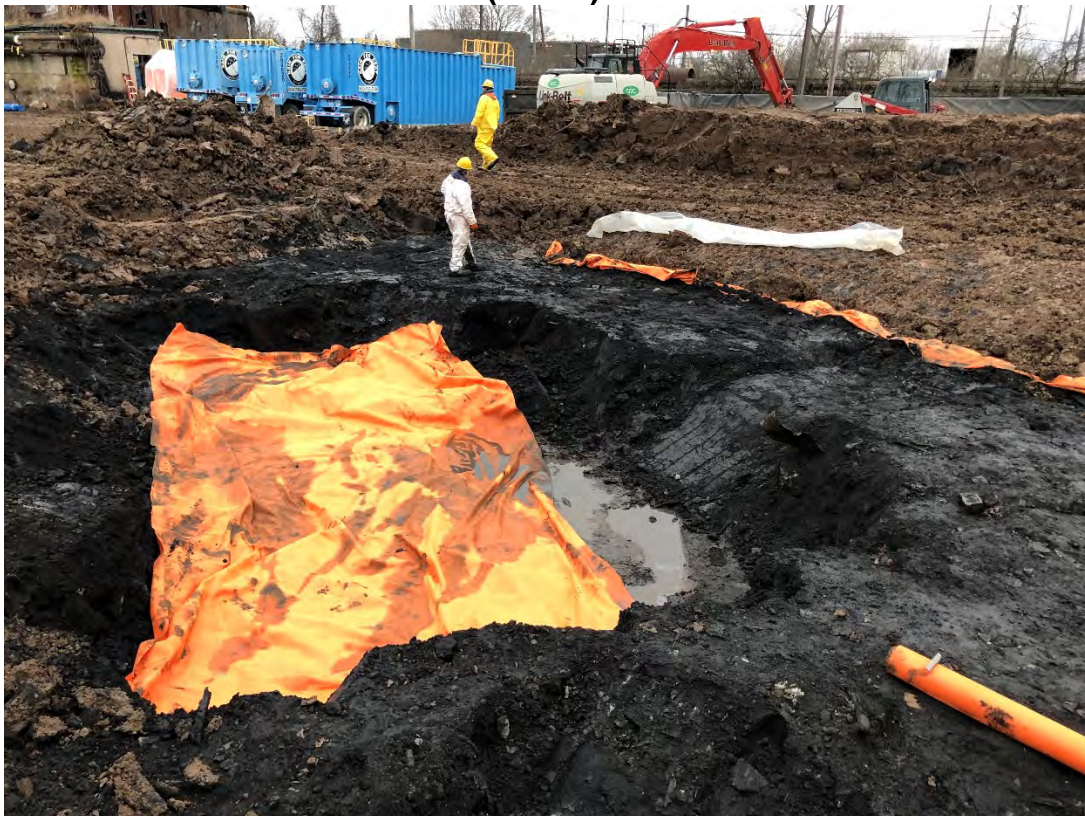
Facing north –Tank 3 excavation completed; demarcation layer installed prior to backfill (1-9-20).
