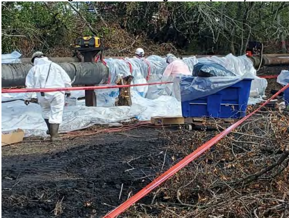
Facing northeast - Glovebag removal (10-1-20).
