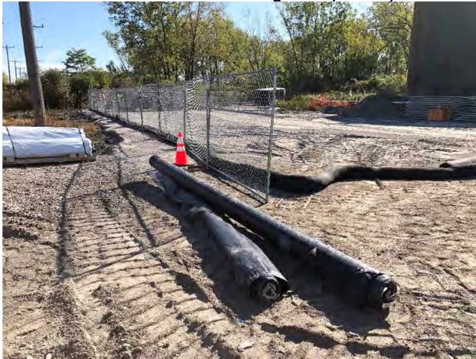
Facing east - Decontamination pad construction. Silt sock used for berm. Tank 3 visible in the background (10-8-19).
