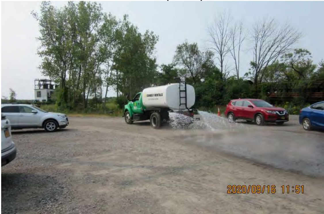
Facing west - Water truck used to address dusty conditions overloading air sample cassettes (9-16-20).
