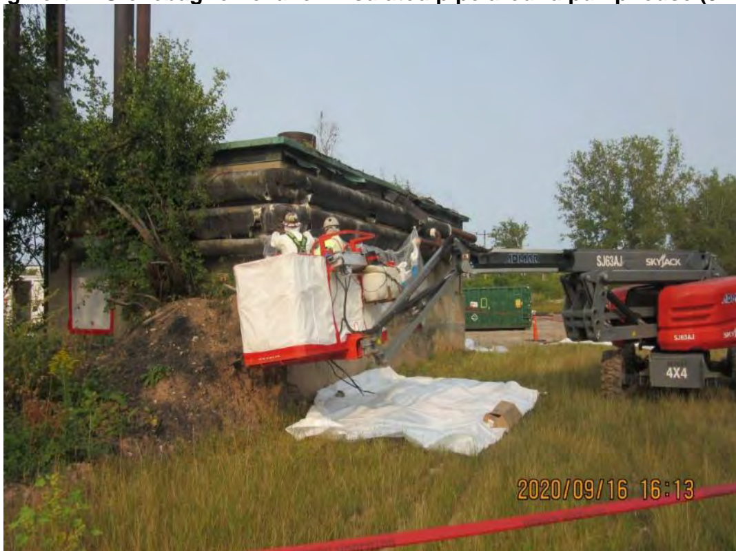
Facing north - Glovebag removal on insulated pipe around pumphouse (9-16-20).
