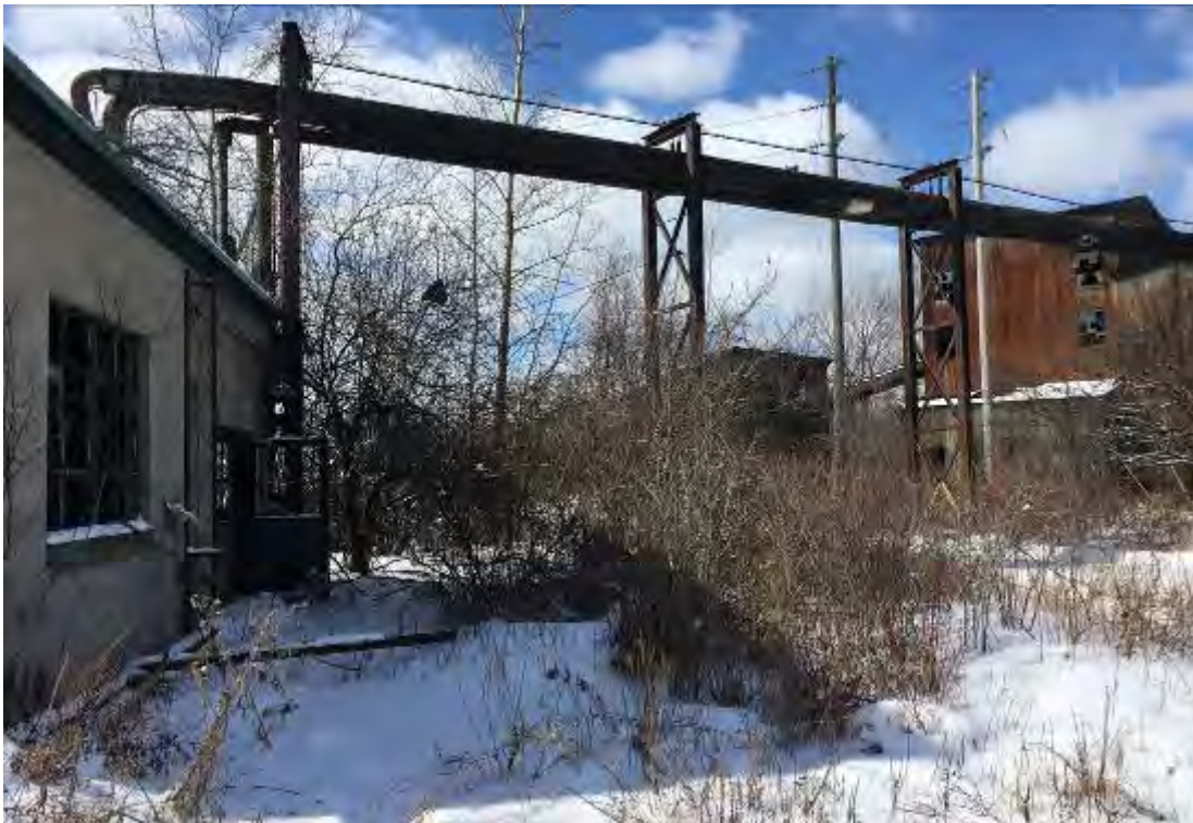
Exterior of building (at left) with ACM piping on overhead rack towards conveyor area
