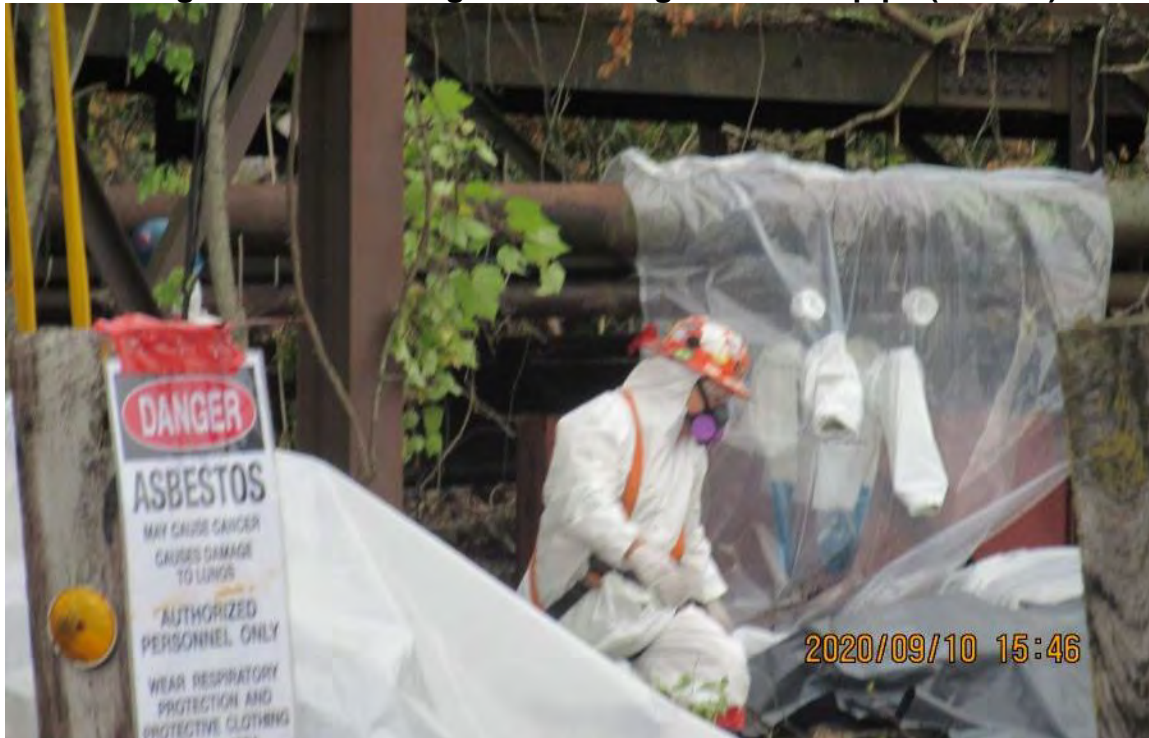
Facing south - Glovebag removal on ground level pipe (9-10-20).
