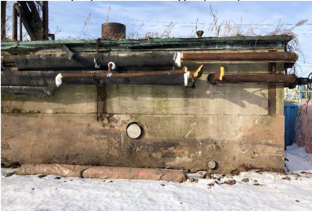
Facing north - Product piping cut flush to the pump house wall and capped (1-22-20).
