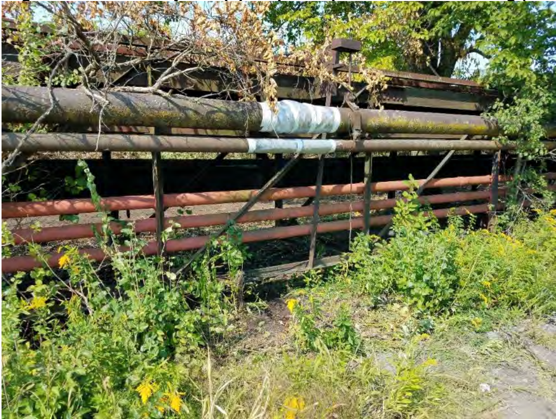
Facing northeast - Conveyance pipe repair to prevent tar from leaking (9-9-20).
