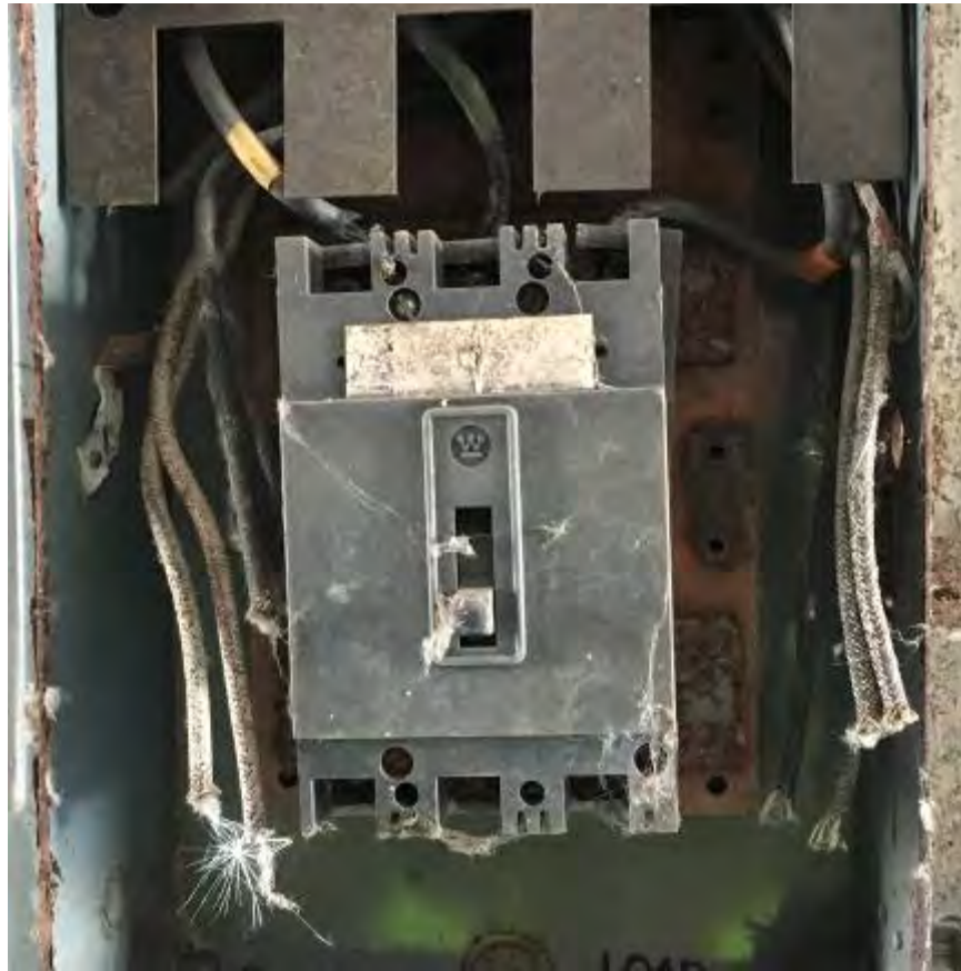
PACM cloth wrap on electrical wiring
