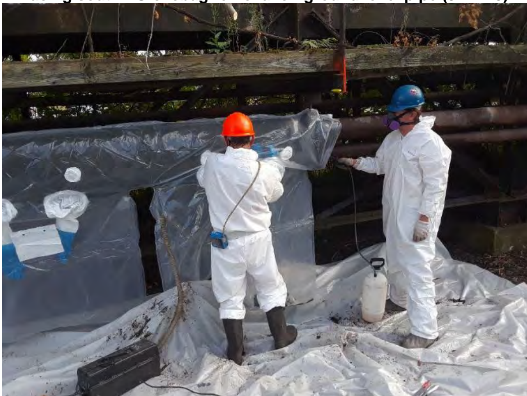
Facing south - Glovebag removal on ground level pipe (9-17-20).
