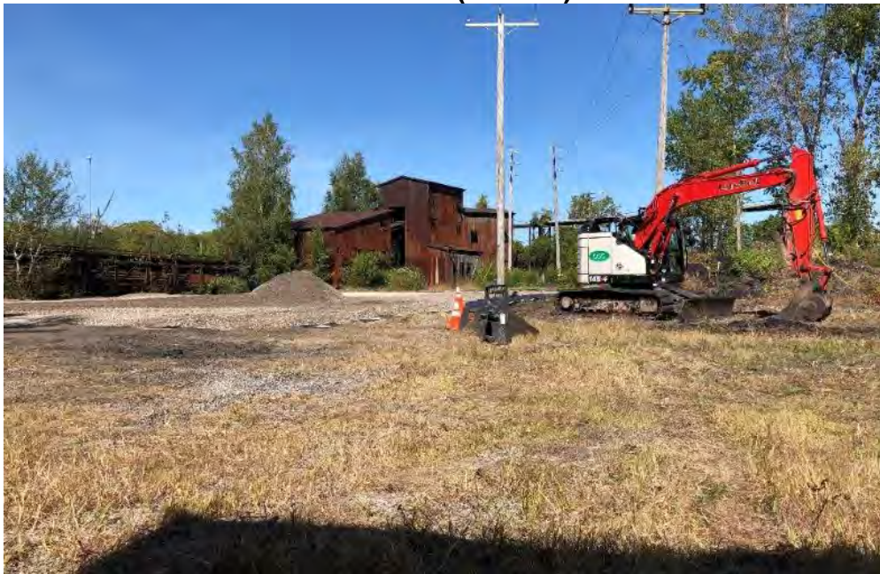
Facing northeast - Support zone construction. Geotextile woven fabric installed below road stone (9-17-19).
