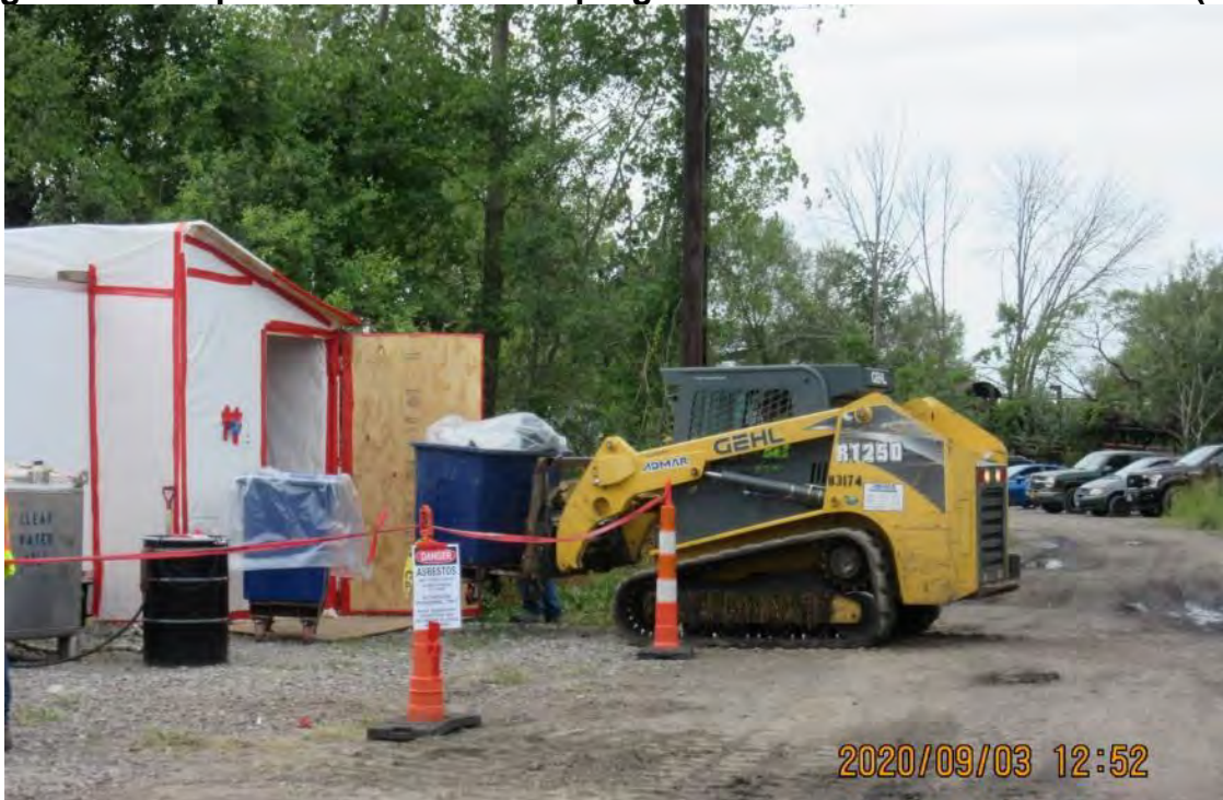
Facing west - Pumphouse abatement in progress: loadout of asbestos waste (9-3-20).
