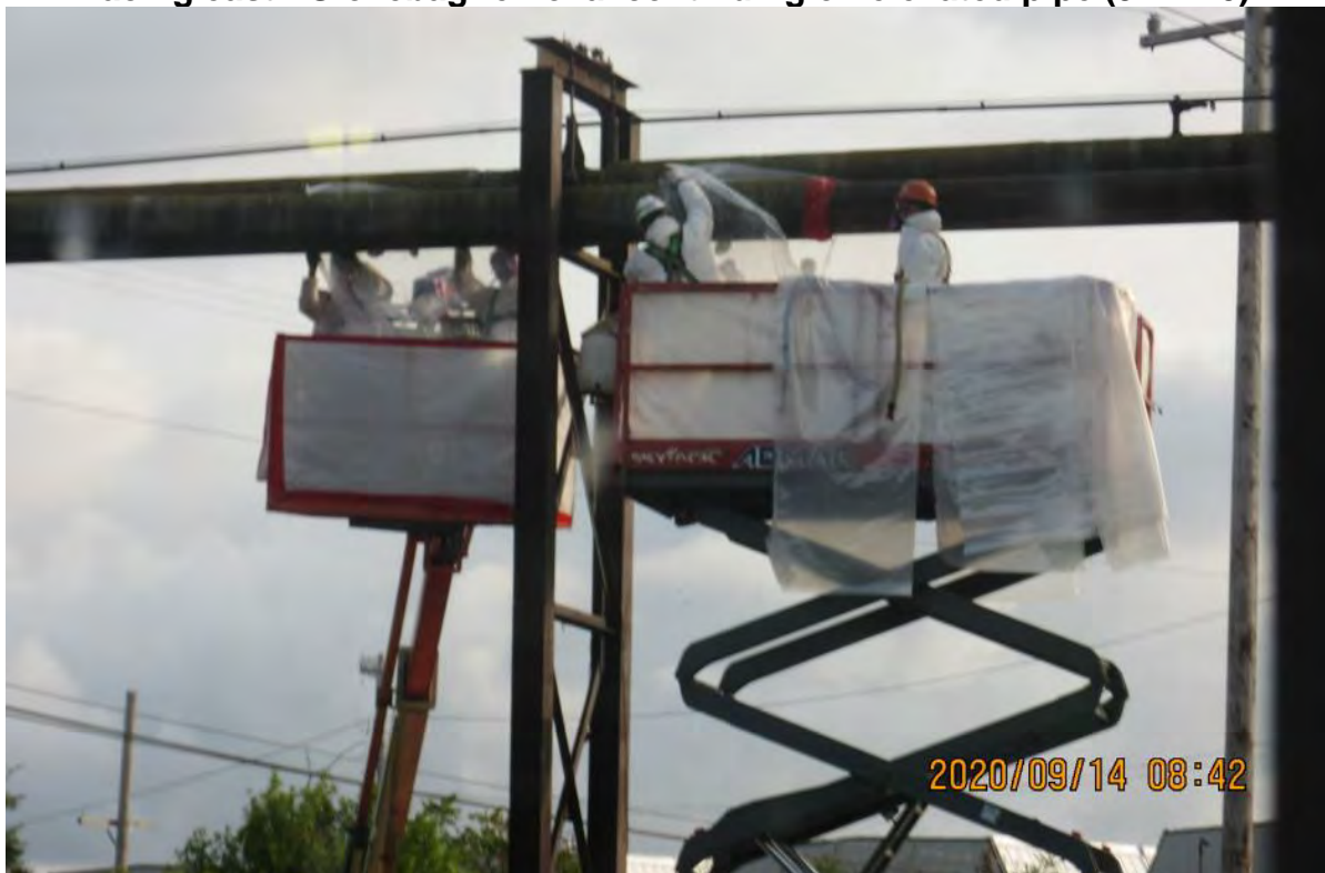
Facing east - Glovebag removal continuing on elevated pipe (9-14-20).
