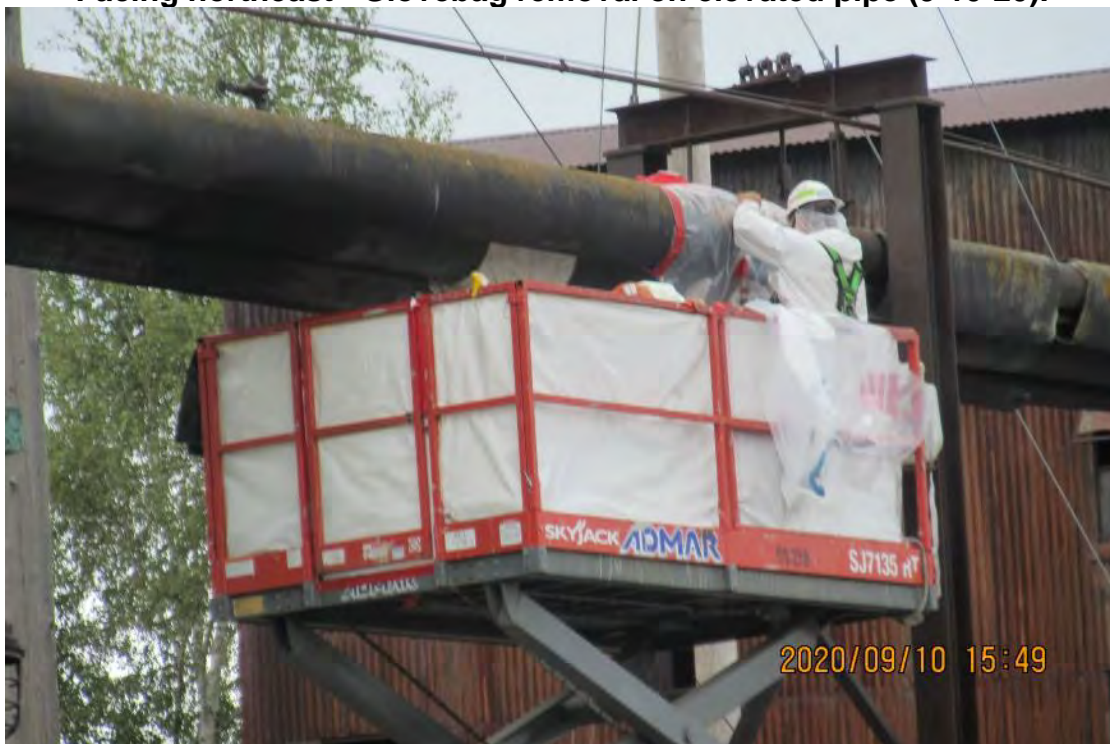
Facing northeast - Glovebag removal on elevated pipe (9-10-20).
