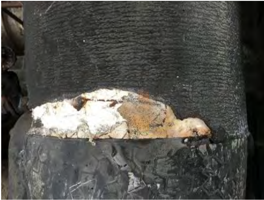
Black pipe wrap with wire (lower pipe) and tar-paper-like wrap on upper pipe
