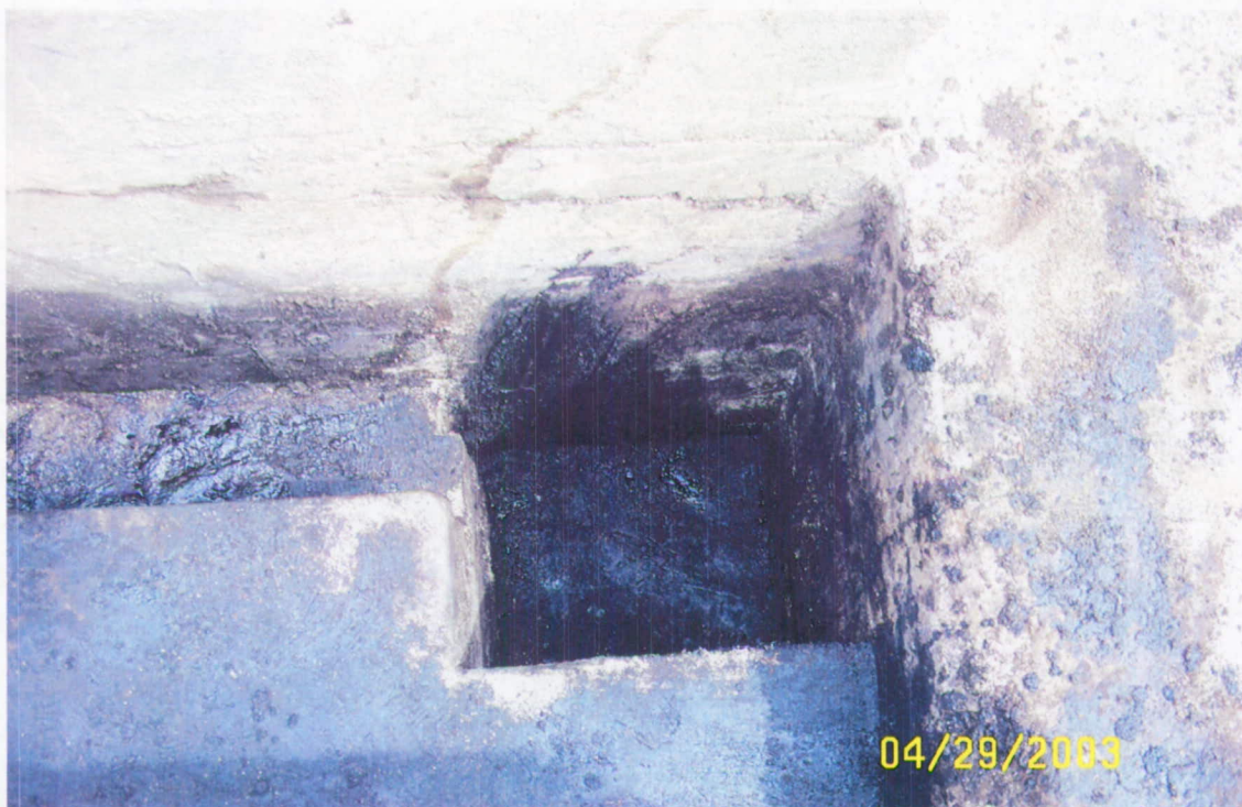
Pit-6 sump corner during excavation.
