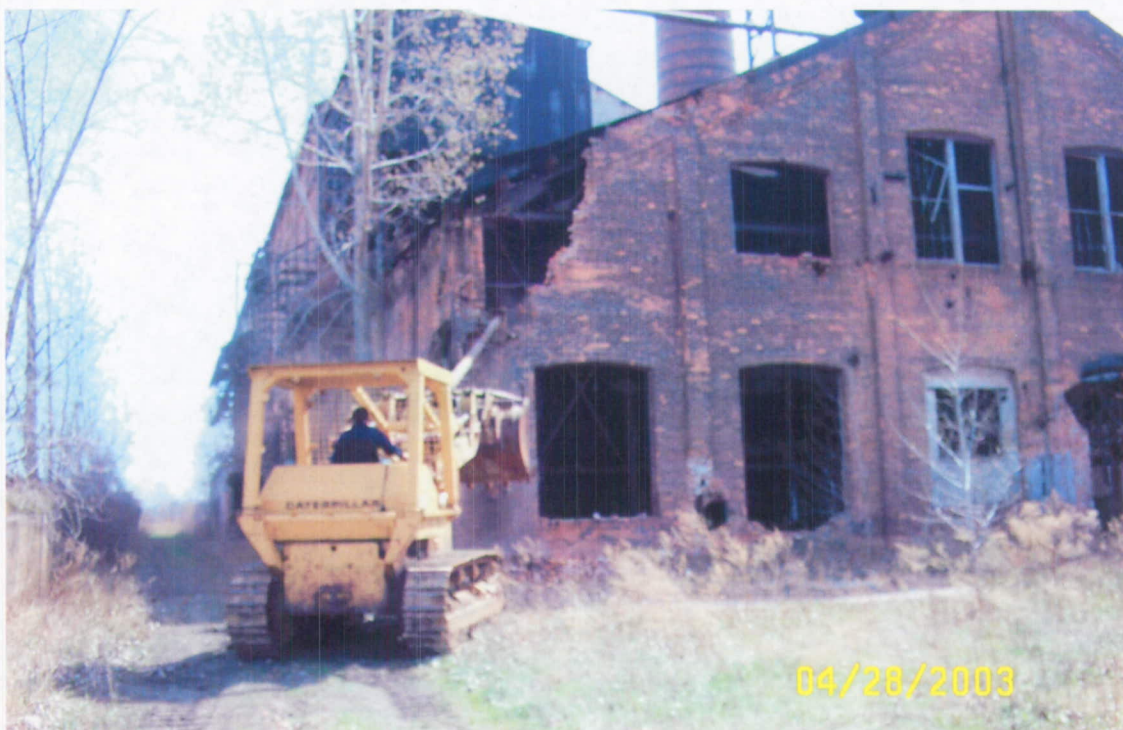
Boiler House, loose bricks removed before excavation activities.
