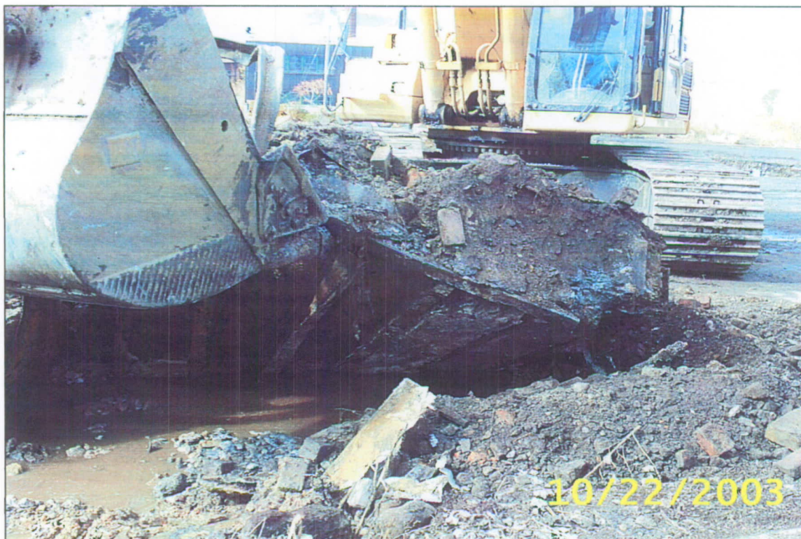
Photograph #16: Apparent containment structure exposed in the unidentified pit.
