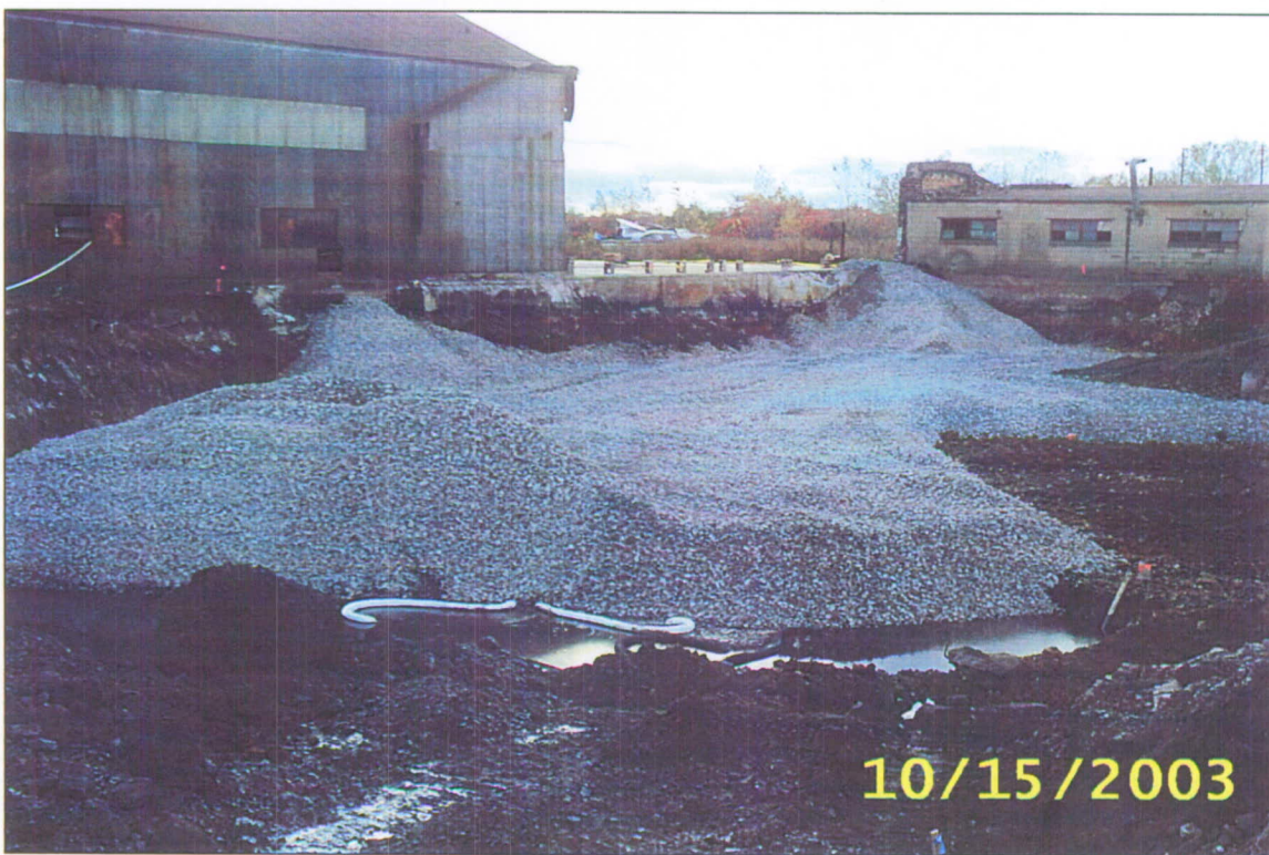
Photograph #10: Placing #3 crushed limestone up to, and into hazardous waste area.
