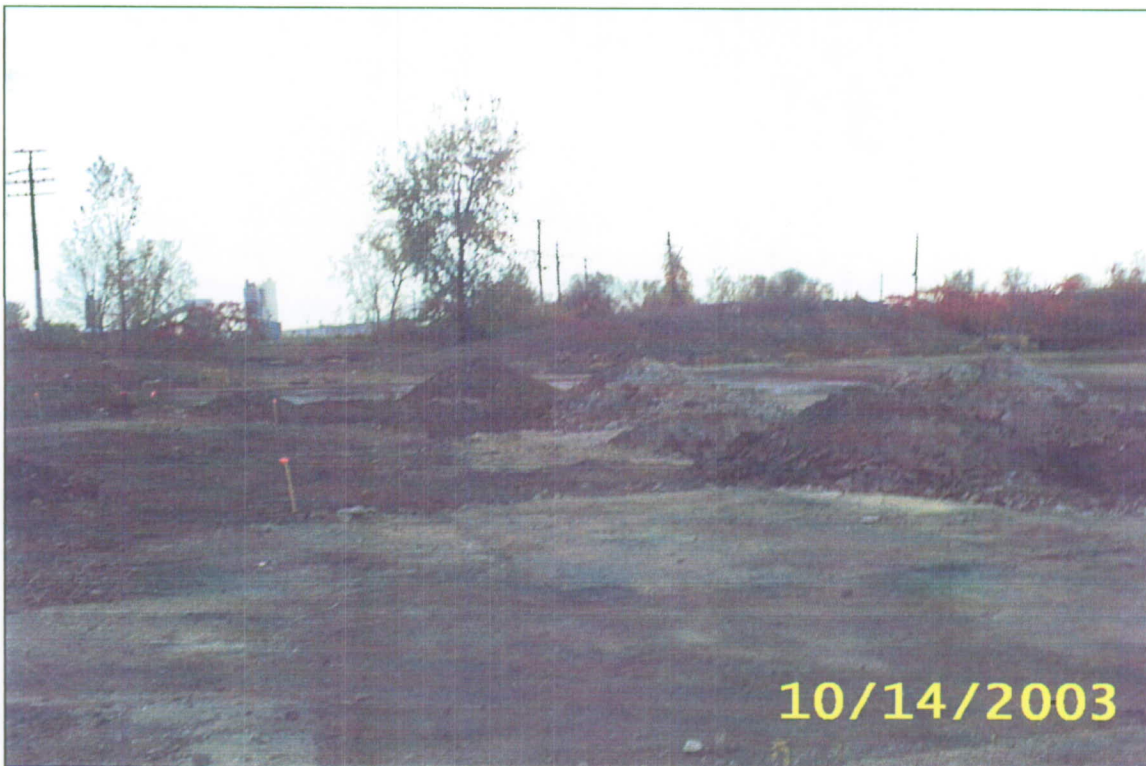
Photograph #6: Test pits excavated for in-situ sampling of reusable soil.
