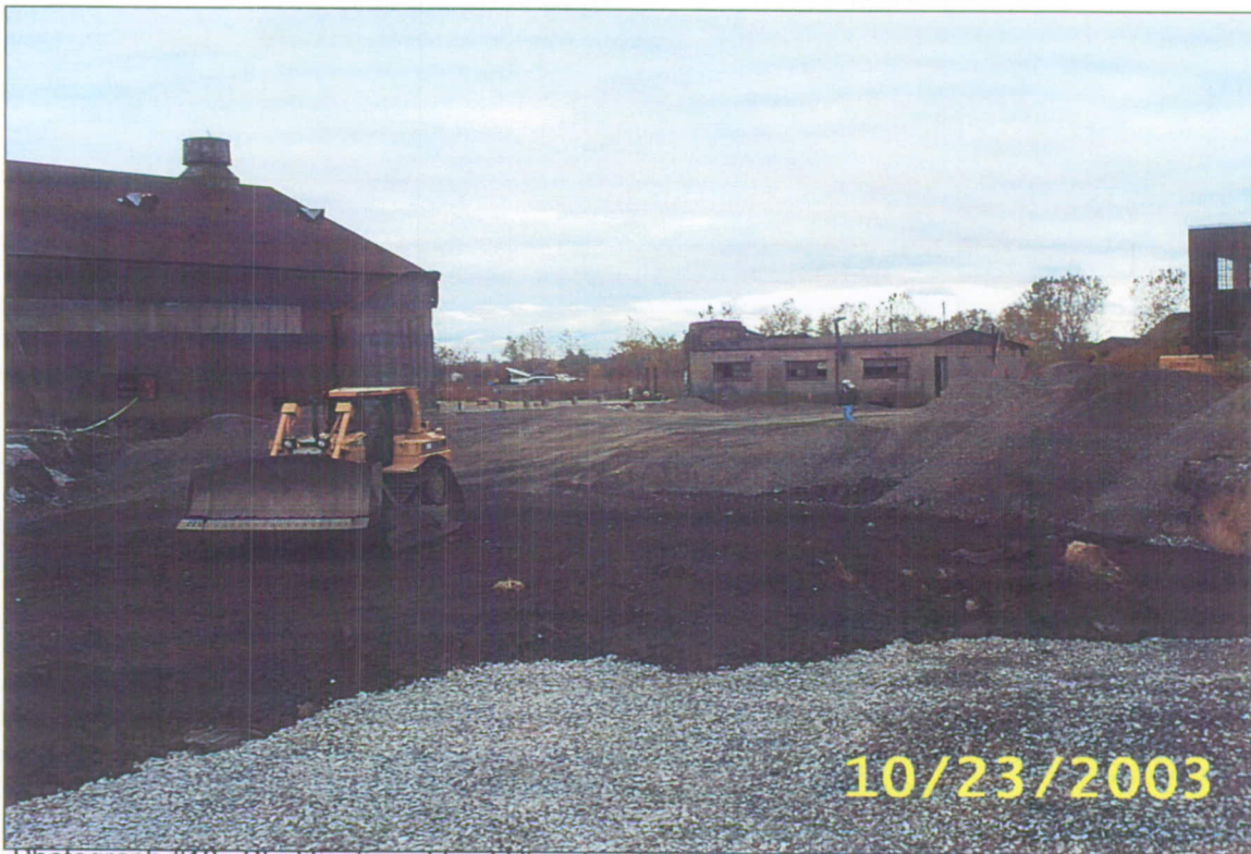
Photograph #18: Stratification of backfill materials.
