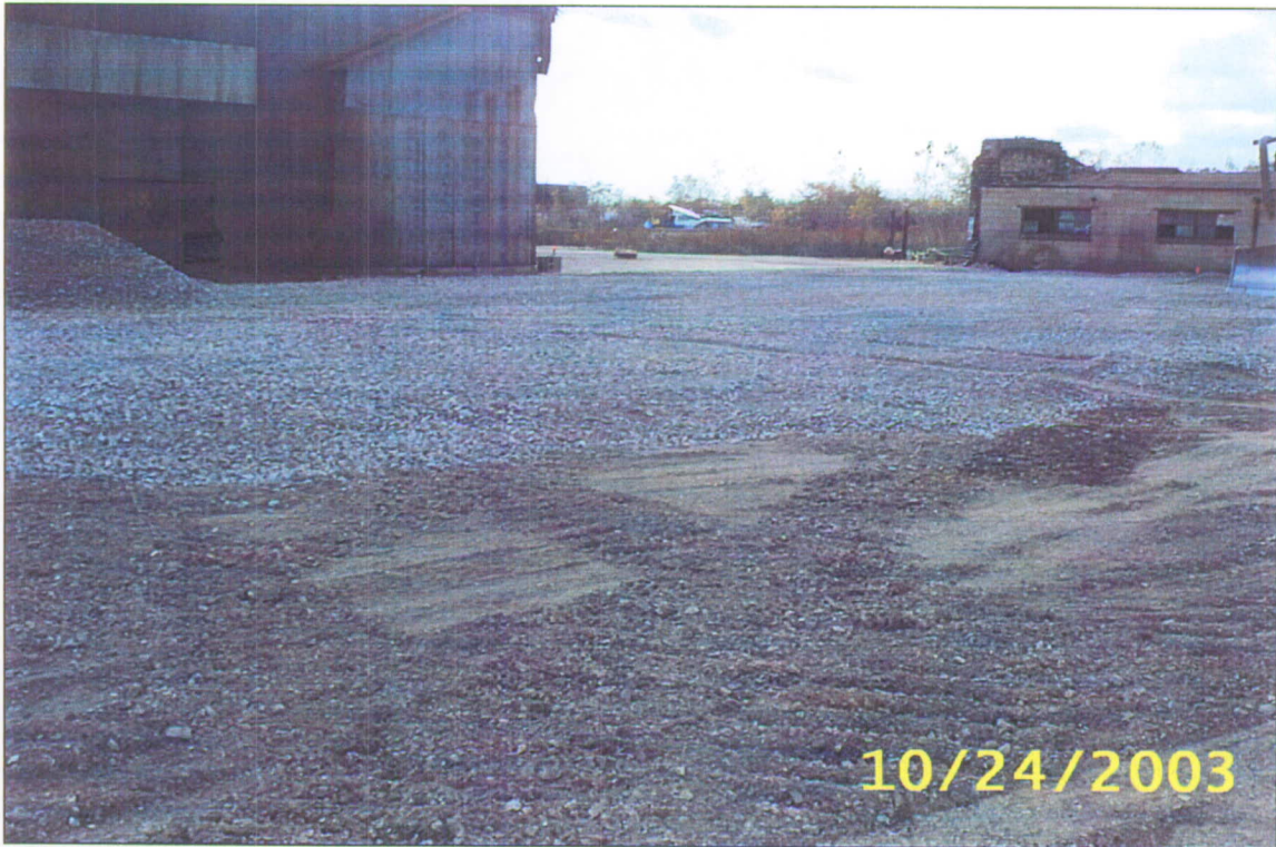
Photograph #20: 12" lift of #2 crushed limestone at surface.
