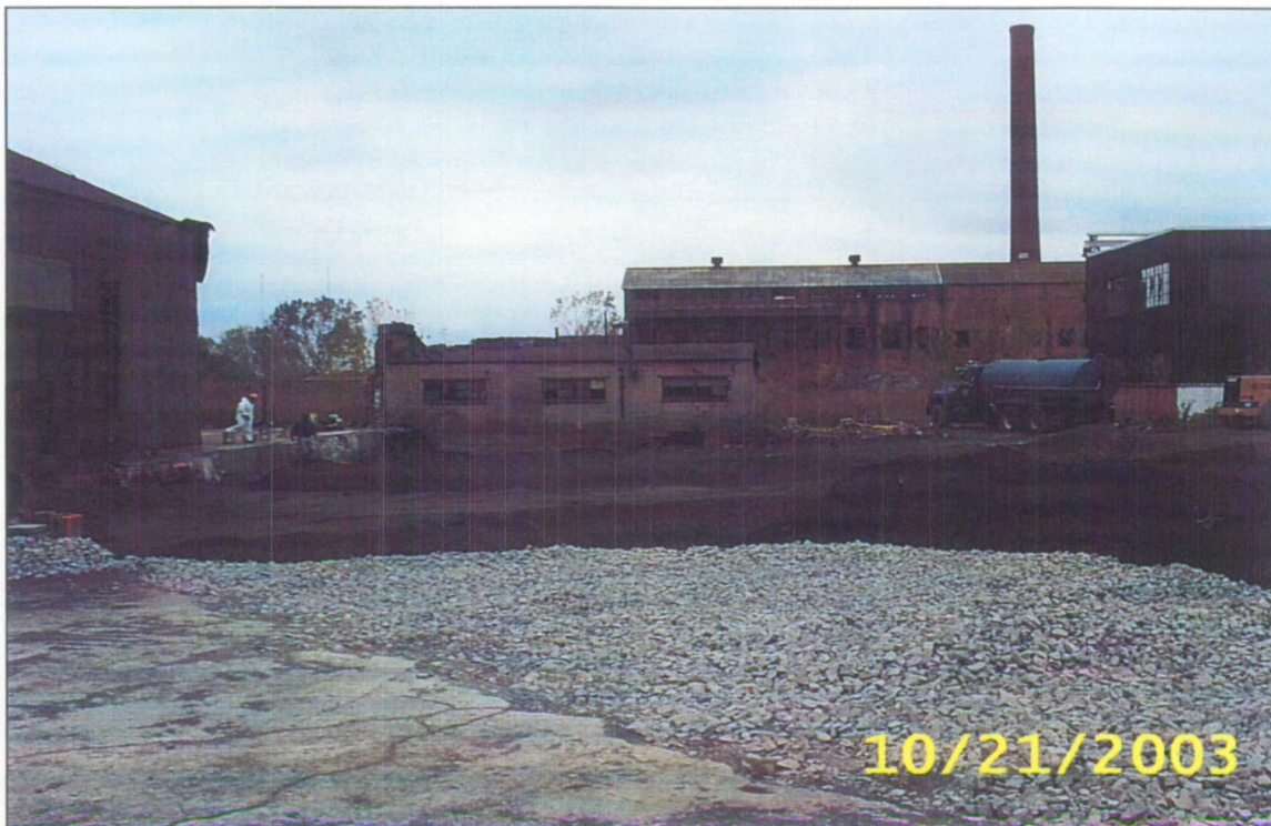
Photograph #15: Recycled concrete being placed and compacted.
