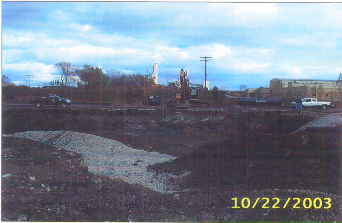
Photograph #17: Final limits of eastern excavation.
