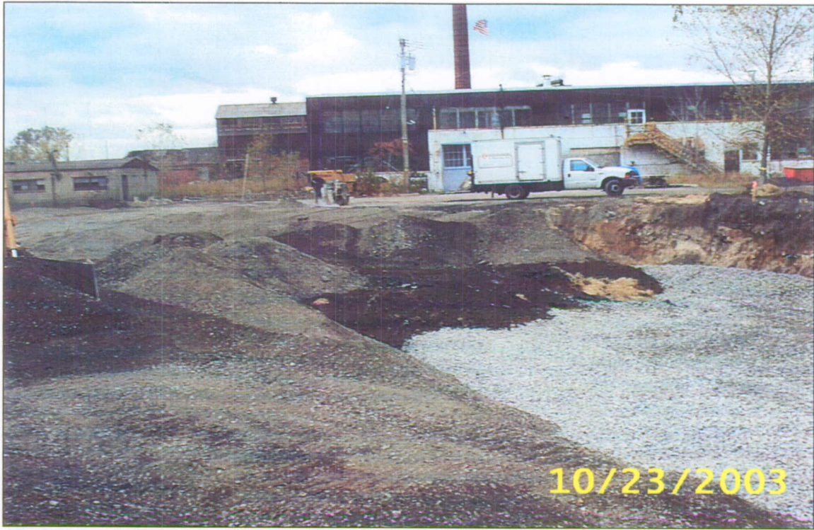
Photograph #19: Limits of reusable soil at northeastern corner.
