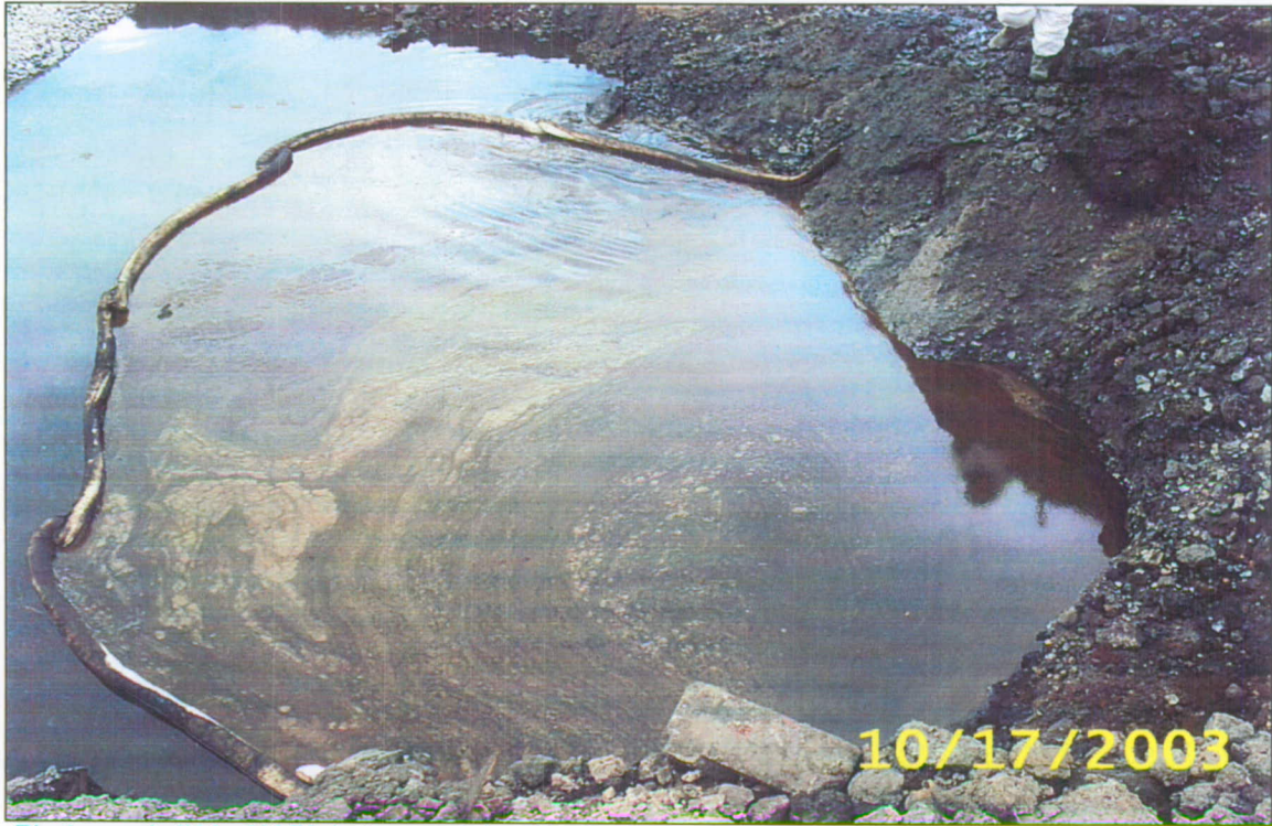
Photograph #11: NAPL being contained in the hazardous waste excavation.
