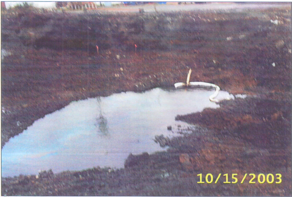
Photograph #8: Hazardous waste excavation (under water).
