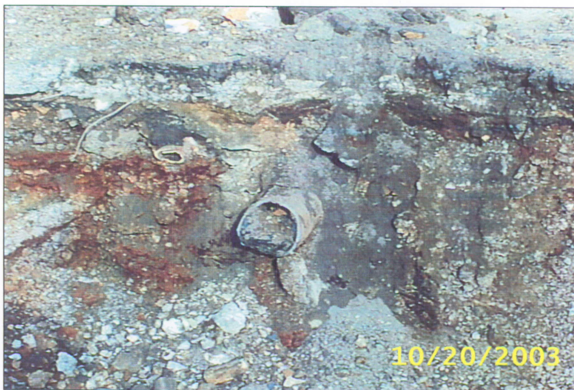
Photograph #14: Steel pipe exposed during excavation at east end.
