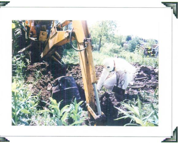
Test Pit excavation in disposal area reveals buried drum. Technician monitors VOC emissions.
