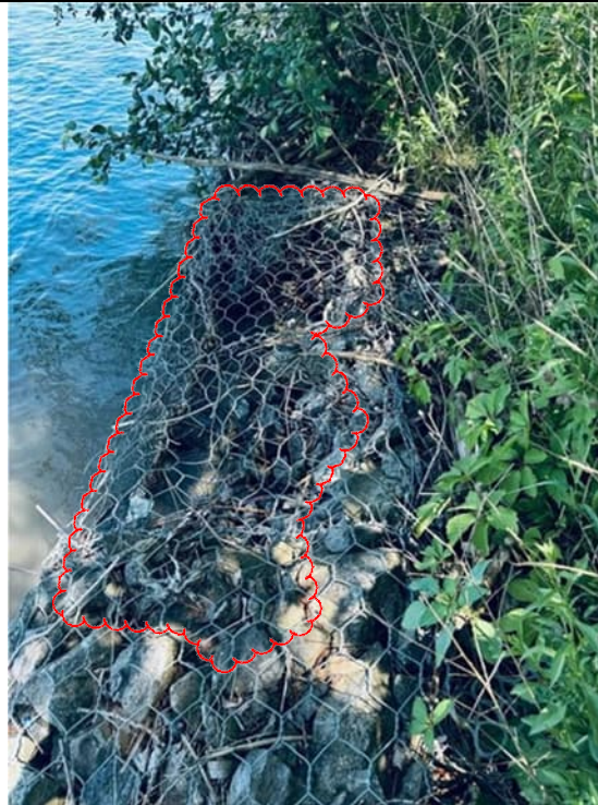
Photograph 4. Gabion wall deterioration/voids just north of the stream gauge.
