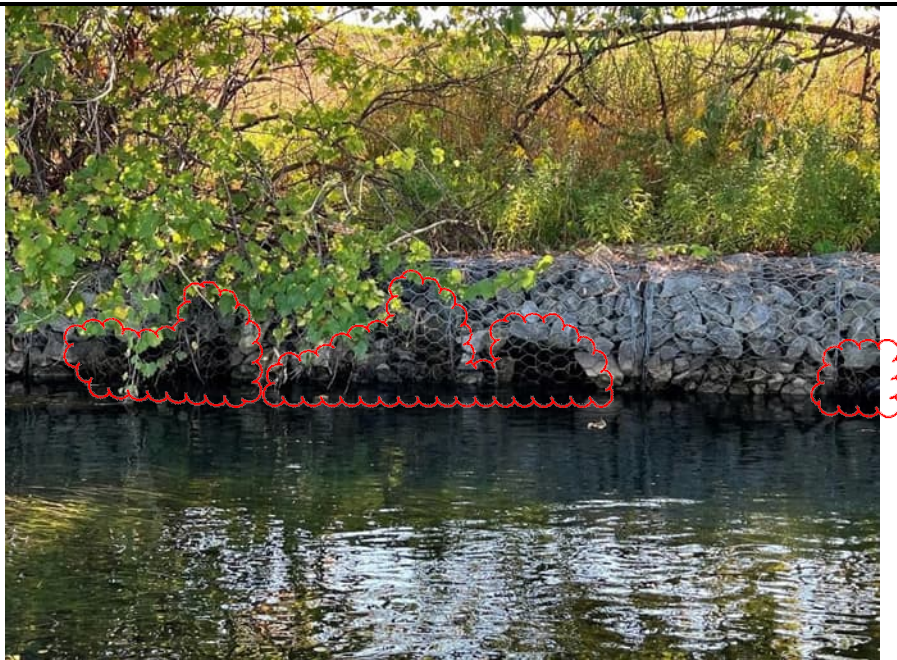
Photograph 10. Additional locations along the gabion wall that show additional rock material falling out of the upper baskets. View is from the Niagara River as the boat travels north along the western side of the Niagara Mohawk-Cherry Farm Site. Location appears to be near Sump 2.
