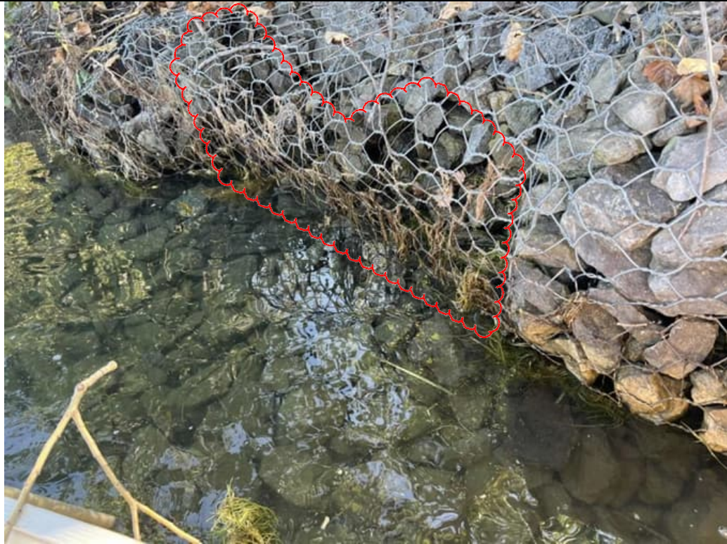
Photograph 5. Closer view of the gabion wall deterioration just north of the stream gauge. View is from the Niagara River.
