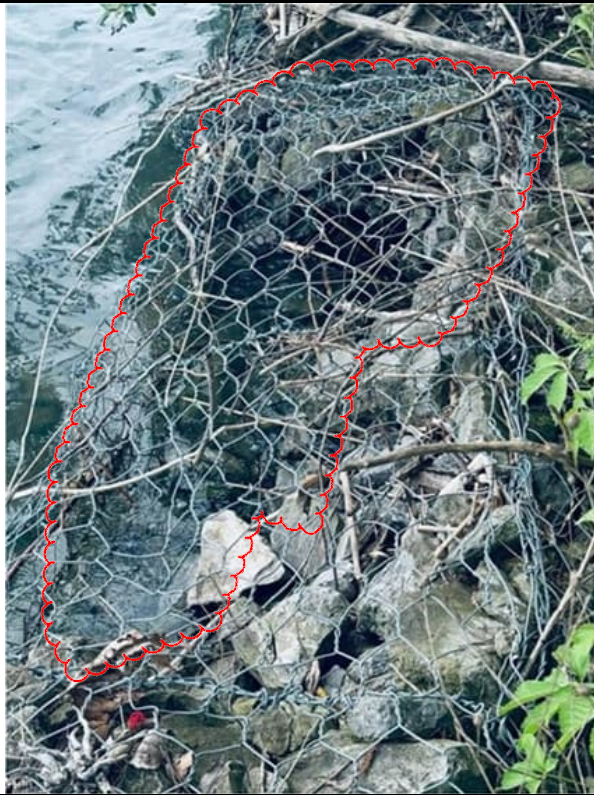
Photograph 3. Gabion wall deterioration just north of the stream gauge.
