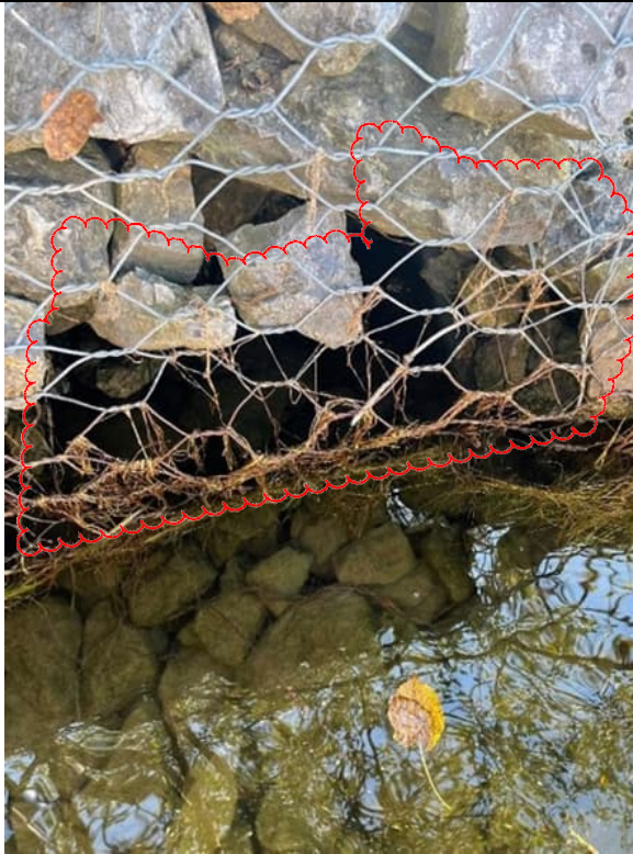
Photograph 9. Closer view of the Gabion Basket voids.
