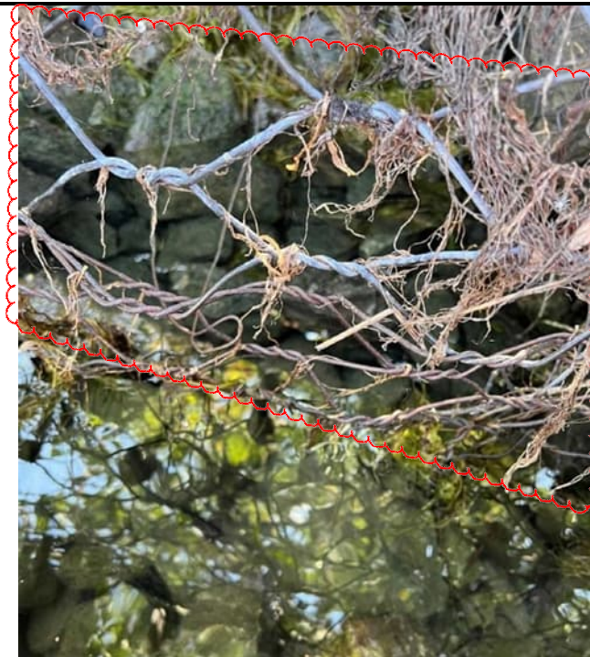
Photograph 6. Closer view of the wire mesh failure on the gabion wall. View is from the Niagara River at the spot just north of the stream gauge.
