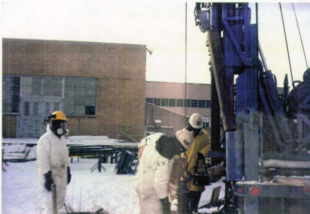
Area I - Oil Storage Building Installation of MW-7
