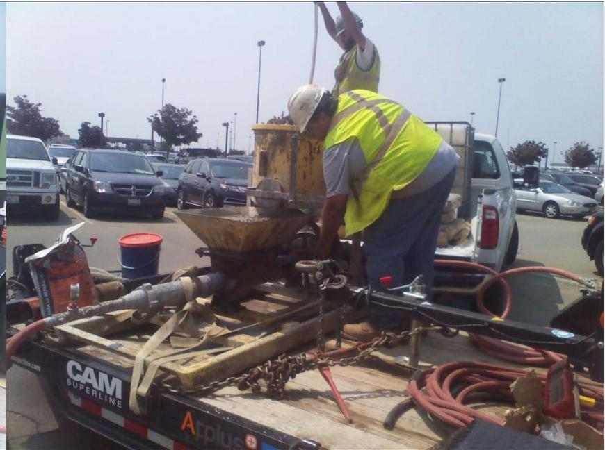
Photograph 14, August 2, 2014: Mixing grout.
