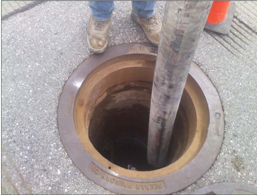
Photograph 1, July 14, 2014: Pumping concrete into MH001-10.
