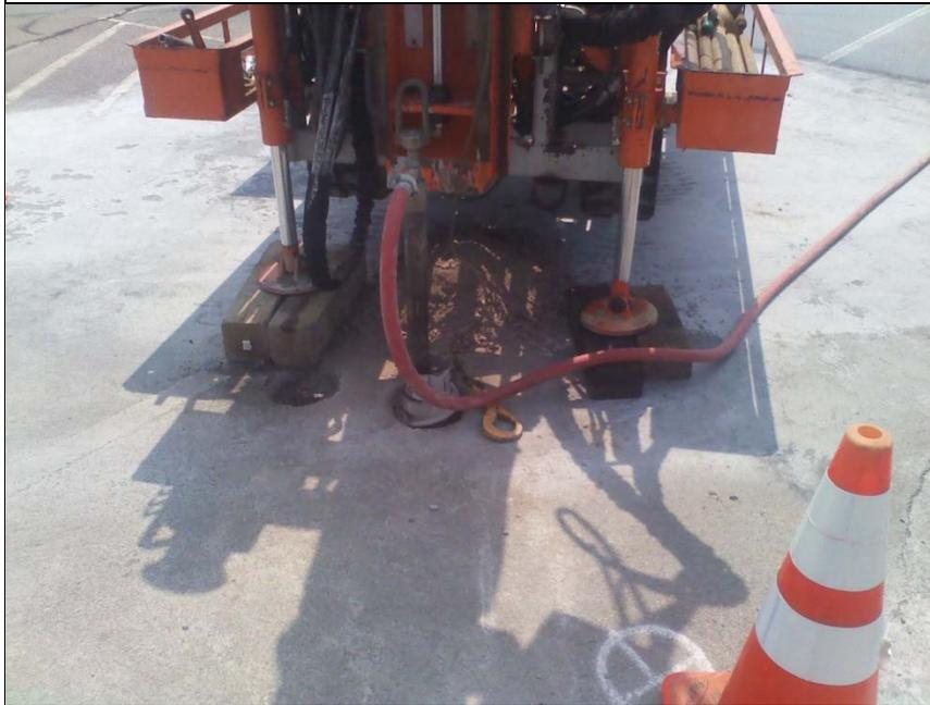
Photograph 15, August 2, 2014: Injecting grout around MH002-02.
