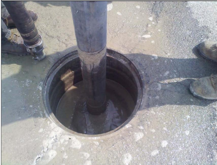
Photograph 11, July 29, 2014: Pumping grout into CSMH-003.
