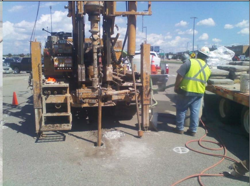
Photograph 16, September 3, 2014: Drilling grout hole at MH003-01.
