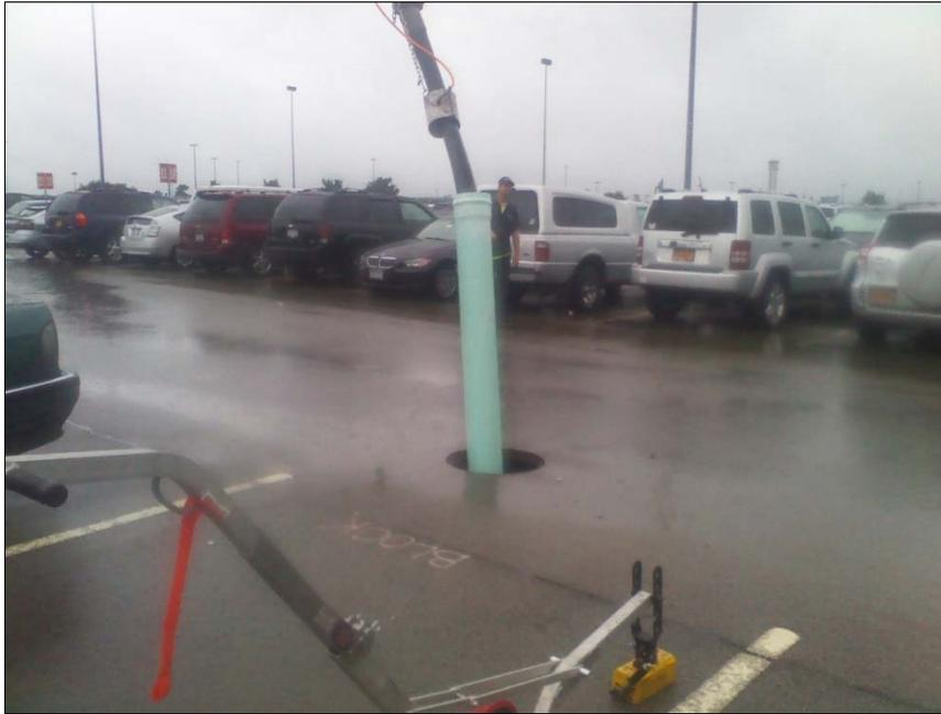
Photograph 9, July 28, 2014: Pumping flowable fill into MH-003-04.
