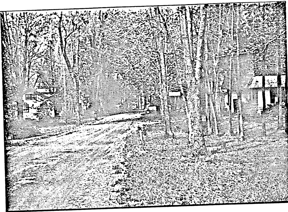
① View of typical roadway at Wide Beach. Road consists of bank-run gravel and earth.
