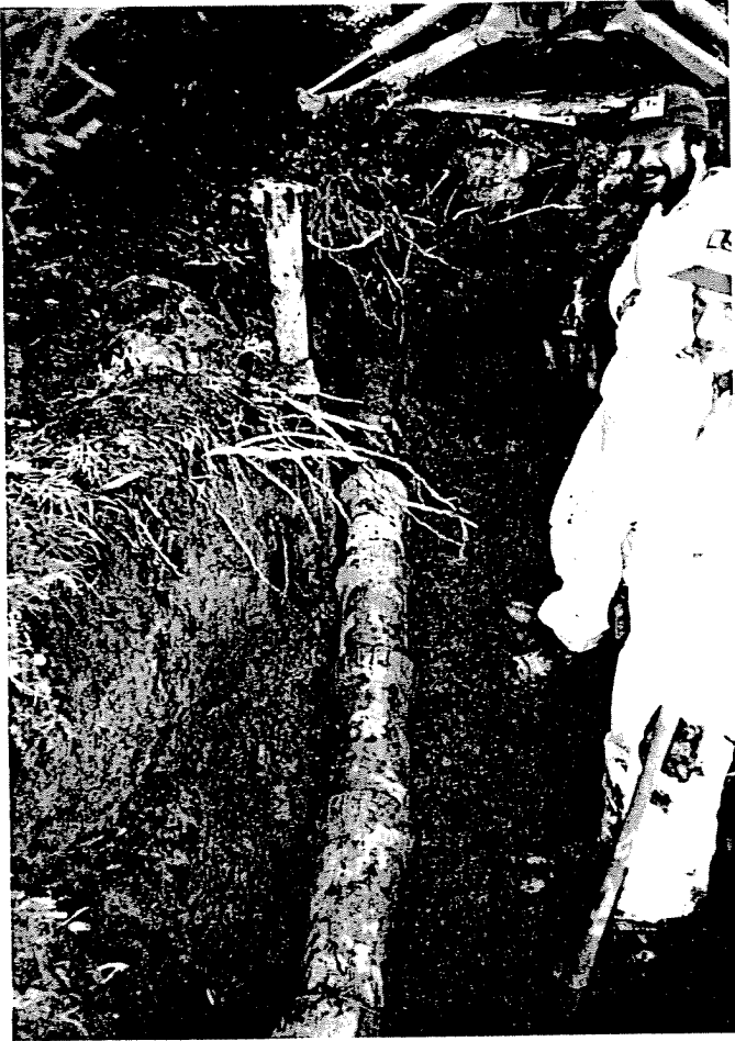
Photo #3 Refurbished 8 inch drain. Existing sampling well is left of the drain. Photo looks north.
