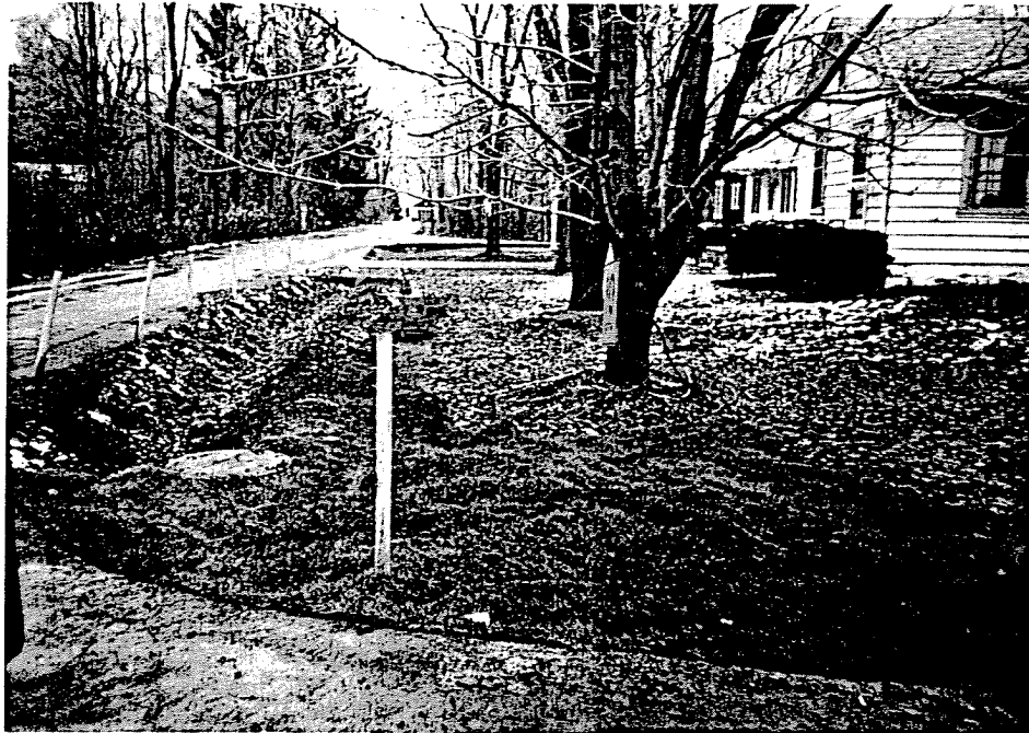
Photo #4 Finished northwest corner of south street showing one of the new manholes, drainage ditch and newly sodded area. Photo looks north.
