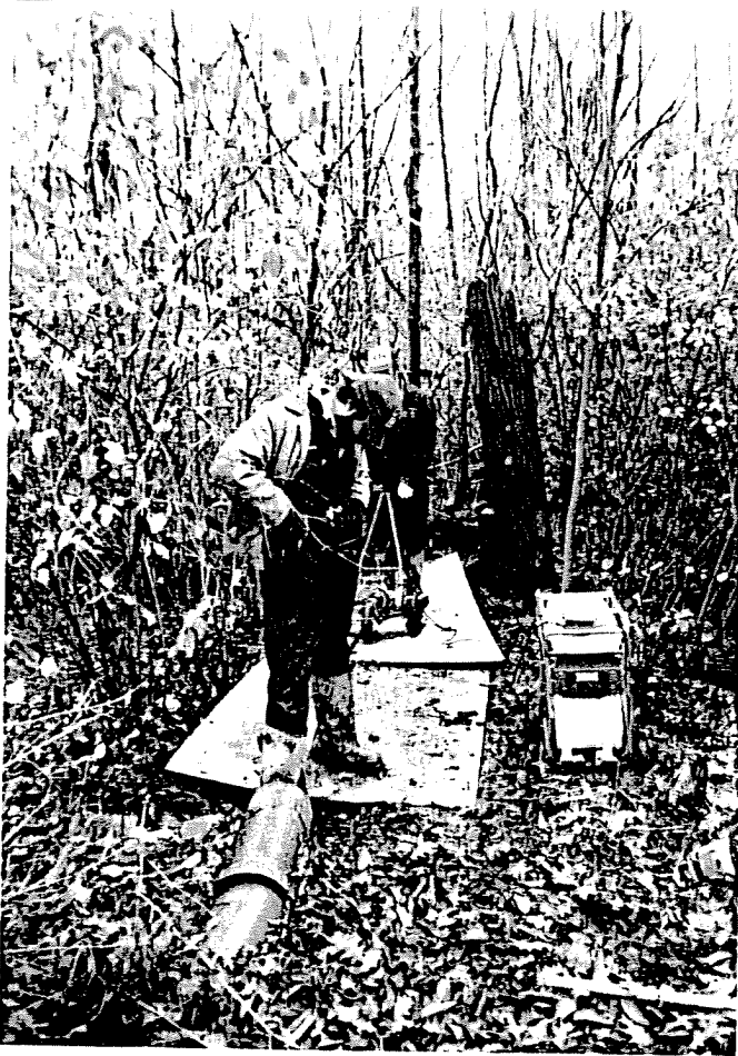
Photo #1 Roto Rooter cleaning of 8 inch pipe draining into swamp area.
