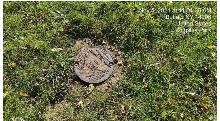
Monitoring Well MW-4
