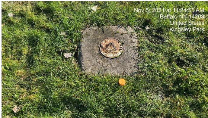
Monitoring Well MW-3
