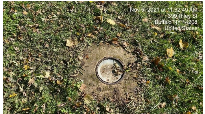
Monitoring Well MW-2
