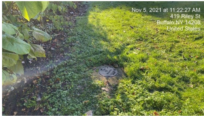
Monitoring Well MW-7
