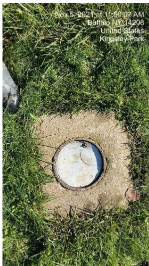
Monitoring Well MW-5
