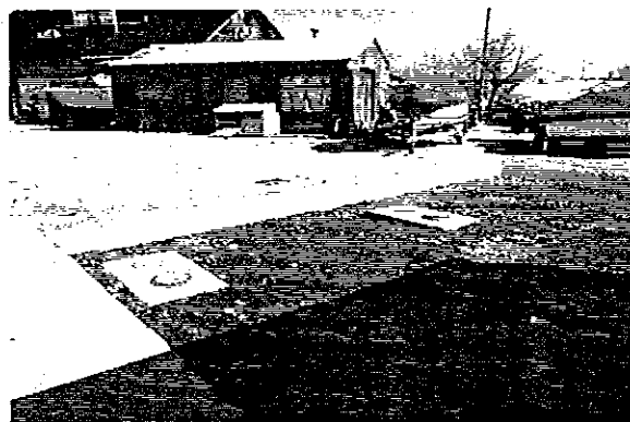
2. Location of (2) 6,000-gallon gasoline USTs, Parcel 1, looking northeast; marine repair shop in background
