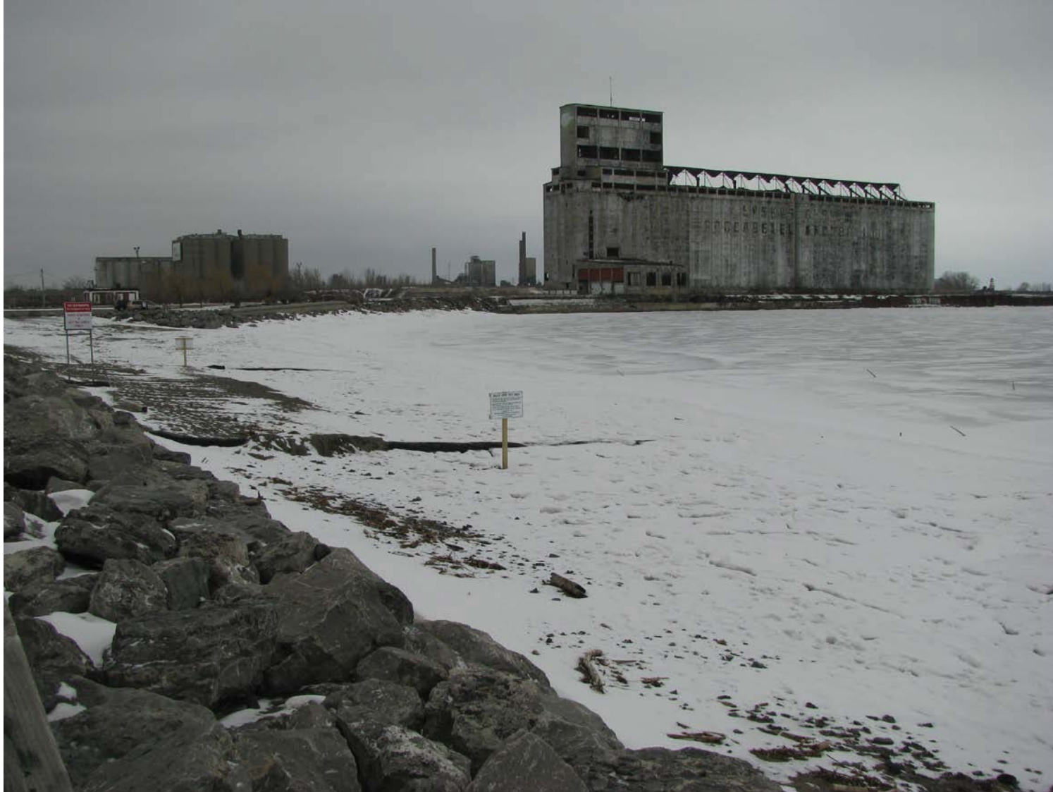
Gallagher Beach Photo 1: Looking South along the revetment at the upper edge of the test area.
