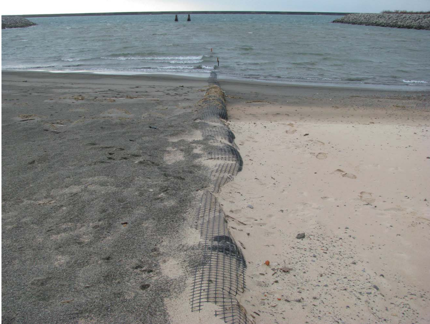
NYPA Parcel Photo 5: Looking lakeward along north edge restraint. Burial in the foreground here is at least partially the result of placement of additional (light-colored) sand on the outside of the test area.
