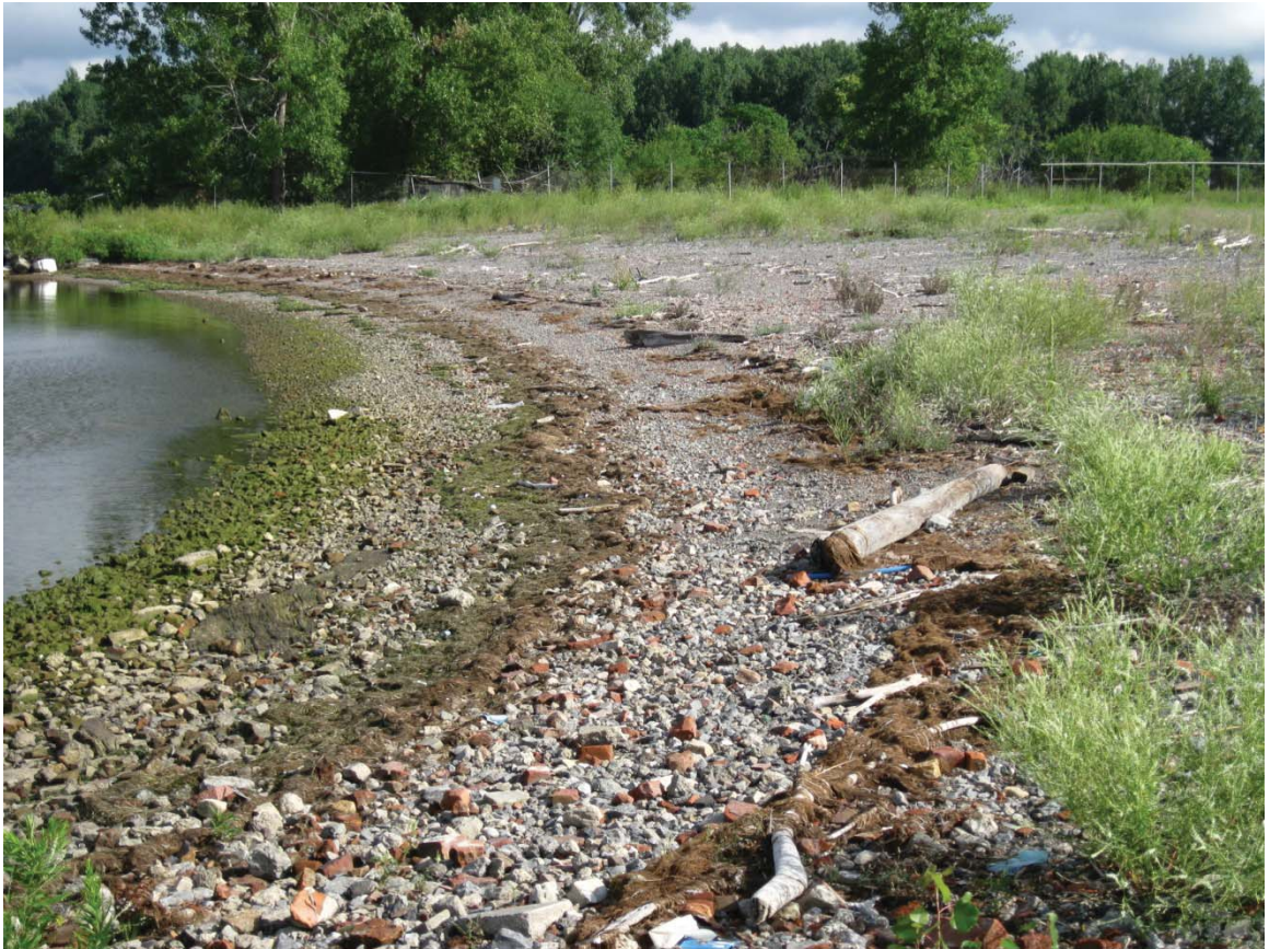
Pre-Construction conditions at the NYPA Parcel
