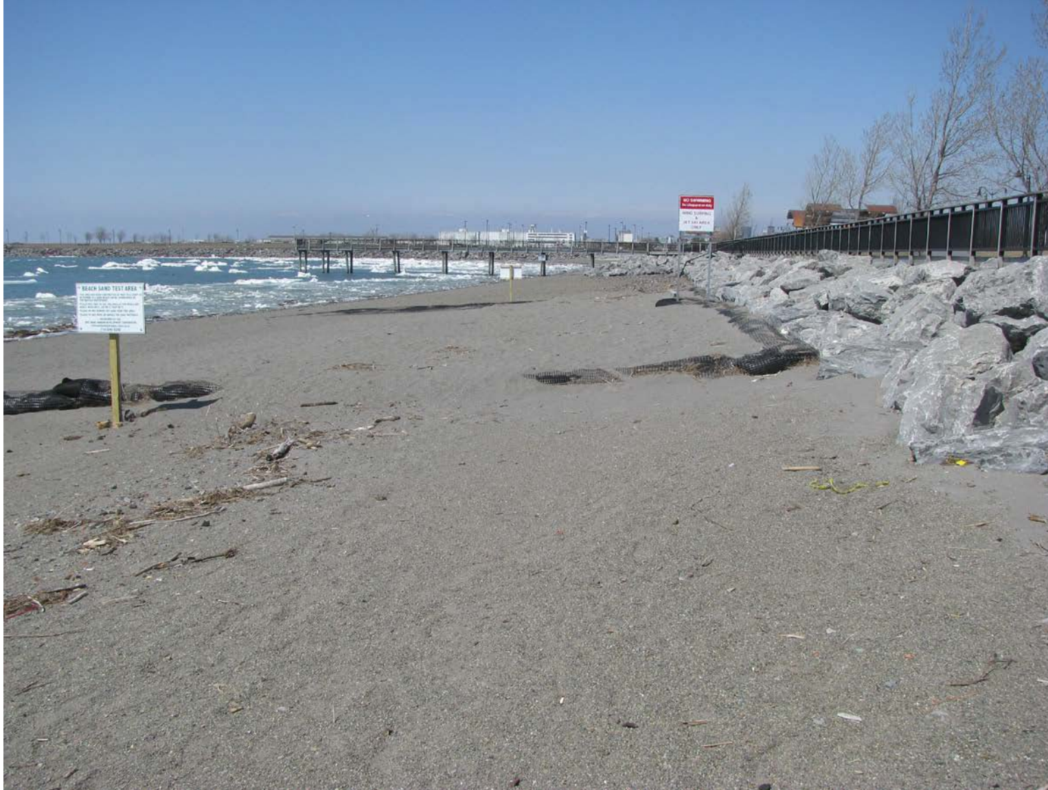
Gallagher Beach Photo 8: Looking north along drift line at the south edge of the test area. The burial of the edge restraint here appears to be man-made as it corresponds to the same condition on the north edge restraint.
