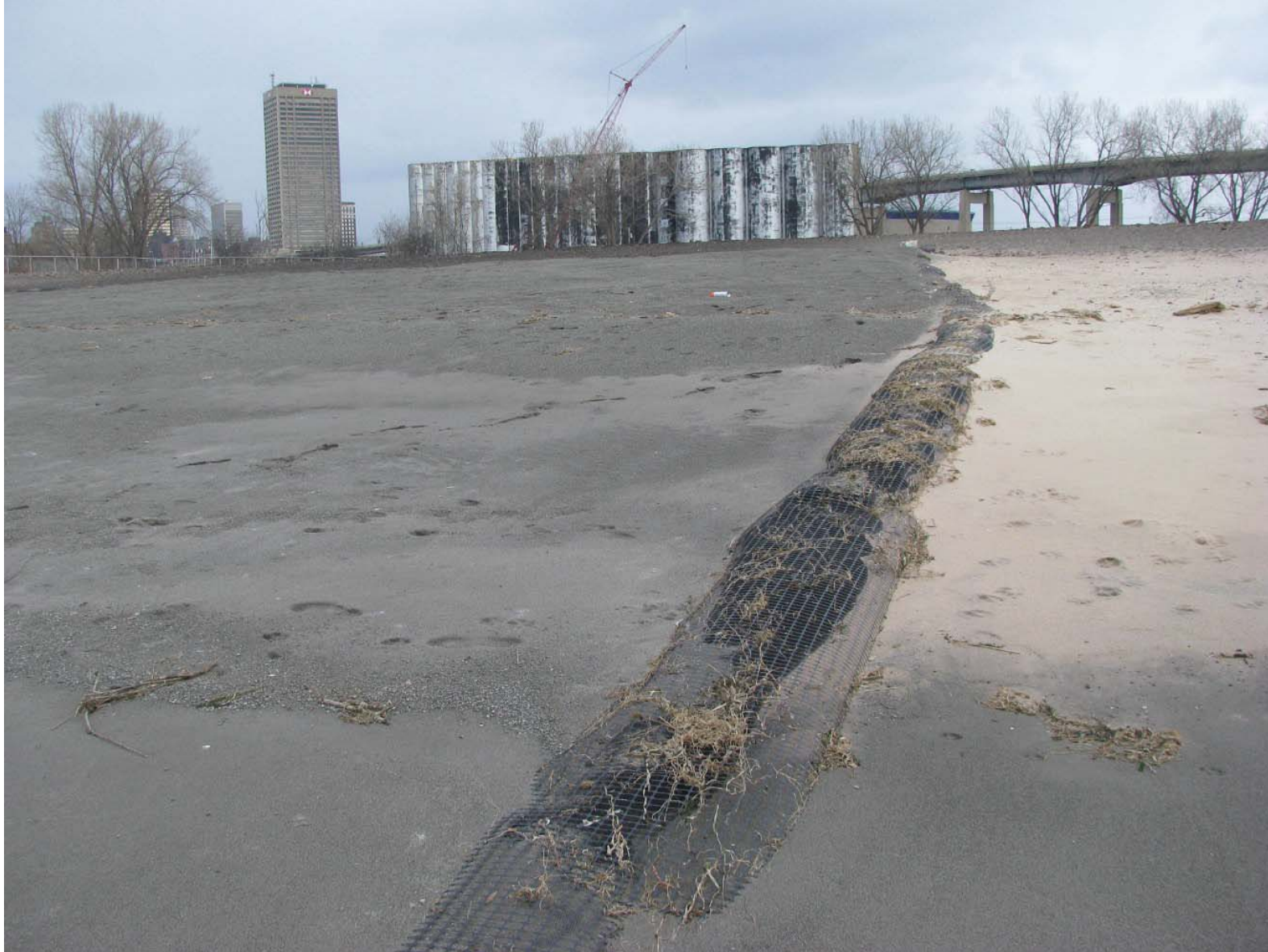
NYPA Parcel Photo 3: Looking eastward (inland) from near waterline. Note apparent burial of the edge restraint in the foreground.
