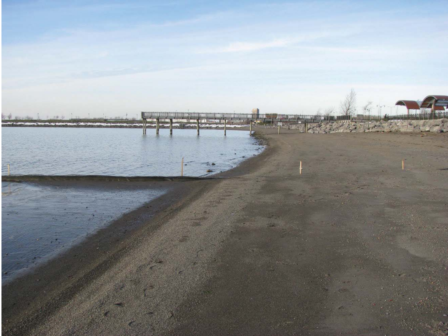
Gallagher Beach Photo 6: Look northward along the waterline. Note exposed top of edge restraint at the waterline and lower.
