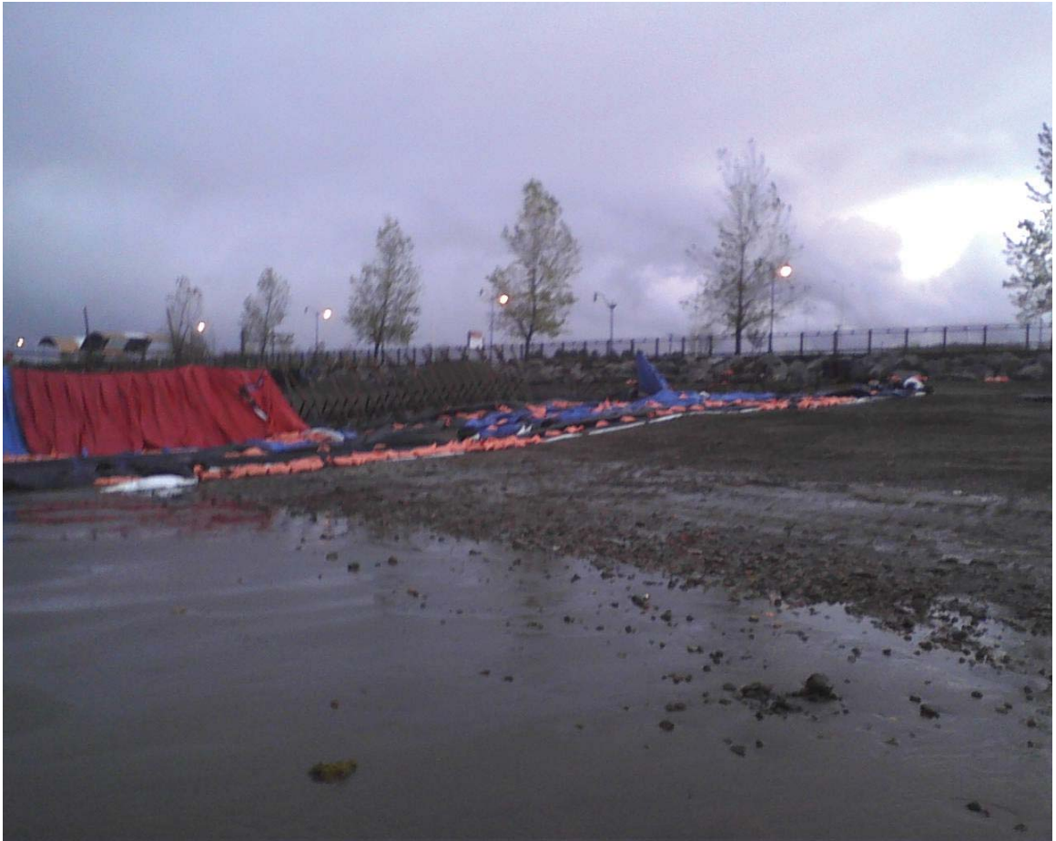
Looking northeast at the fabric from the coffer dam blown off of its frame, as well as the sandy bottom of the Gallagher Beach nearshore area exposed during negative seiche due to passage to the west of the remnants of Hurricane Sandy.
