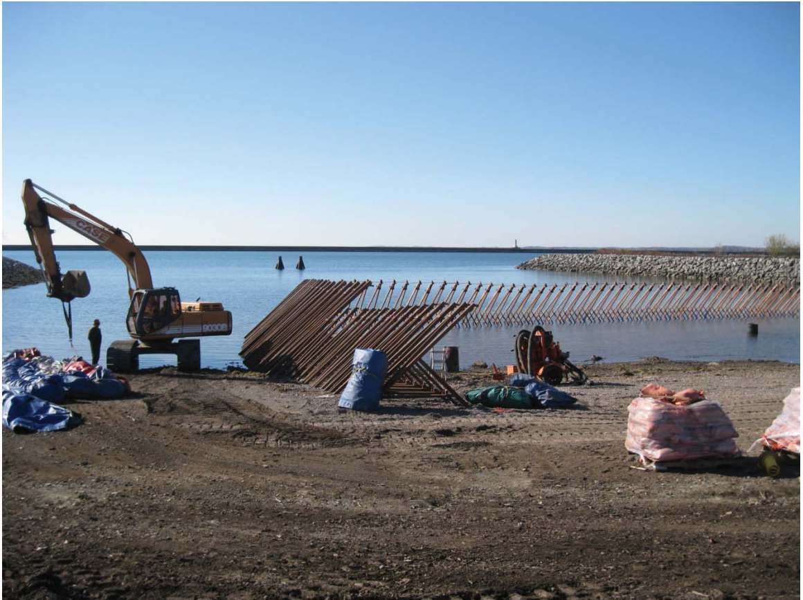
Set-up of Coffor Dam at NYPA Parcel.
