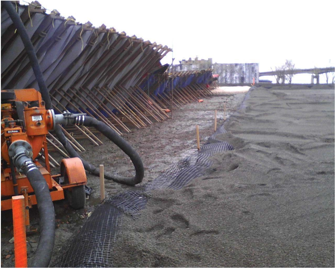
Looking upslope along the north side of the test area during installation at the NYPA Parcel.
