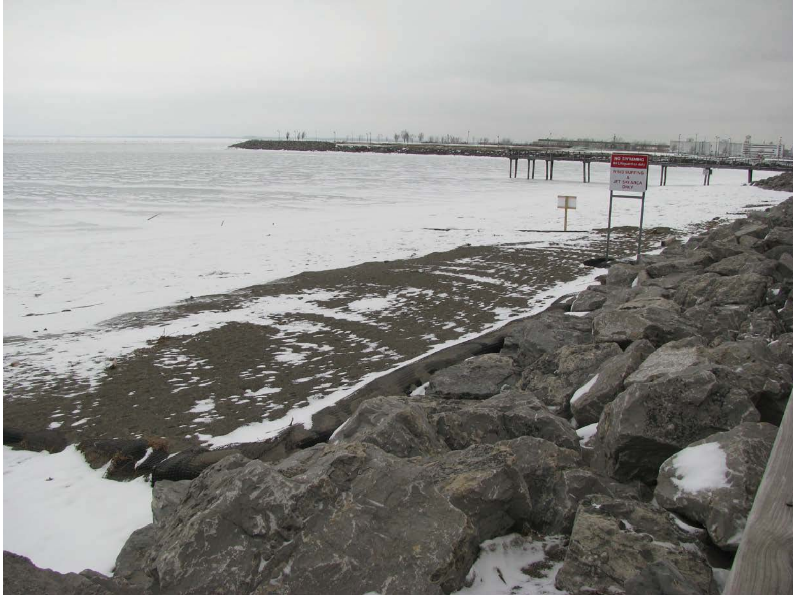
Gallagher Beach Photo 3: Looking northwest over the test area. Note the sand blown over the edge restraint.
