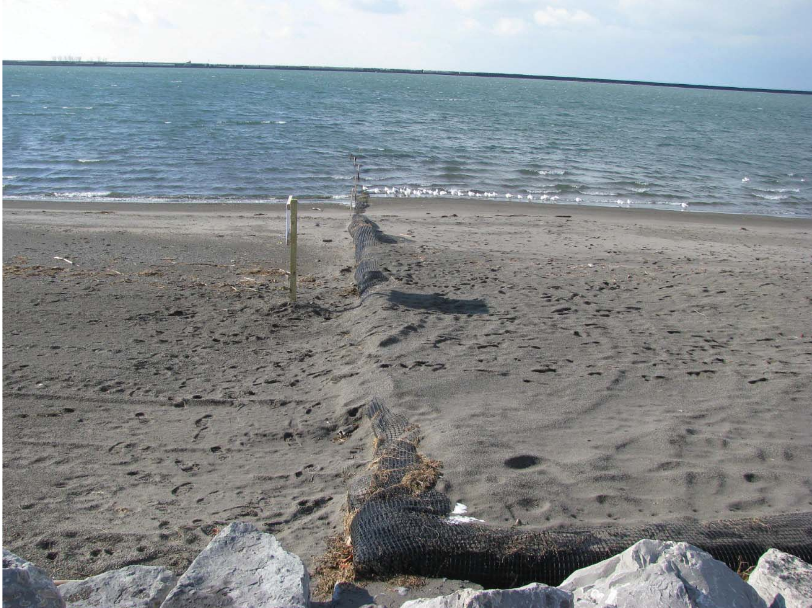
Gallagher Beach Photo 4: Look westward along southern edge restraint.
