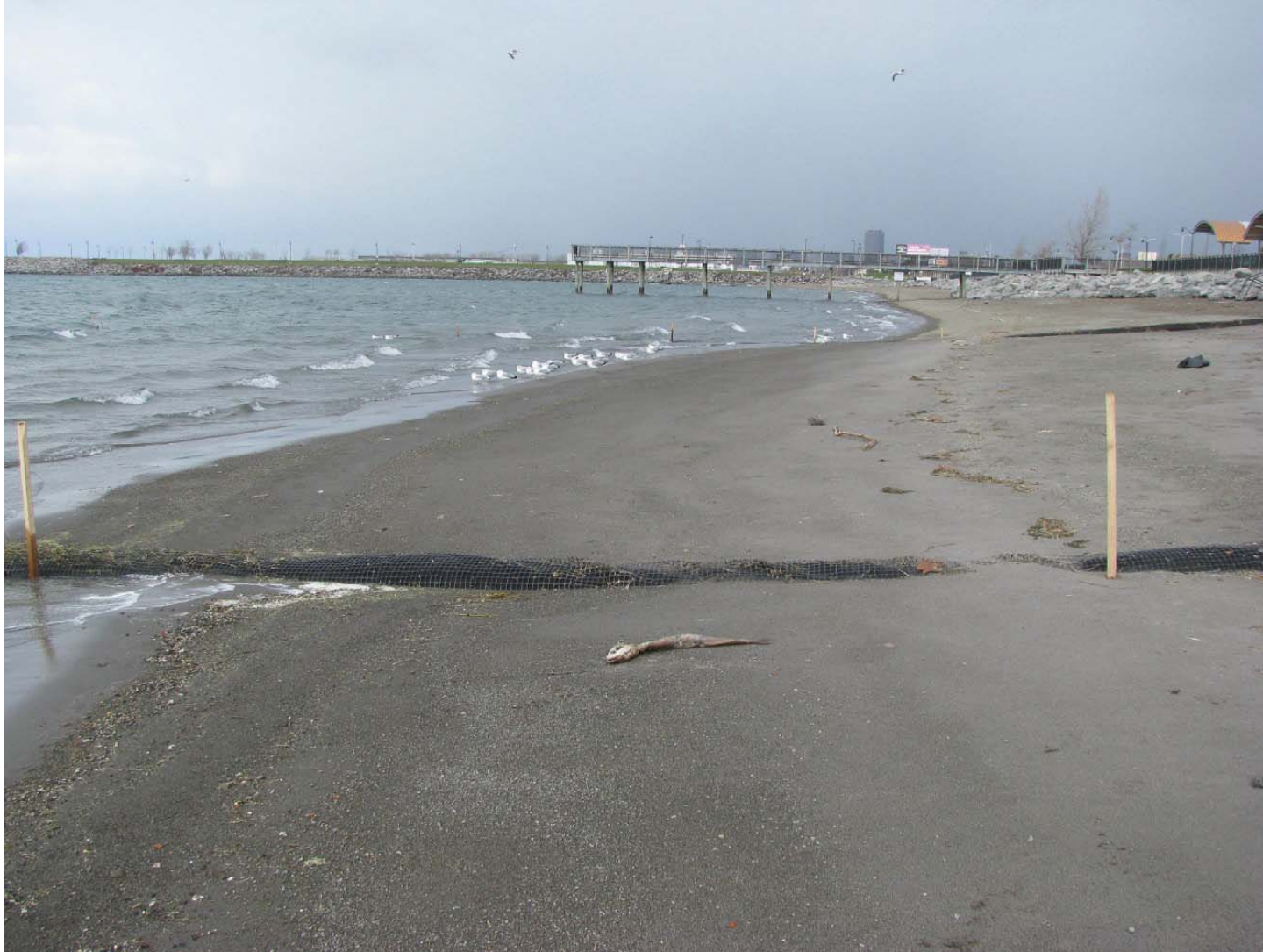
Gallagher Beach Photo 1: Looking North along the shoreline – note the downslope movement of sand within the test area, and the burial of the restraint both inside and outside of the restraint.
