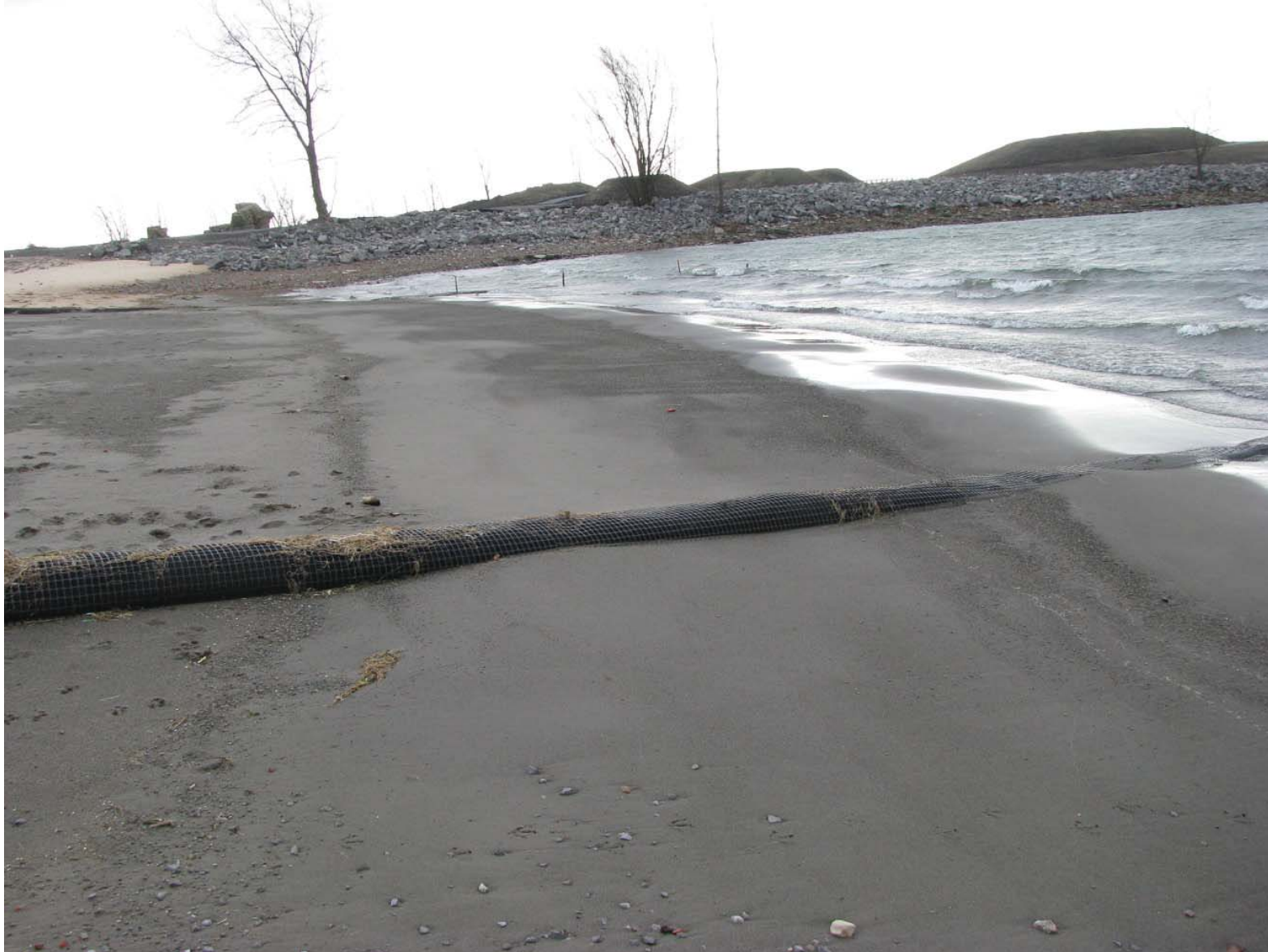
NYPA Parcel Photo 4: Looking southward at the test area – note the apparent burial of the edge restraint near the waterline.
