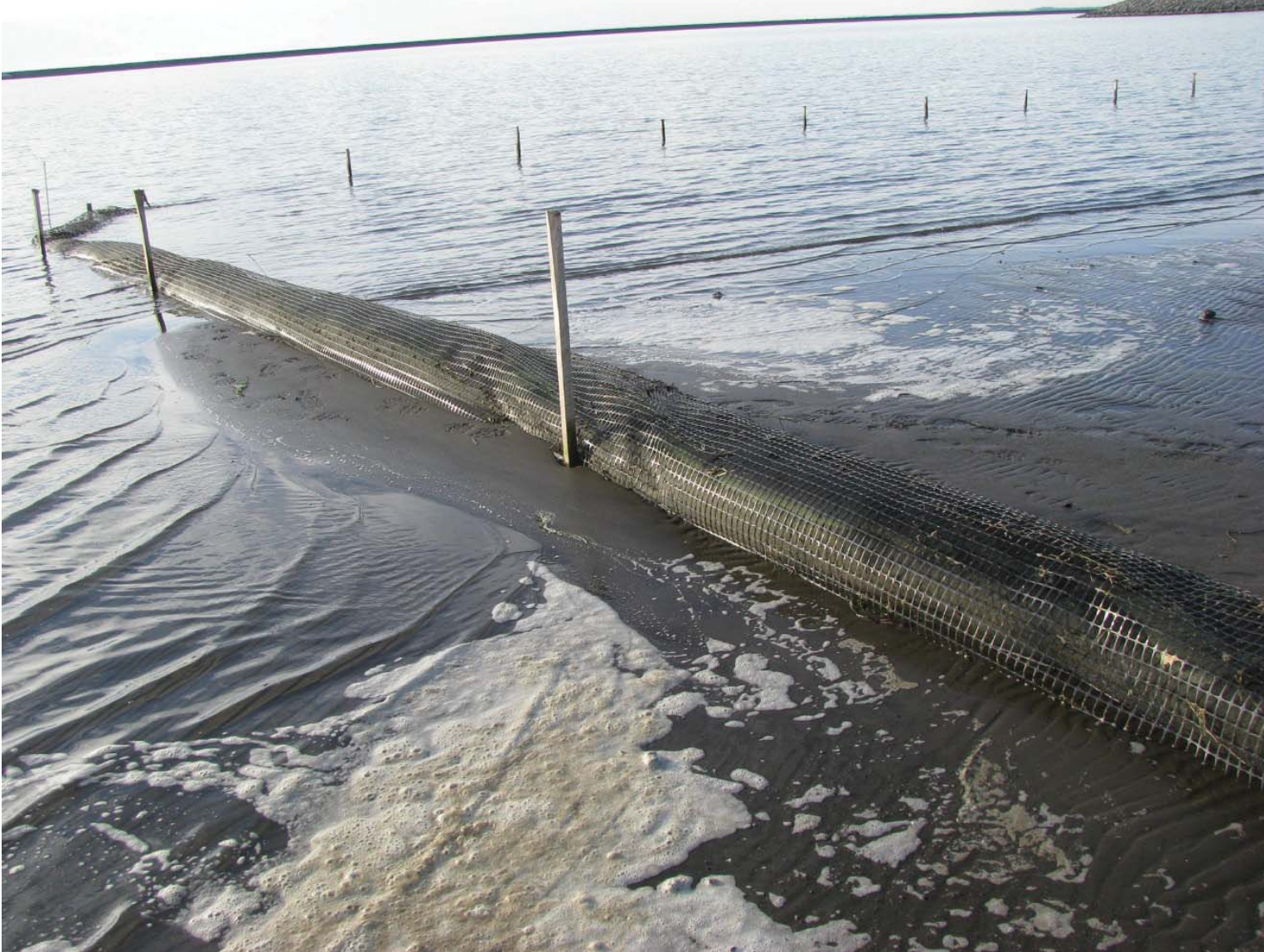
Gallagher Beach Photo 7: Look northwest from just south of the southern edge restraint. Note the loss of sand from within the test area.
