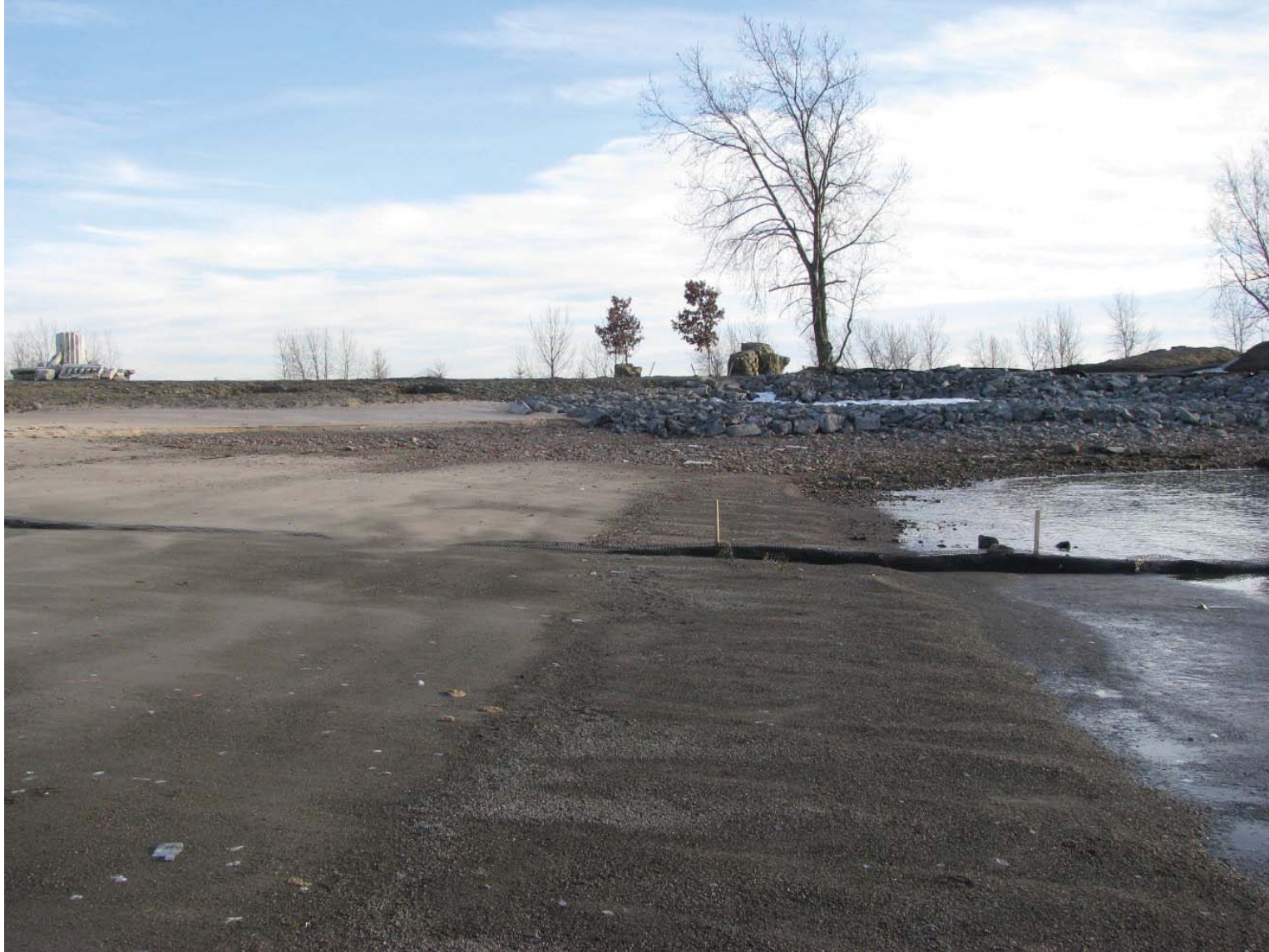
NYPA Parcel Photo 5: Look south along the waterline. Note again the process similar to Gallagher Beach: an accumulation of sand at the midsection, and loss of sand from the area at the waterline and below.
