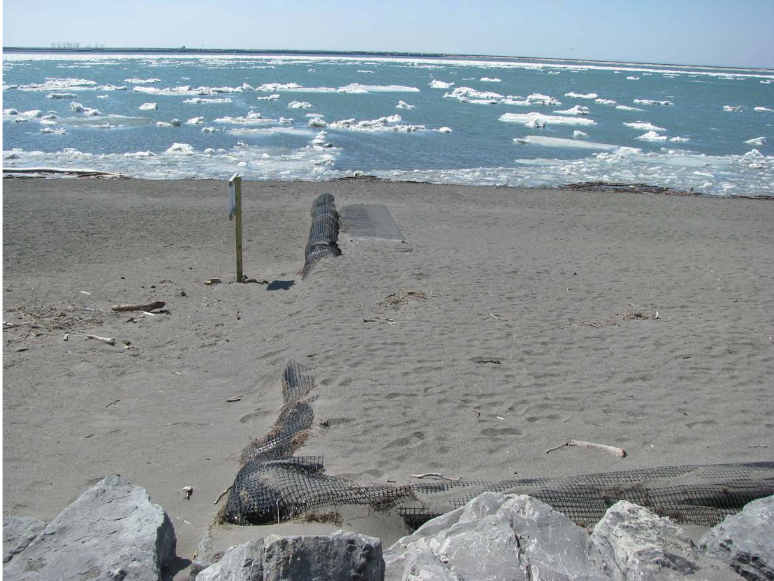
Gallagher Beach Photo 11: Looking westward along the southern edge restraint. This photo shows clearly the apparent
