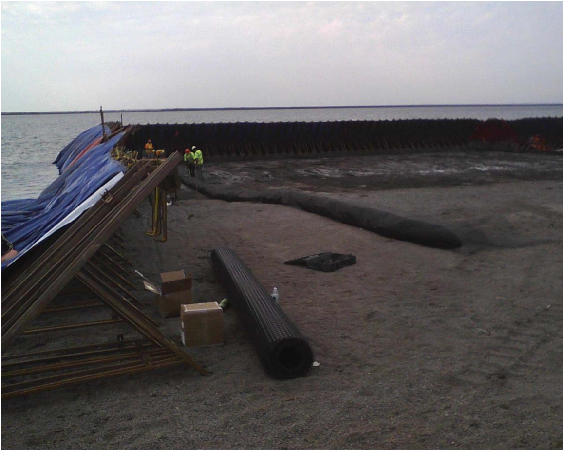
Installation of the southern edge restraint at Gallagher Beach.
