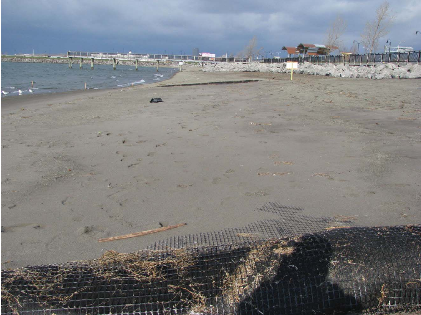
Gallagher Beach Photo 10: Same as photo 8, looking north. Note exposed lock-down netting.
