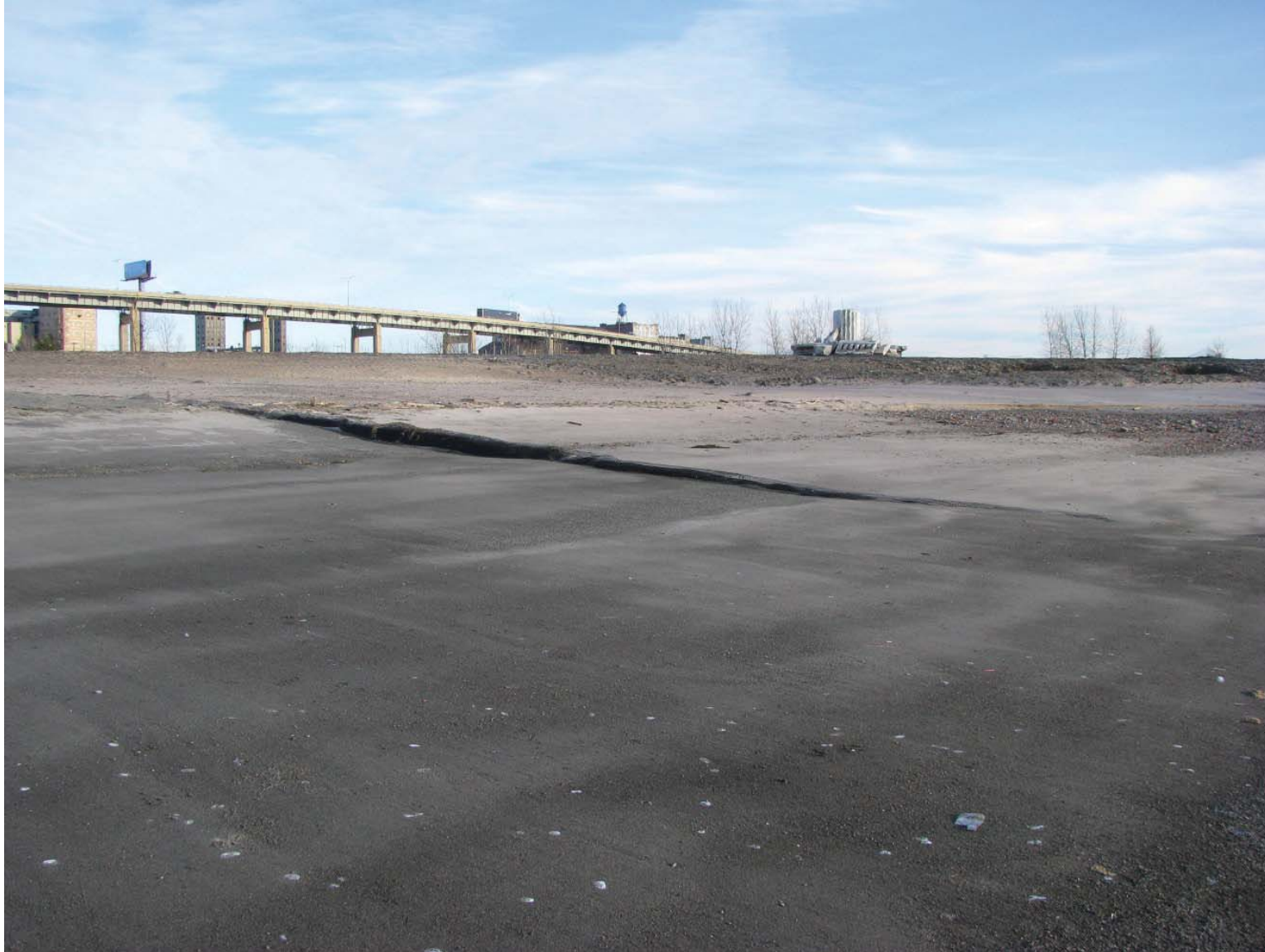
NYPA Parcel Photo 4: Look southeast from within the test area. Processes here are similar to Gallagher Beach – a laterally (north-south) symmetrical translocation of sand from the upper reach to the midsection of the test area.
