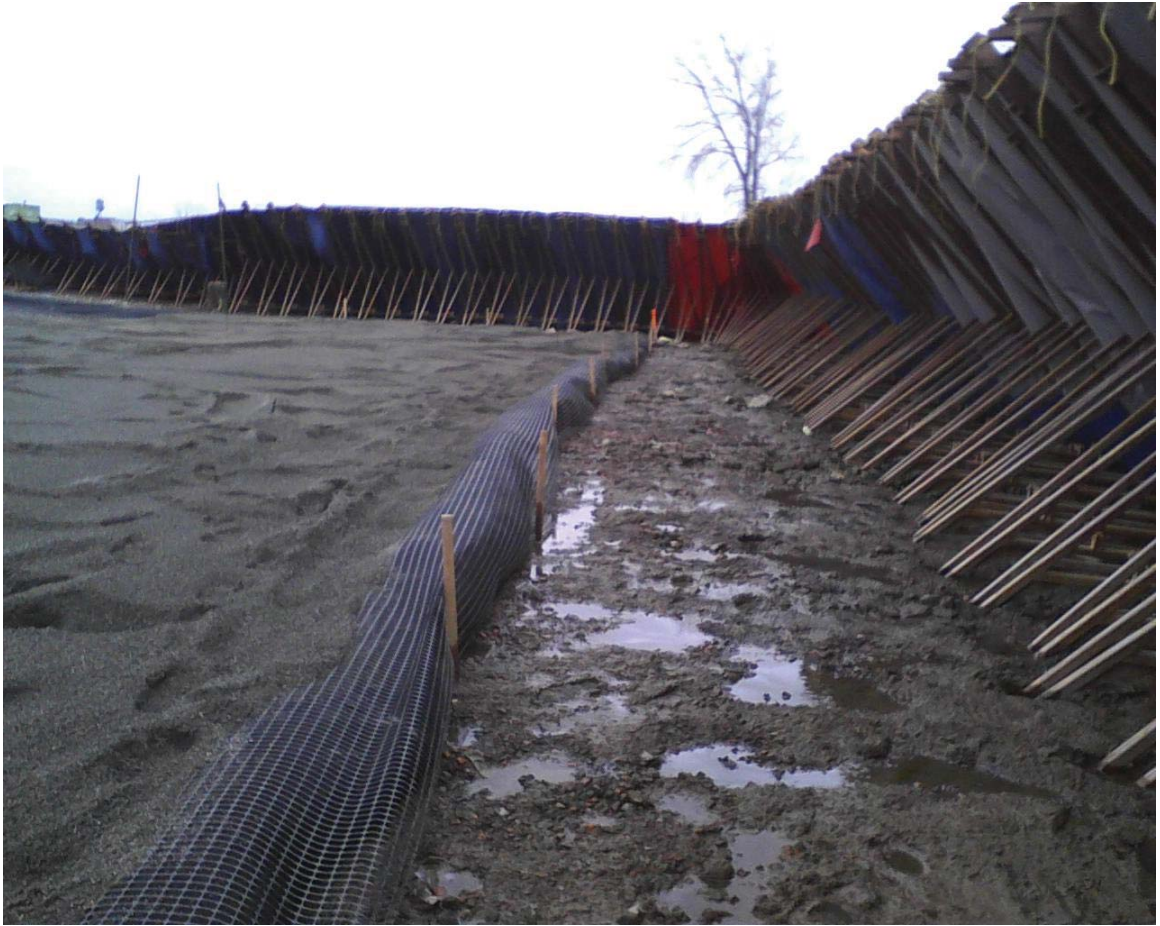
Looking along (south) the downslope toe of the test area behind the coffer dam at the NYPA parcel.
