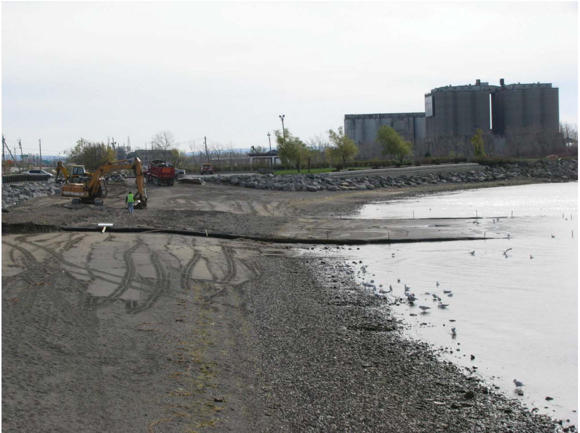
Final clean-up and demobilization of the Gallagher Beach test area
