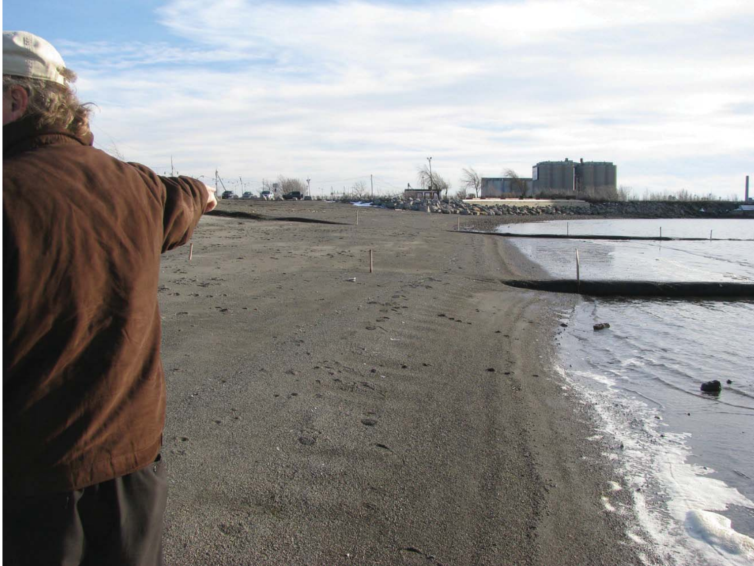
Gallagher Beach Photo 4: Look south along the waterline showing the sand accumulation in the middle section as well as the area of sand loss (note exposed top of edge restraint) at the waterline and lower.
