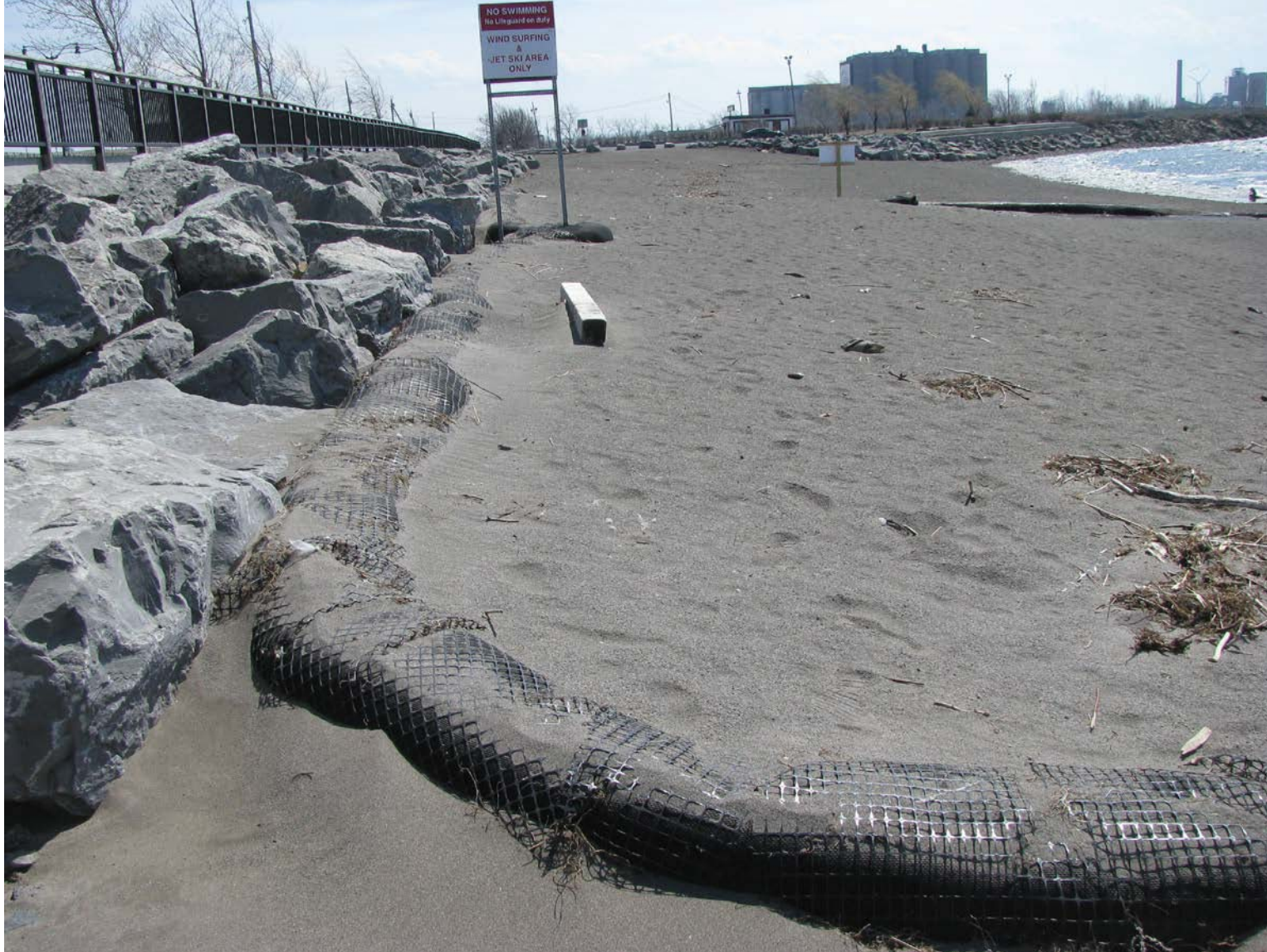
Gallagher Beach Photo 6: Looking south along the top of the test area. Note the uniform, fine wind-blown sand over the top of the edge restraint.
