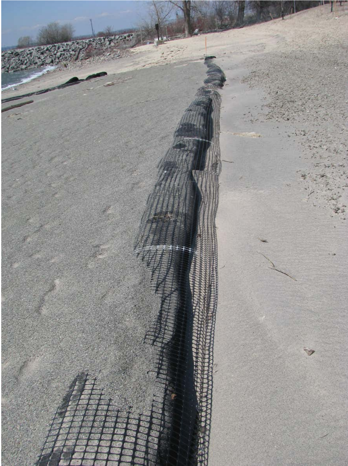
NYPA Parcel Photo 5: Looking north along upslope edge restraint. Note uniform, fine-grained wind-blown sand on upslope side.
