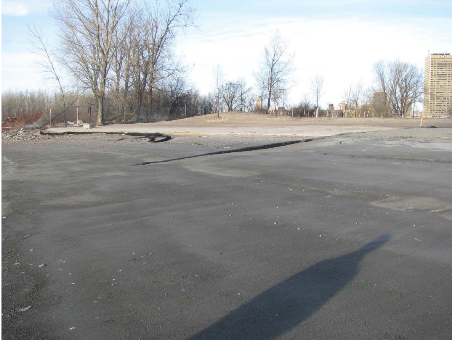
NYPA Parcel Photo 3: Look northeast from within the test area. Note the translocation of sand from the upper portions (where edge restraint is exposed) to the approximate mid section, similar to the process observed at Gallagher Beach.
