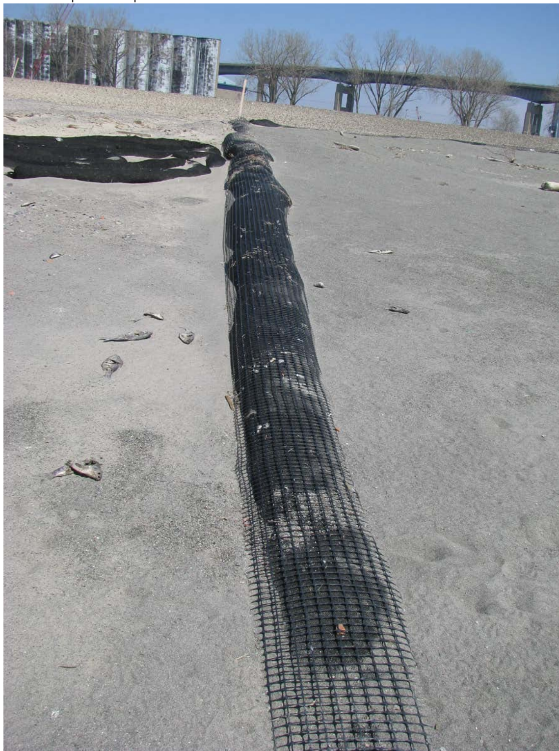
NYPA Parcel Photo 2: Looking upslope (eastward) along northern edge restraint.
