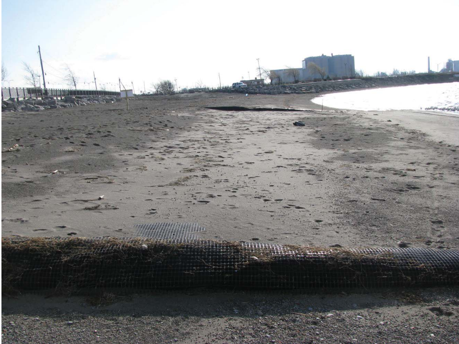
Gallagher Beach Photo 8: Look south at the area from which sand has been removed, upslope of the area in the previous photo. Note the slight scarp at the upslope edge of the area of removal.
