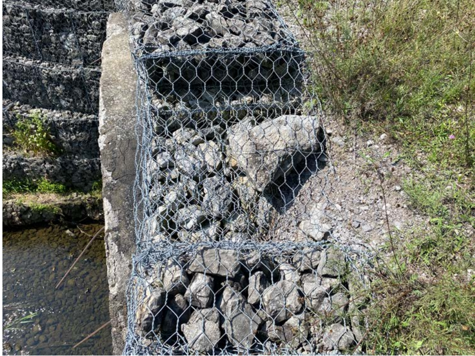
Photo 1: (8/22/2024) The gabion basket on-site that needs to be repaired.
