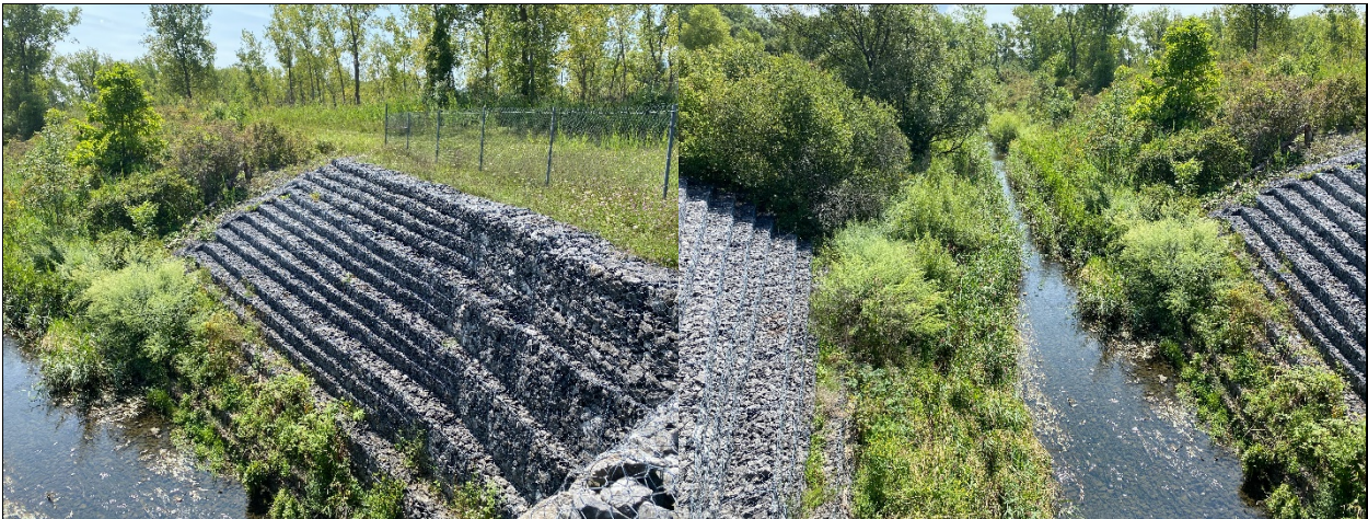
Photo 23-24: Gabion basket wing walls adjacent to the culvert.
