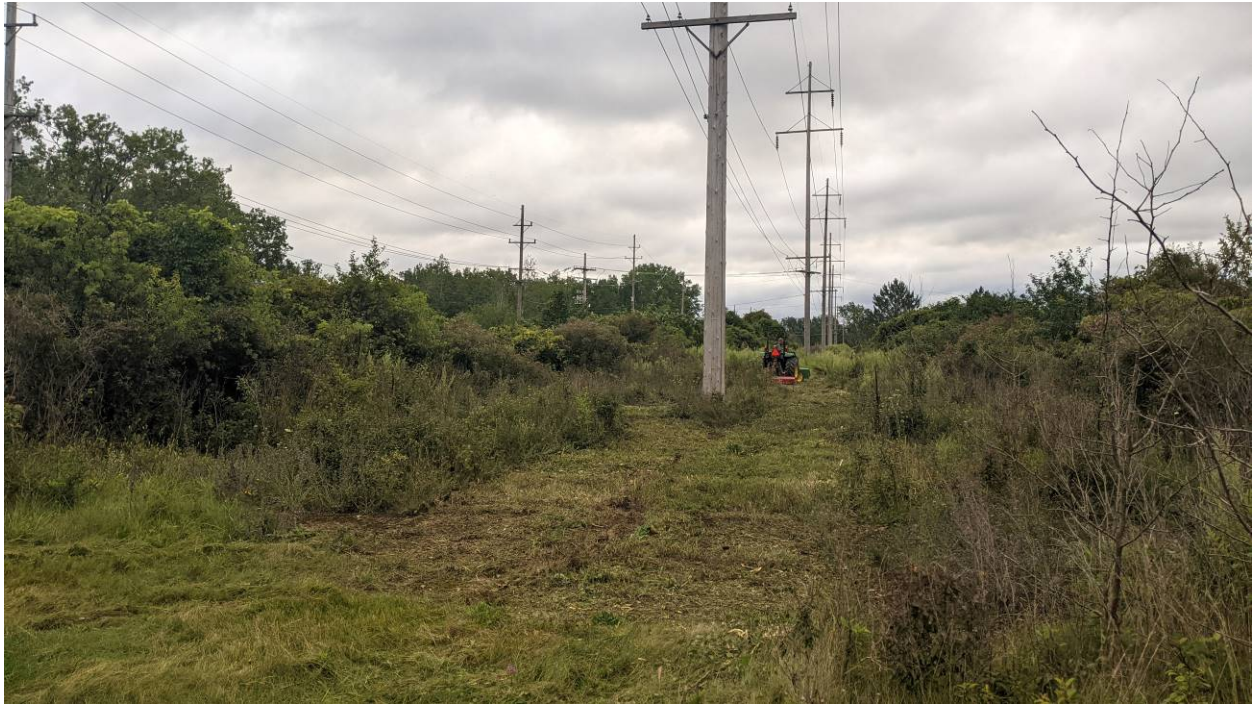
Clearing vegetation along the eastern side of the Former Roundhouse
