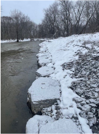
Photo 5: Area 1 Embankment Restoration
