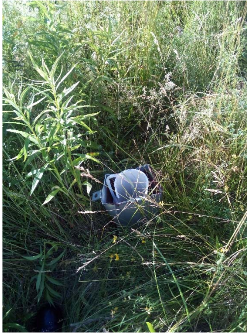
Photo No. 1 – Monitoring well RD-3/RD-3R with damaged protective casing and damaged PVC riser.
