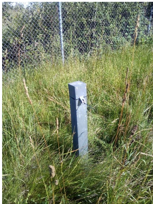
Photo No. 18 – Monitoring well RD-1.
