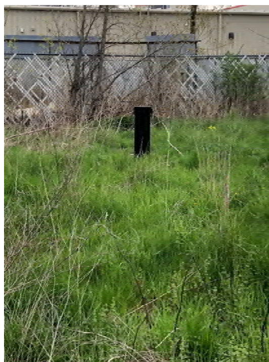
Photo No. 2 – Monitoring well RD-3/RD-3R with new protective casing and repaired PVC riser.
